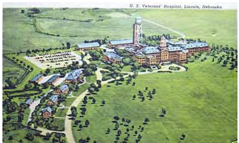
Postcard aerial view of Lincoln VA Hospital from northwest, ca. 1932 Extant in 2015 (Lincoln/Lancaster County Planning Dept.)
