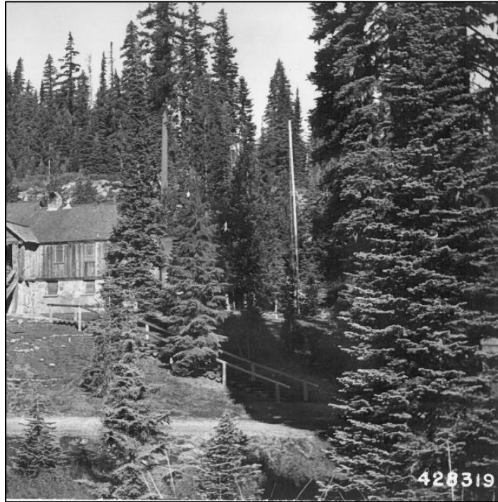
Figure 12: View North with access road in foreground, half round log stairs and east side of front elevation.
