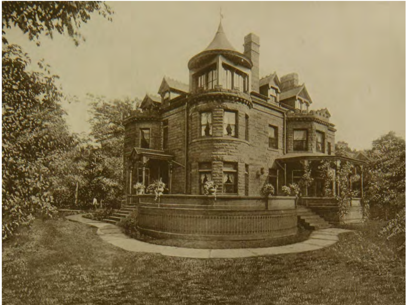
Figure 9. North-facing corner of the Scofield Mansion with original porch, main entry, and dormer ornamentation. From Beautiful Homes of Cleveland, 1917 via Cleveland Public Library Digital Photograph Collection.
