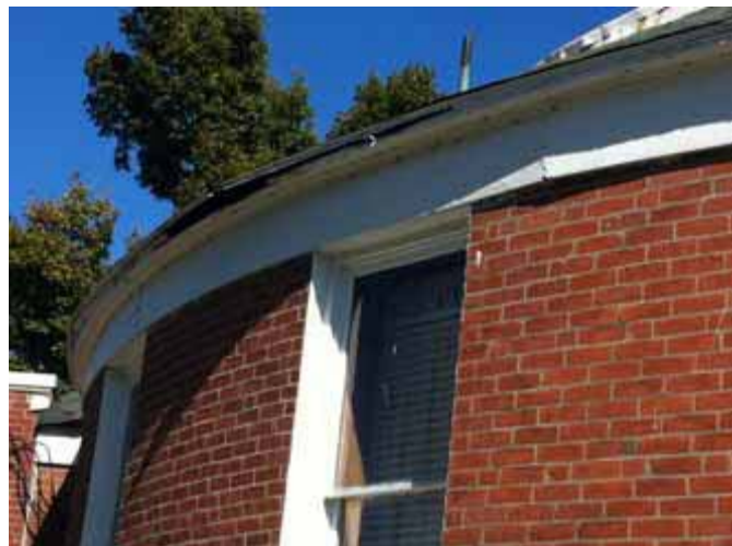
West façade, partial
