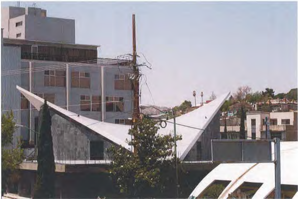
Fig. 17. Nogales Border redevelopment 1962, Architect Mario Pani. Photo by THPF.
