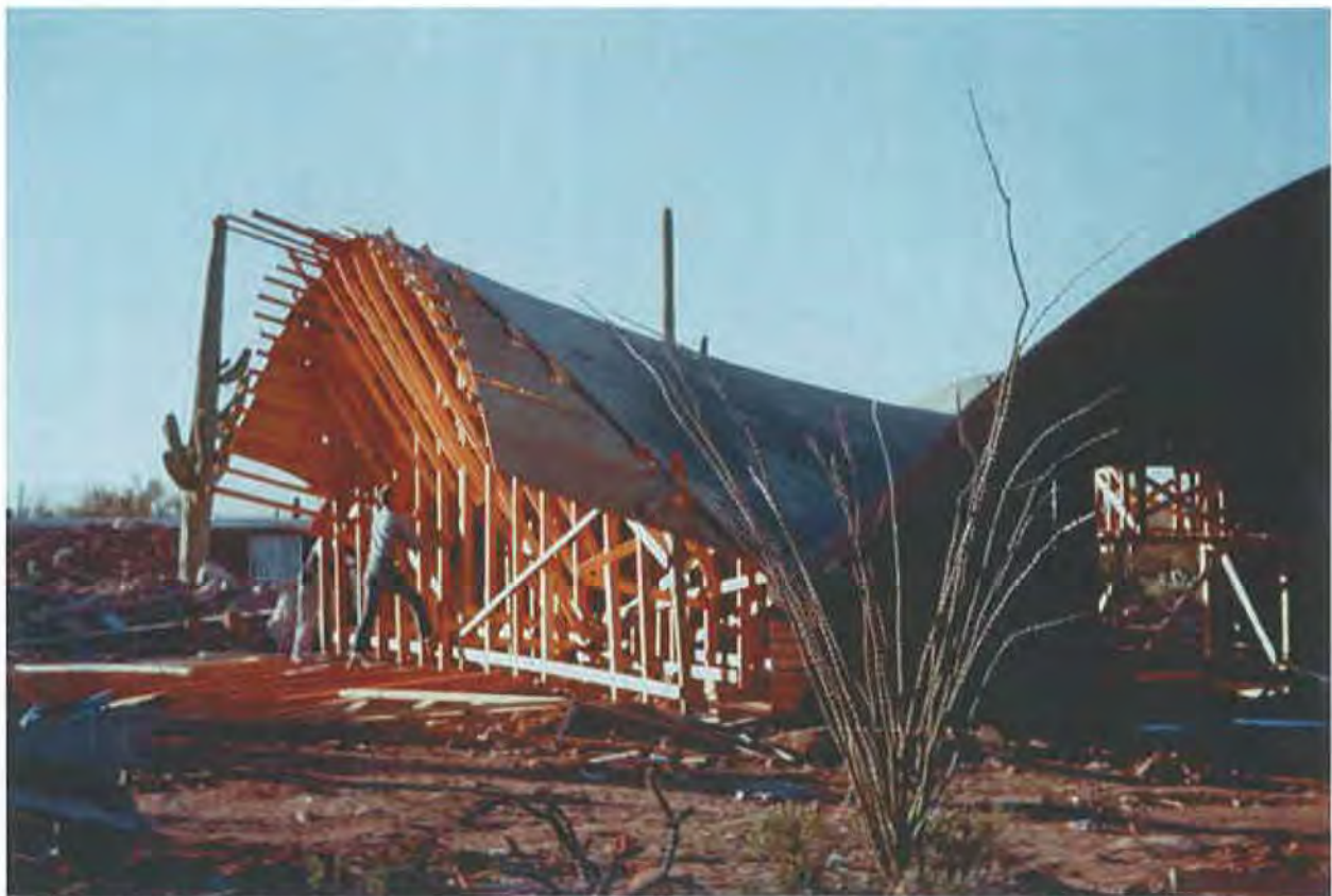
Fig. 11. Harrenstien House under construction, photo by Howard Harrenstien 1962-63. THPF digital collection.
