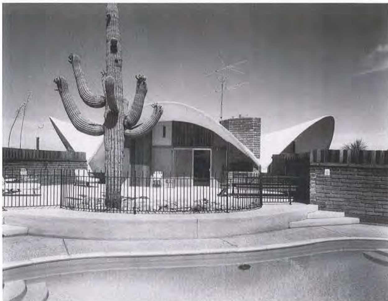
Fig. 3. Harrenstein House, southeast elevation, "backyard" with pool in foreground. Photo by Bill Sears, 1966.
