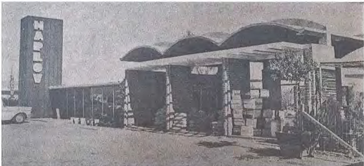
Fig. 13. Harlow Nurusy, Thin Shell concrete barrel roof design, Architect William Wilde, 1958. Photo Tucson Daily Citizen , 1958.
