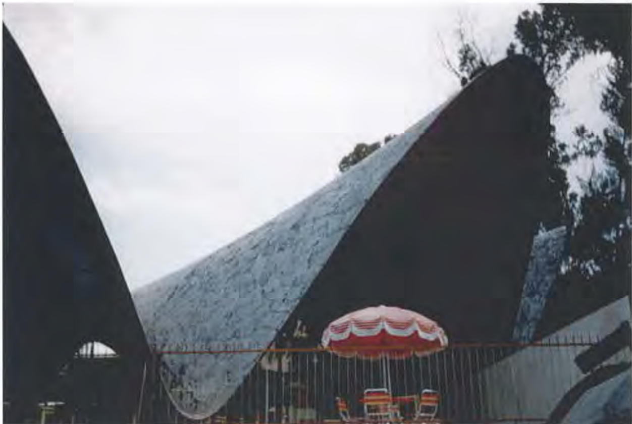
Fig. 8. “Los Manantiales” (1958) designed by architect Felix Candela, Mexico City, photo by Howard Harrenstien. THPF digital collection.
