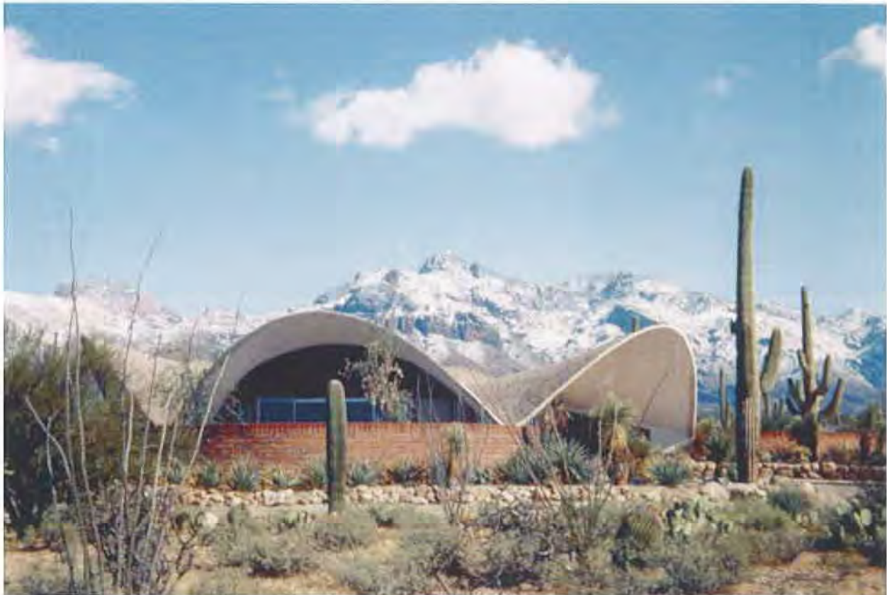
Fig. 7. Harrenstien House west elevation, photo by Howard Harrenstien 1963. THPF digital collection.
