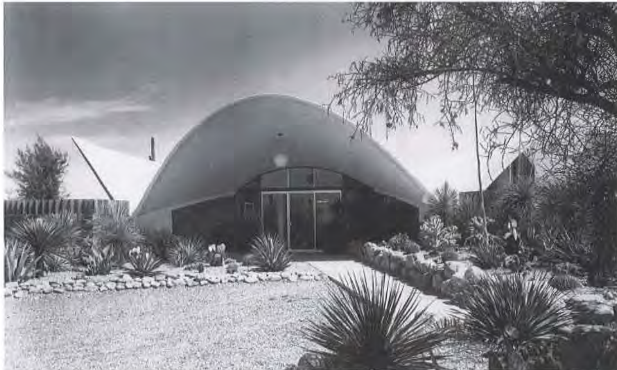
Fig. 6. Harrenstein House, South Elevation Entrance, photo by Bill Sears 1966.
