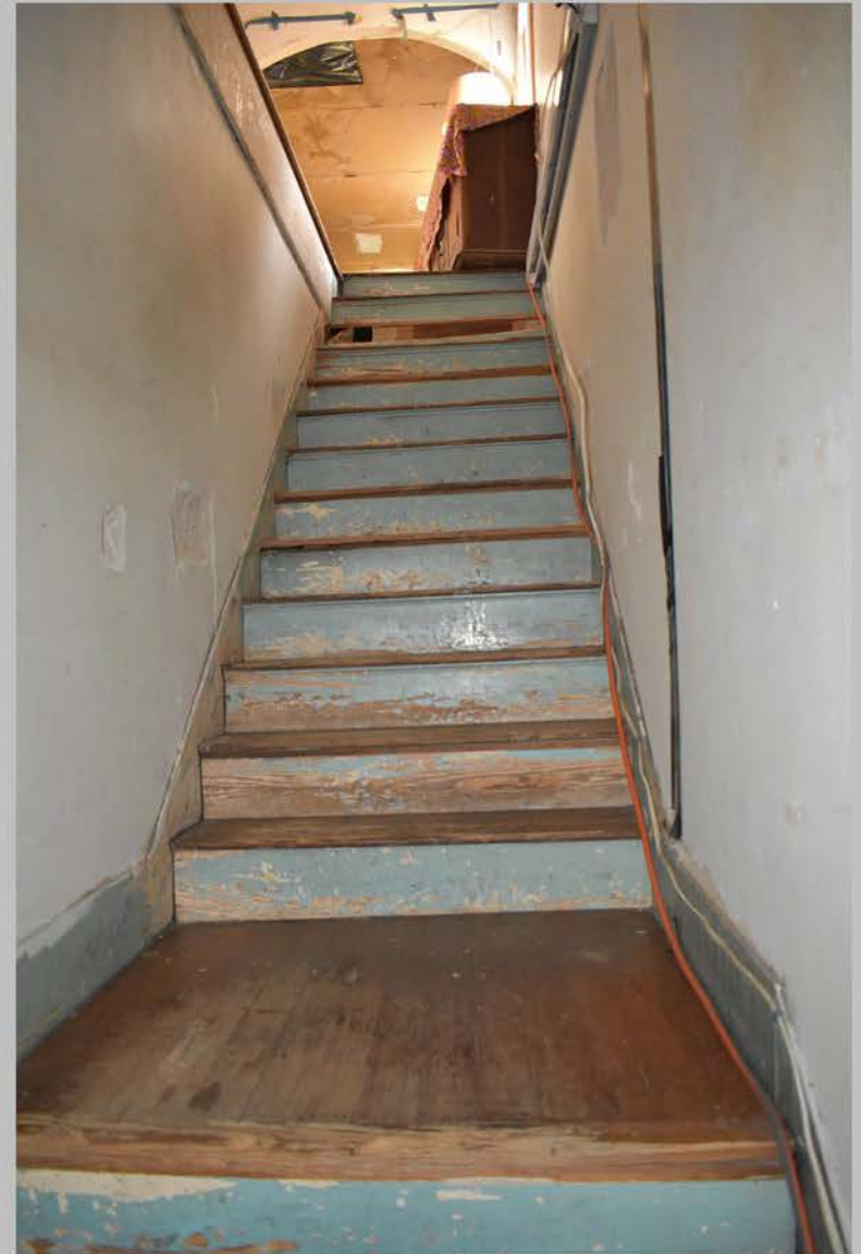
4. Stairs from first story entry to second story living space, looking southwest.
