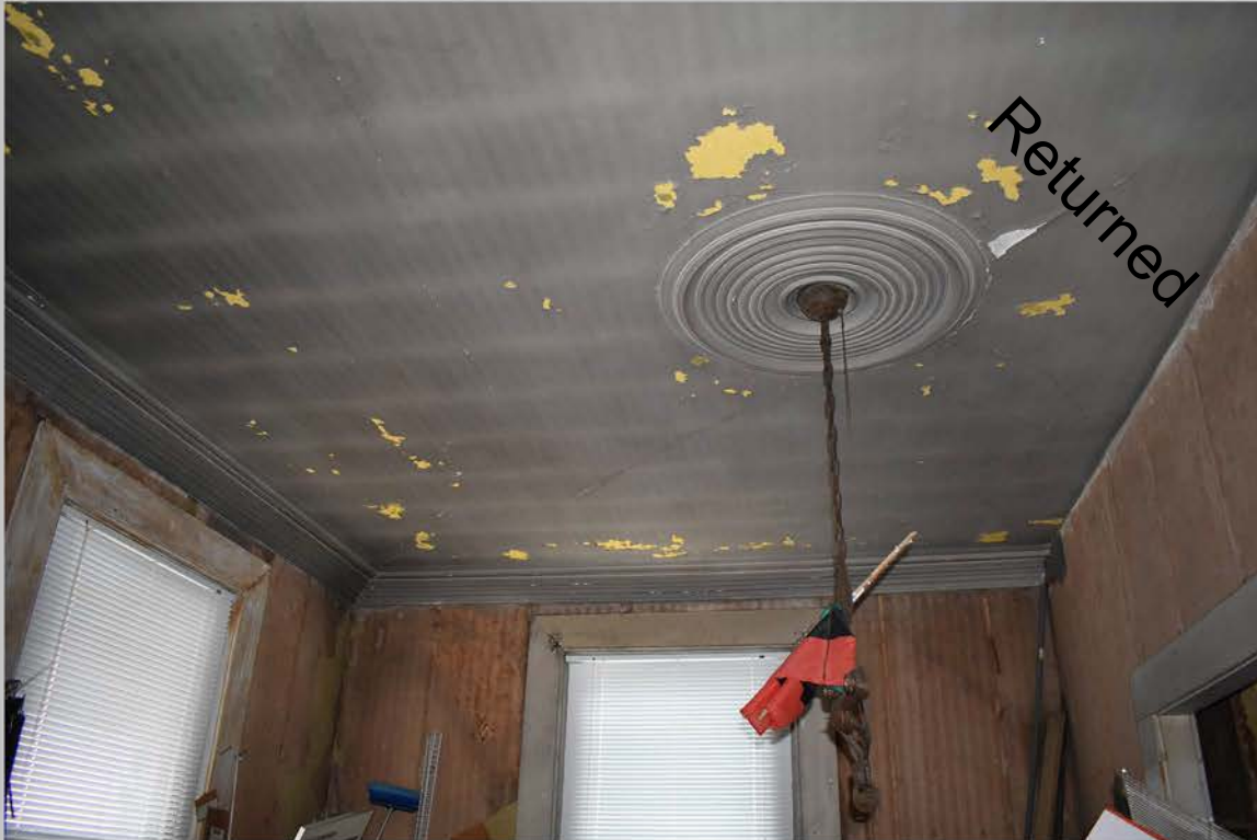
3. Plaster medallion and crown molding in first floor parlor, looking east.
