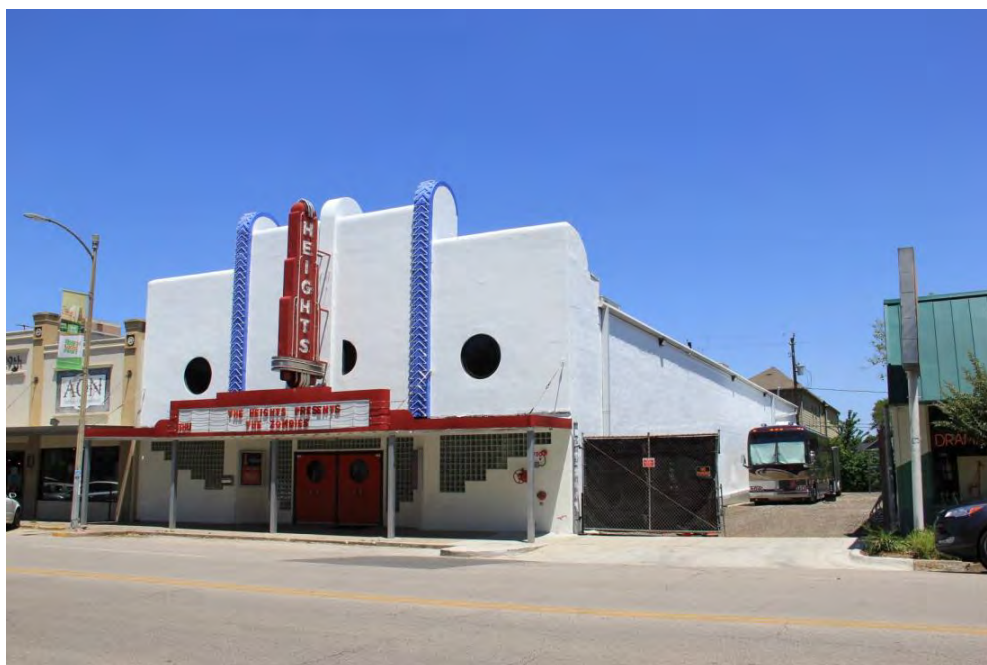
Photo 2: South facade, looking northwest, May 5, 2017
