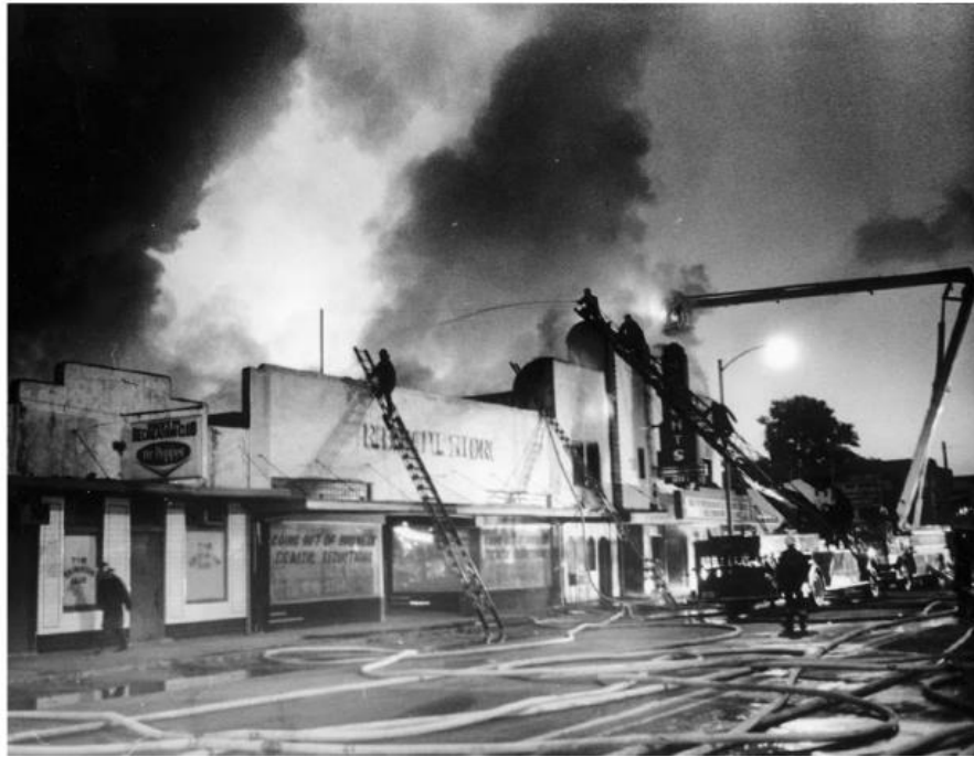
Figure 3: Photograph showing Heights Theater on fire, June 6, 1969. There is no known image in existence of the theater between 1935 and this time. Courtesy of the Houston Post.
