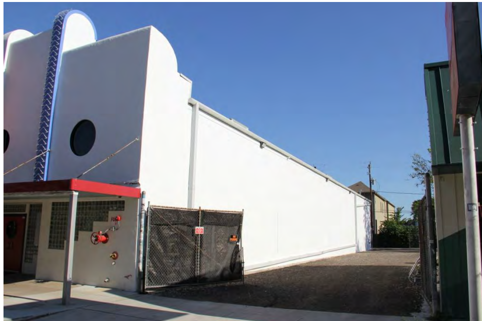
Photo 4: East Facade, looking northwest, May 5, 2017
