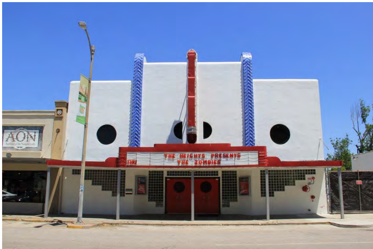
Photo 3: South Facade, looking north, May 5, 2017
