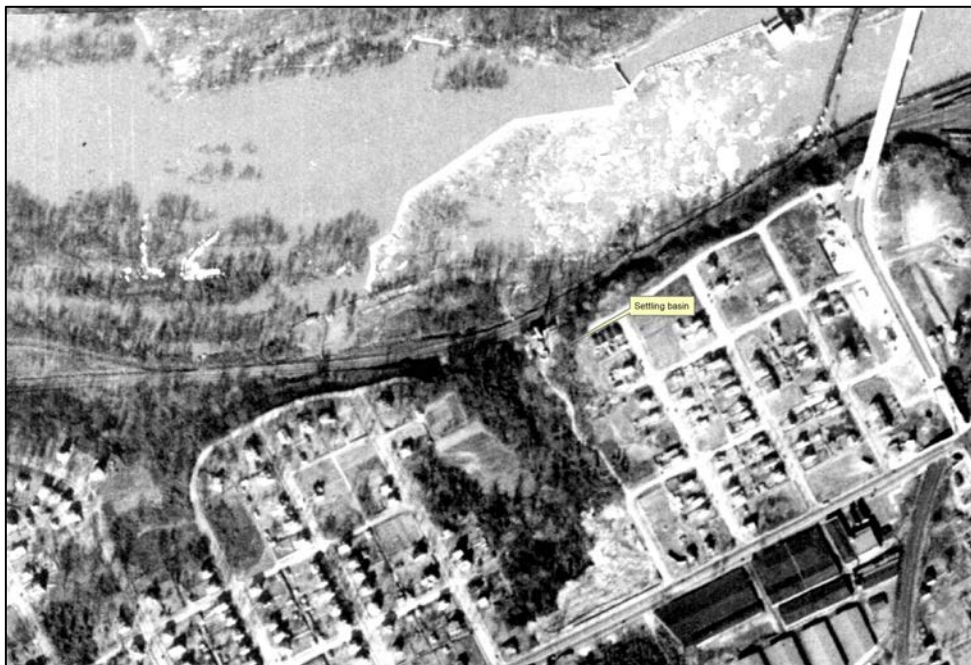
Figure 4. 1937 Aerial Photograph Showing the Location of the Abandoned Manchester Waterworks (the settling basins are circled in red). Image and annotation provided by Scott Williams.
