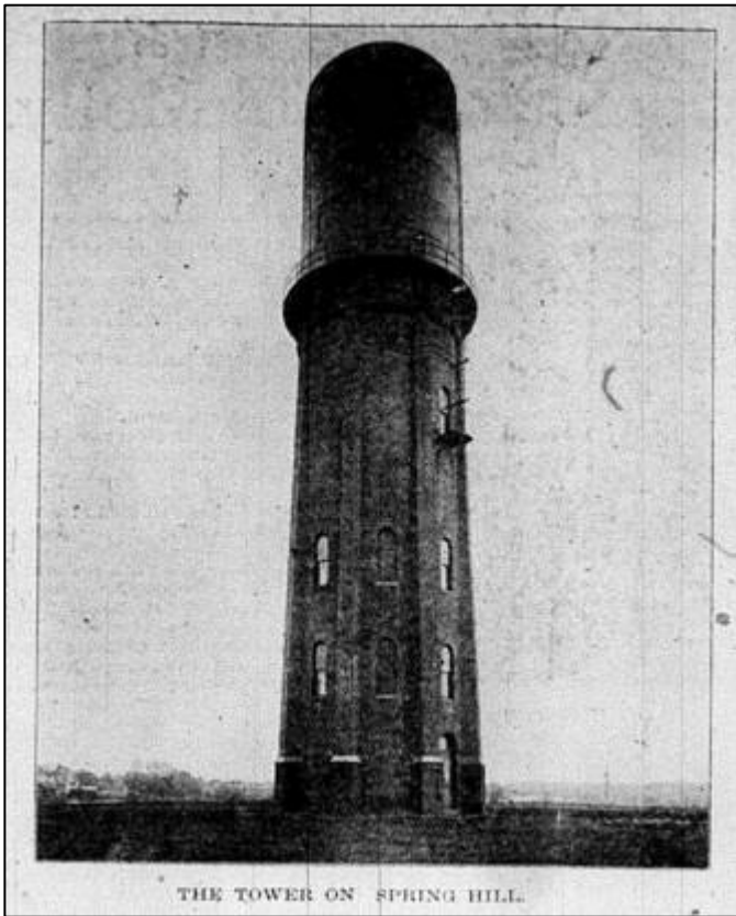
Figure 5. 1888 Photograph of the Manchester Waterworks' Water Tower. Image provided by Richard Helm.
