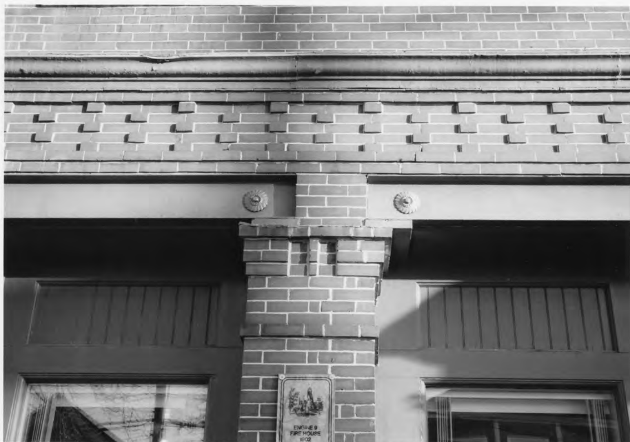
(FORMER) ENGINE CO.#9 FIREHOUSE; CUMBERLAND CO., ME
