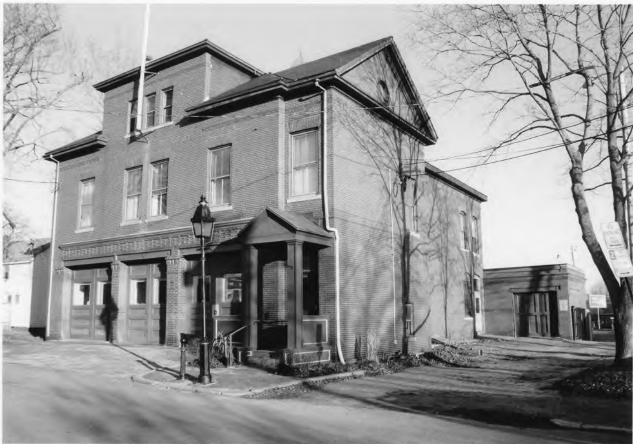
(FORMER) ENGINE CO. #9 FIREHOUSE; CUMBERLAND CO., ME
