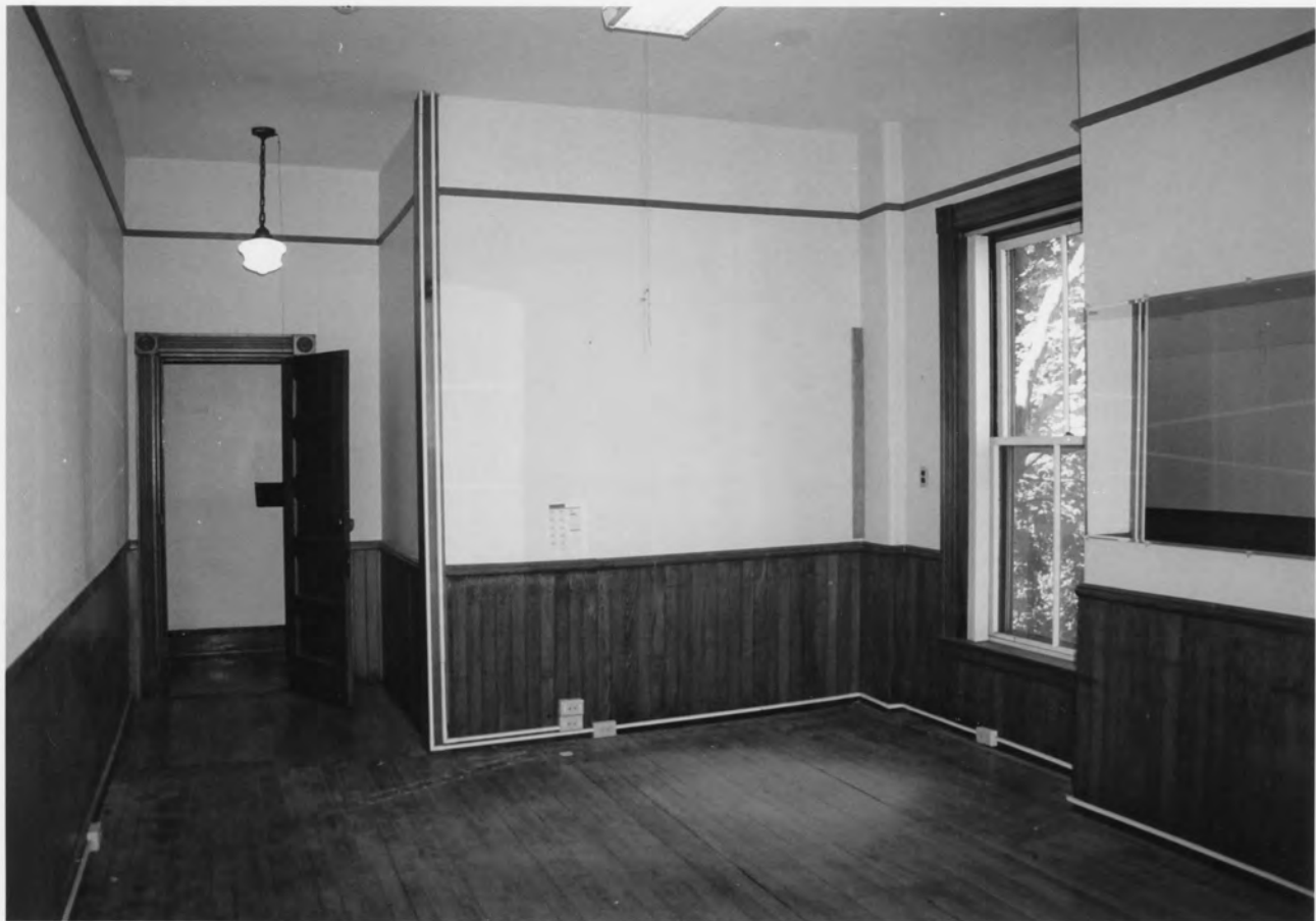
(FORMER) ENGINE CO. #9 FIREHOUSE; CUMBERLAND CO., ME.
