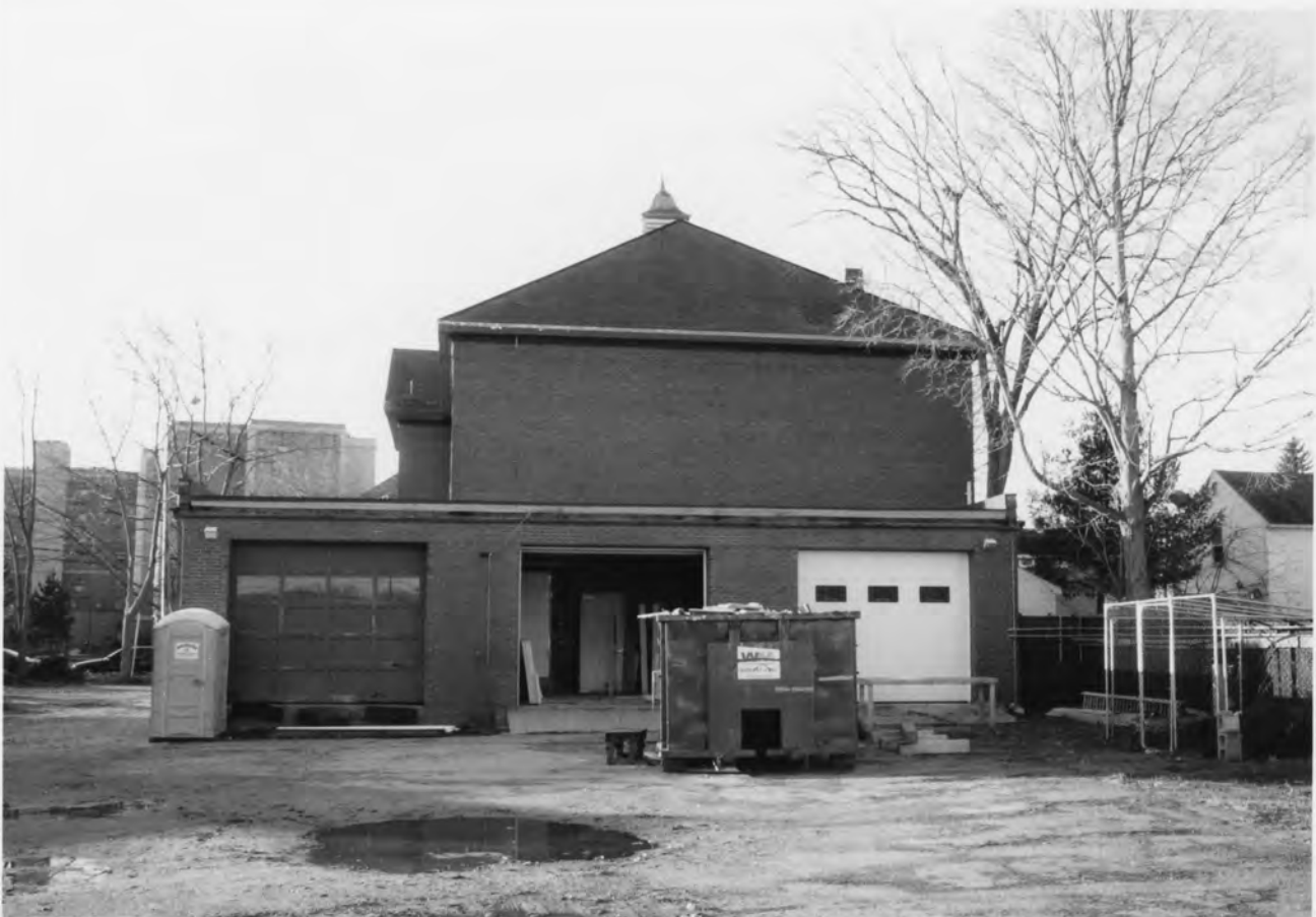
(FORMER) ENGINE CO. #9 FIREHOUSE; CUMBERLAND CO., ME
