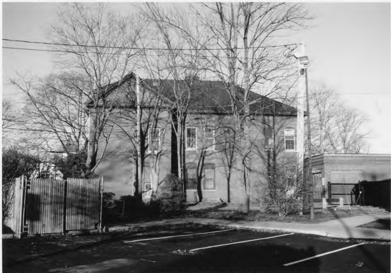
(FORMER) ENGINE CO. # 9 FIREHOUSE; CUMBERLAND CO., ME
