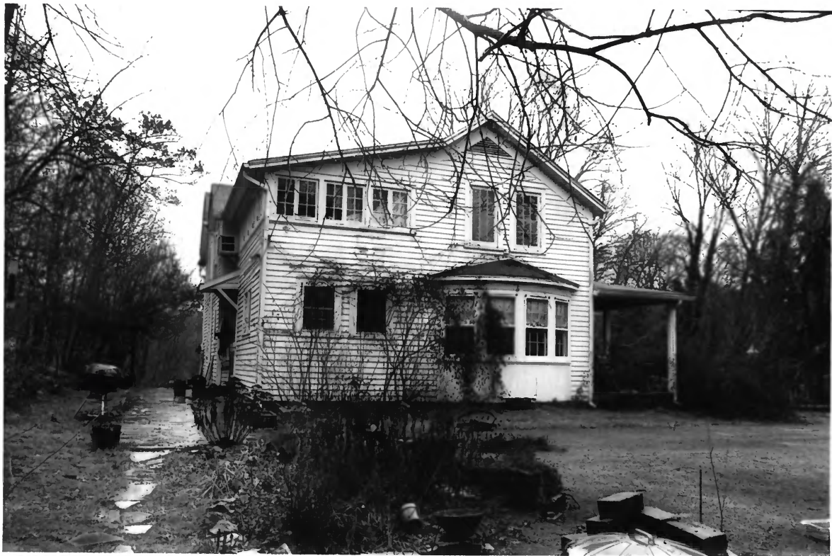
MAXWELL-KIRBY HOUSE KNOX COUNTY TN
