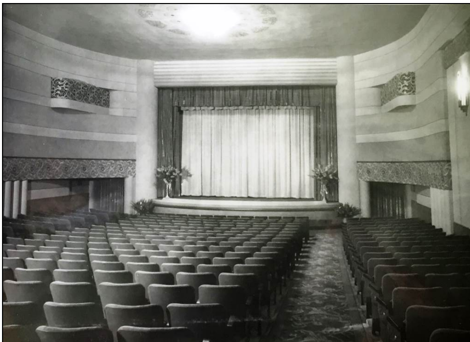
Figure 24: Cameo Theatre auditorium, 1937 (Brian Francis collection)
