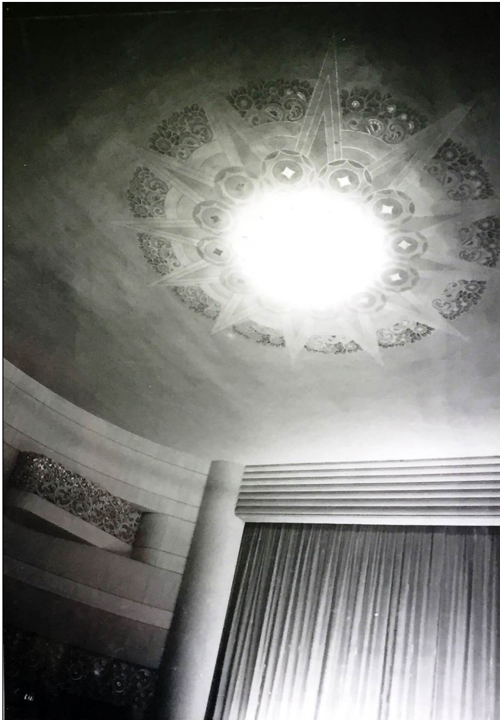
Figure 25: Cameo Theatre auditorium, 1937 (Brian Francis collection)
