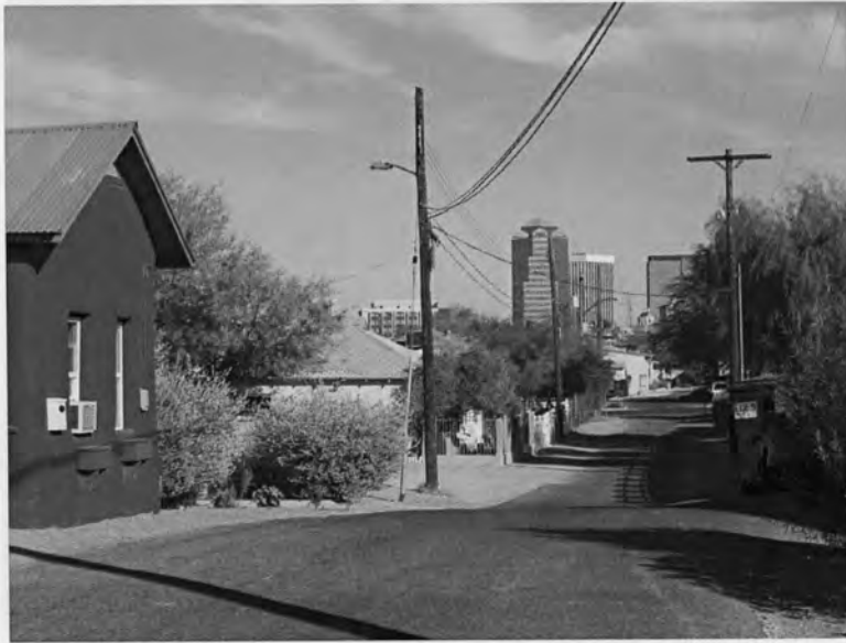
Photograph 17. S. Rubio Ave., at W. 19th St.; view north-northwest.
