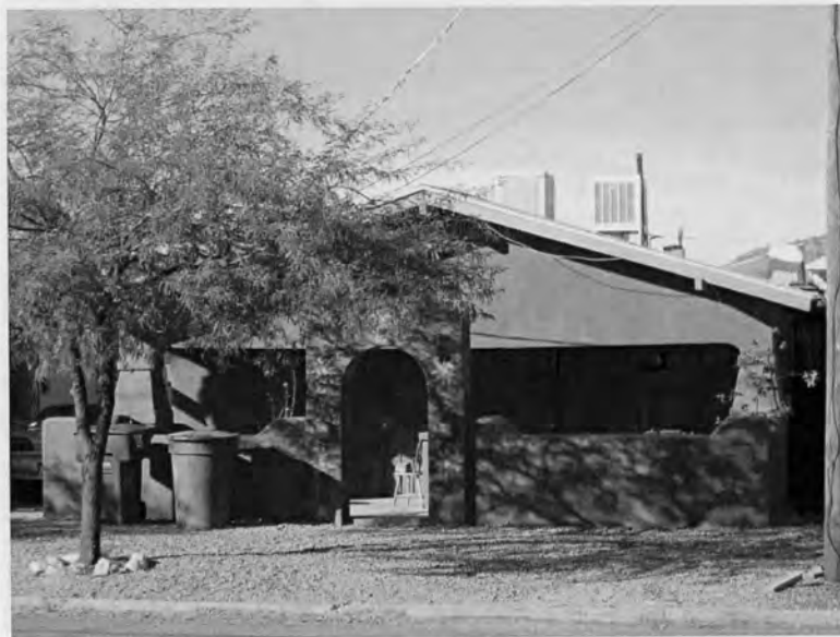
Photograph 6. 928 S. 8th Ave.; view west-southwest.
