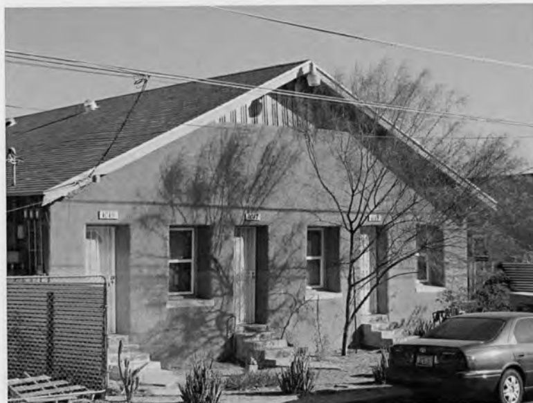
Photograph 2. 1015-1019 S. Meyer Ave.; view east-southeast.
