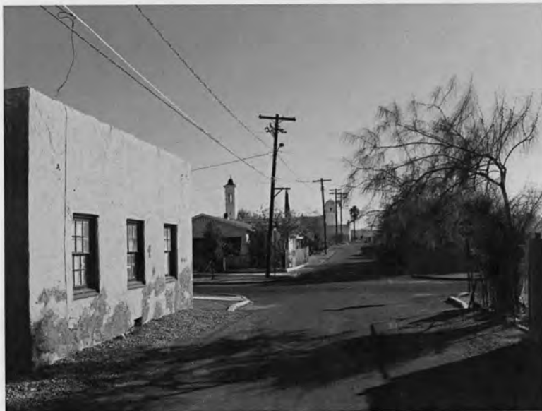
Photograph 18. S. Russell Ave. at W. 21st St.; view south-southeast.
