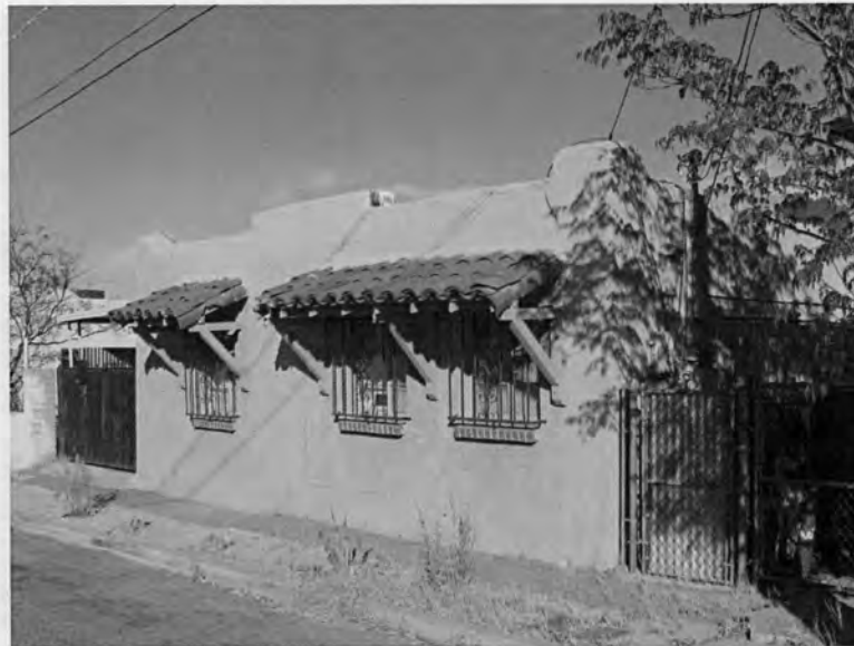
Photograph 8. 126 W. Armijo St.; view northwest.
