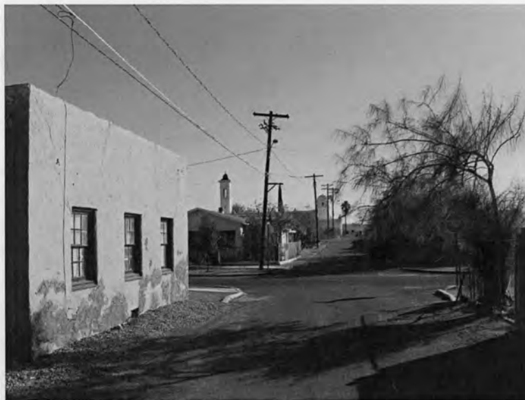
Photograph 20. S. Russell Ave. at W. 21st St.; view south-southeast.
