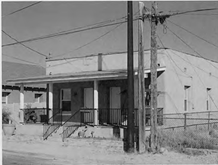
Photograph 3. 1023-1025 S. Meyer Ave.; view east-northeast.
