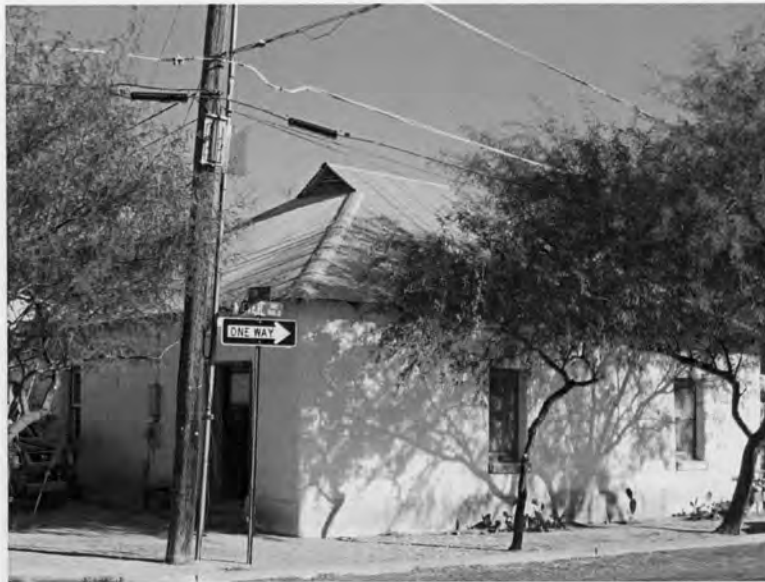
Photograph 11. 901 S. Meyer Ave.; view east-southeast.
