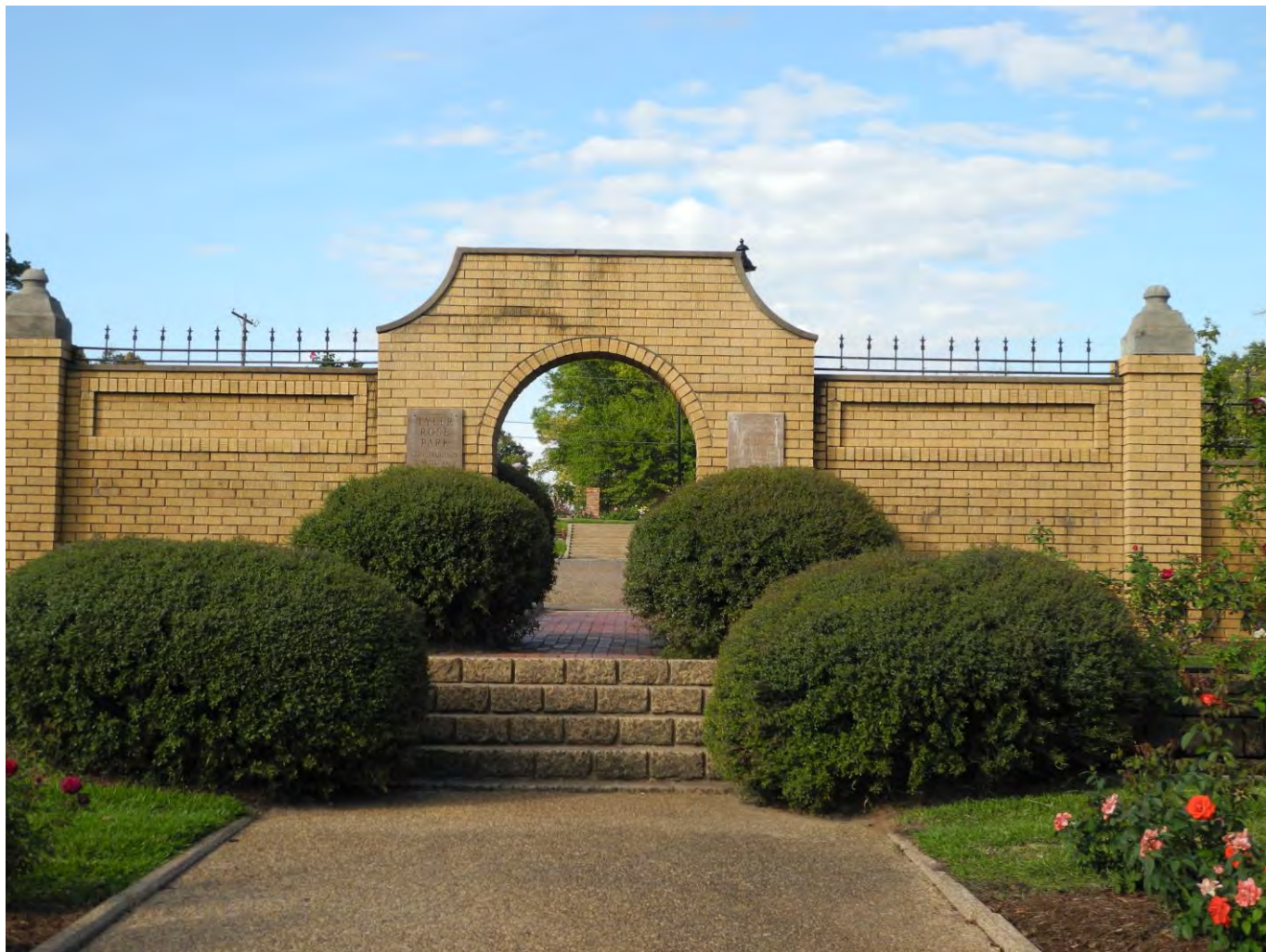
Photo 1: View of Wall with dedication plaques built by WPA c. 1938. Camera facing north.
