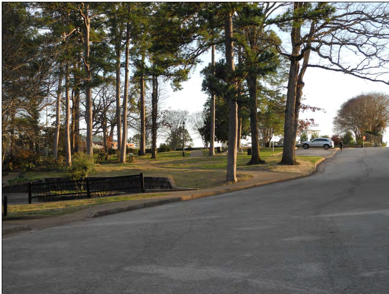
Photo 20: Site 17 – Driveway and parking area, built 1952 to access garden floor and Smith Memorial Building (razed). Camera facing southwest.
