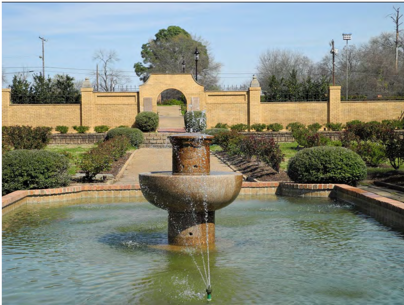
Photo 12: Site 9 – Reflecting Pool, Fountain and Wall built by WPA c. 1938. Camera facing north.
