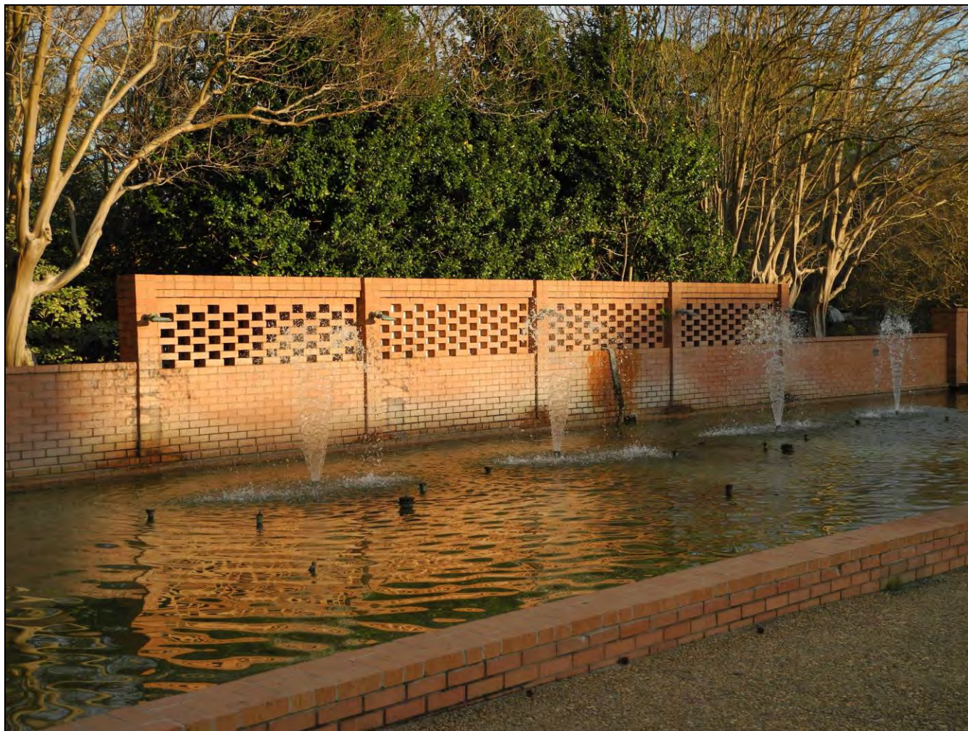
Photo 6: Site 2 - Brick Wall and fountain at rear of Queen's Court lawn, built c. 1960. Camera facing southeast.
