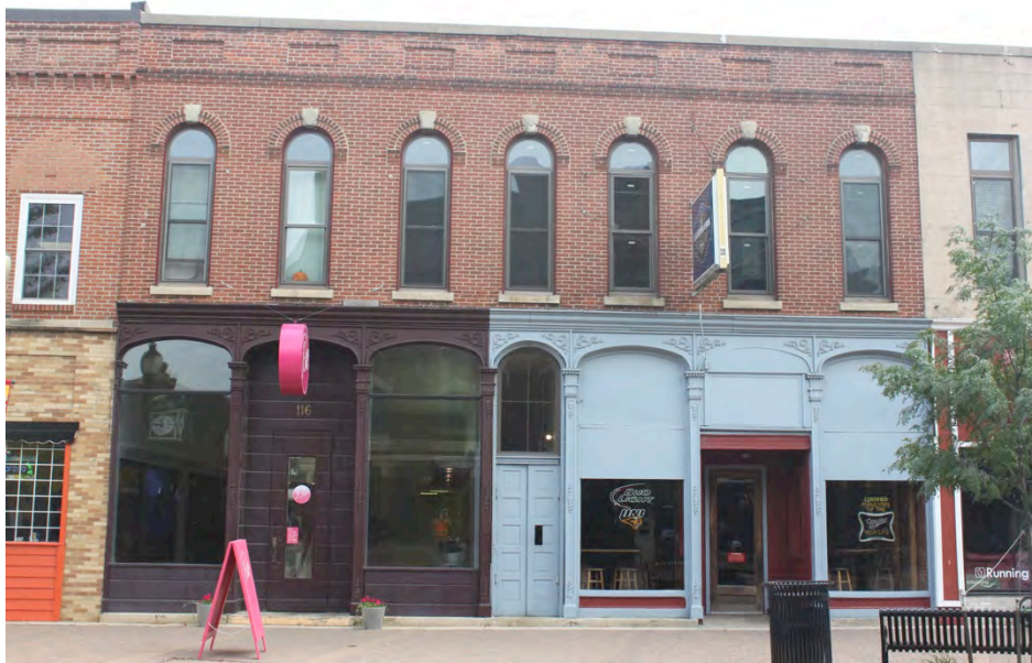
Figure 14: View of Severine & Price Block, 116–118 Main Street. Note Cast-iron storefront detailing. 2016 Photograph.
