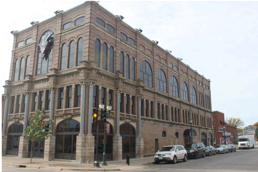
Figure 30: View of I.O.O.F. Temple, 401 Main Street. 2016 Photograph.
