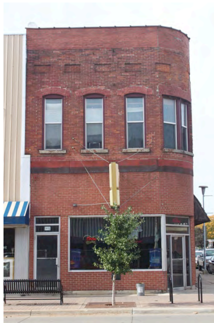
Figure 19: View of 201 Main Street. 2016 Photograph.
