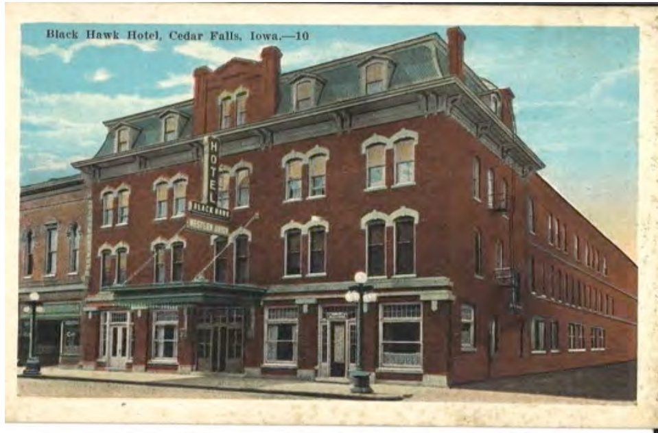
Figure 10: Postcard of Black Hawk Hotel after renovation, circa 1920. Source: Cedar Falls Historical Society.
