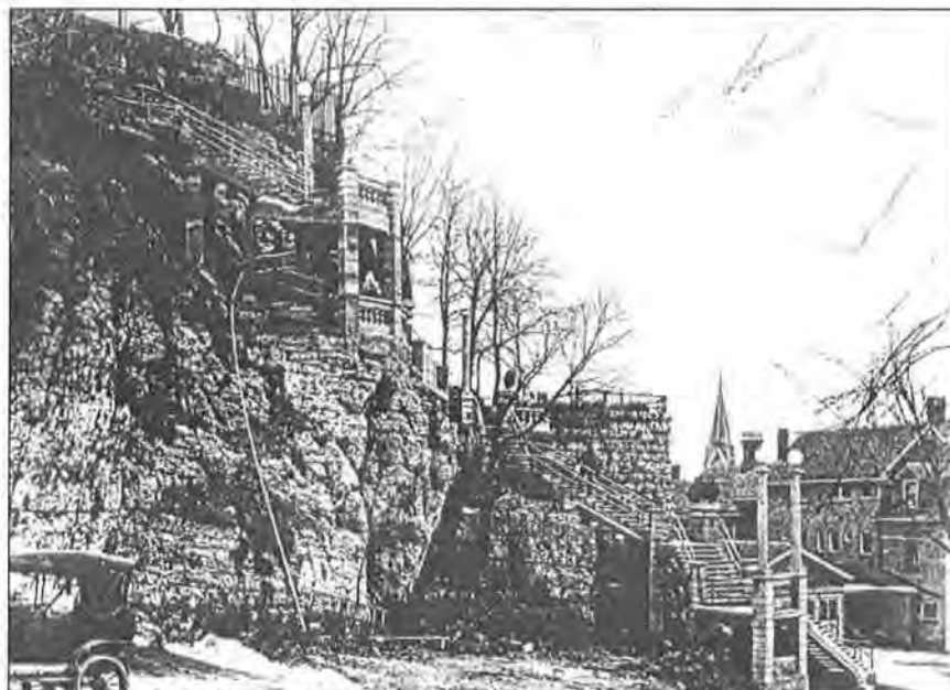
Figure 16: Madison Park Steps, view east, c.1918 (Center for Dubuque History, Loras College)
