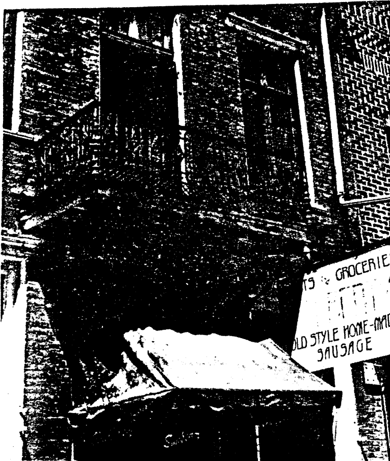
(Note) Balcony on the Gilbertz Building shows the ornamental iron grillwork popular during this period. In earlier days a cigar factory was in this building, today it remains a meat market.
