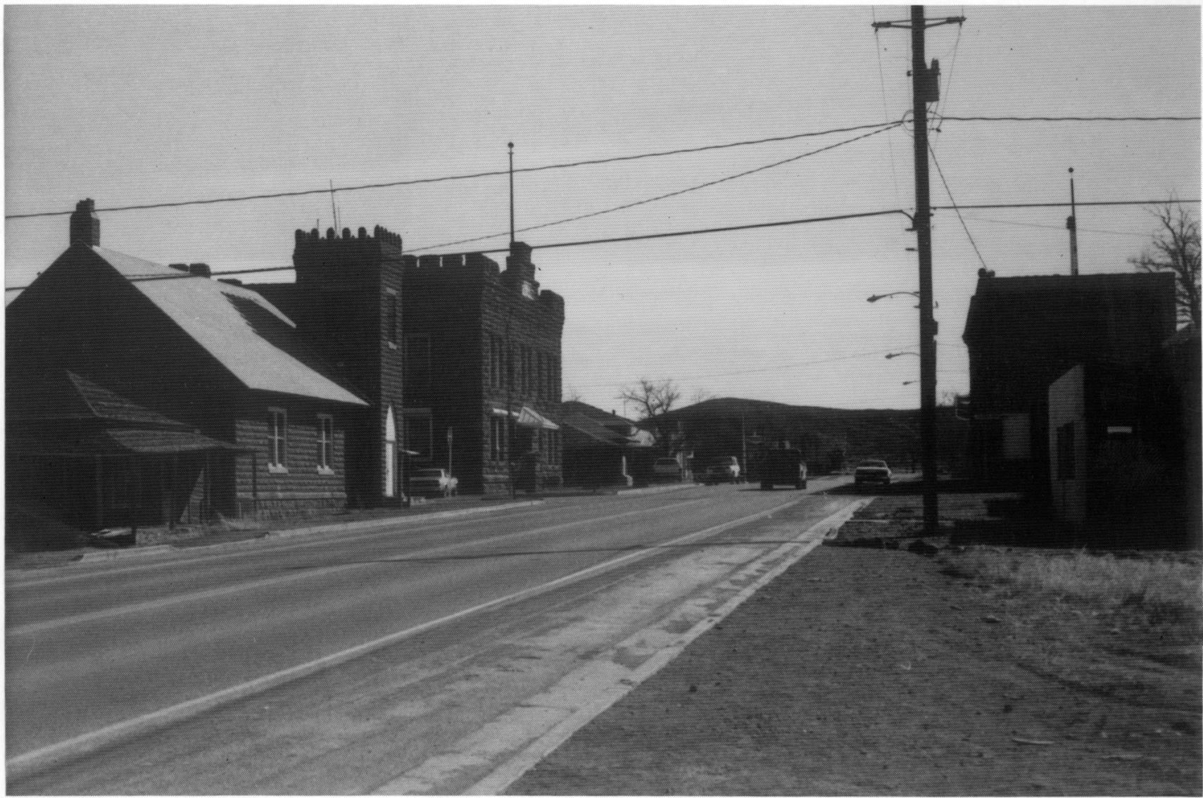
PHOTO # 8. CROOK AVENUE, LOOKING EAST. MAY 1981 JANUS ASSOCIATES PHOTO
