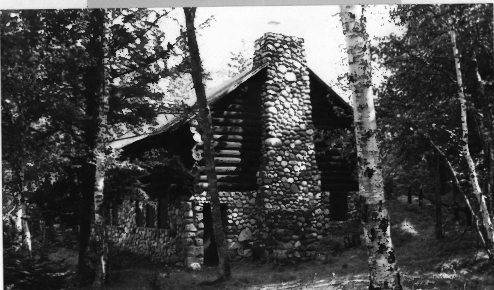
VIEW TO NORTHEAST
