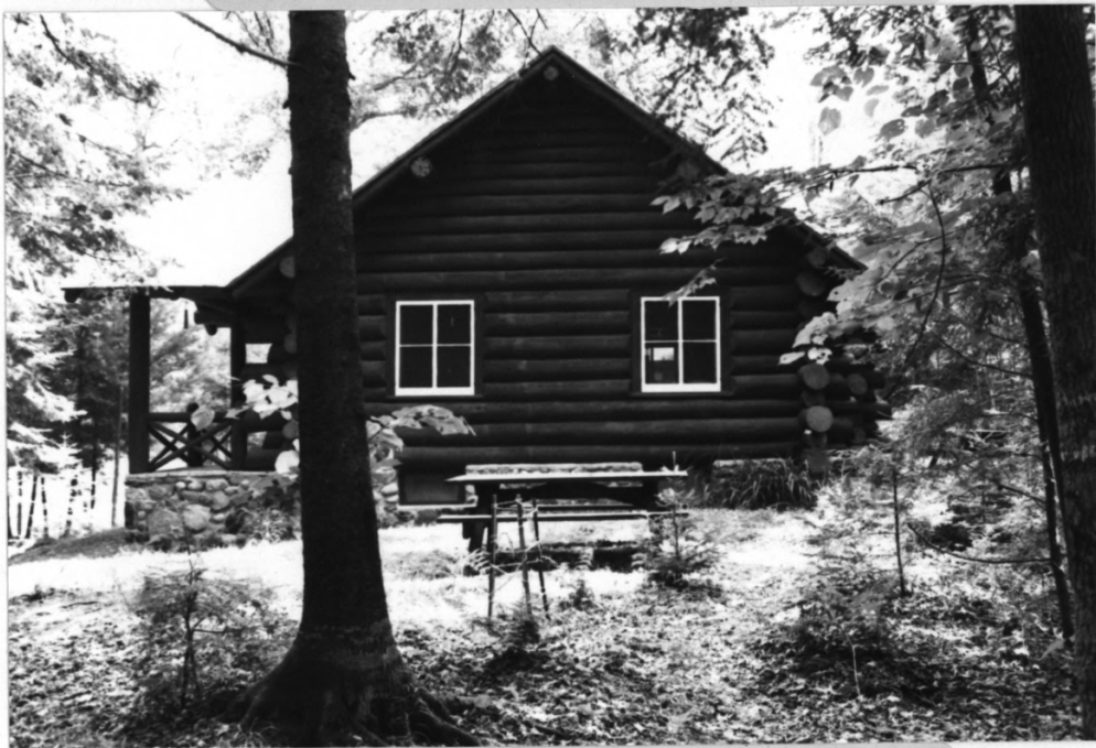
VIEW TO NORTHEAST
