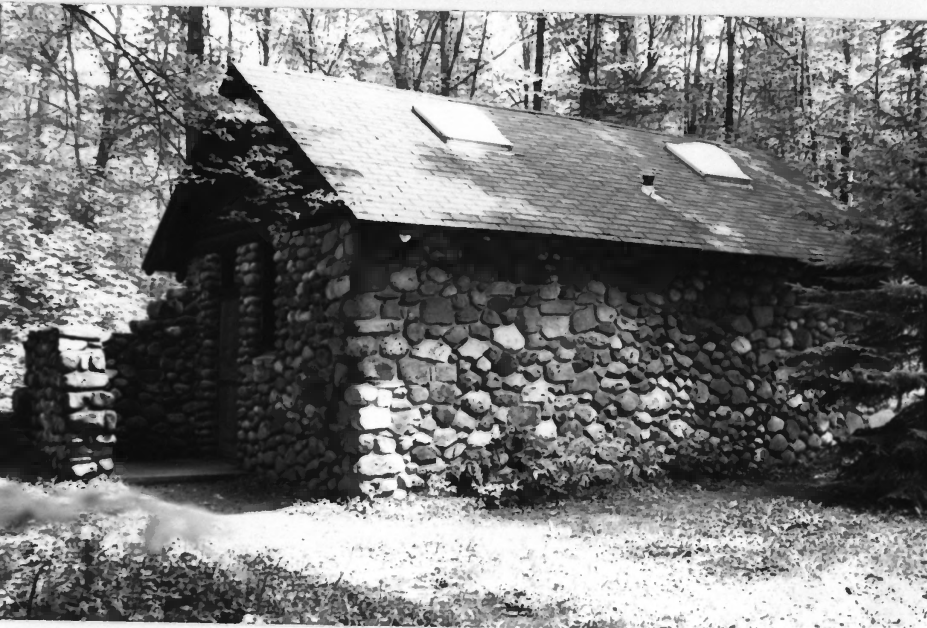
VIEW TO NORTHEAST
