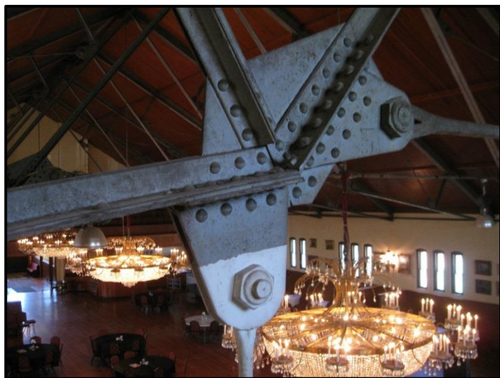
Figure 12. Scissors Joint in Truss Supporting Roof of Drill Shed, 2016.
