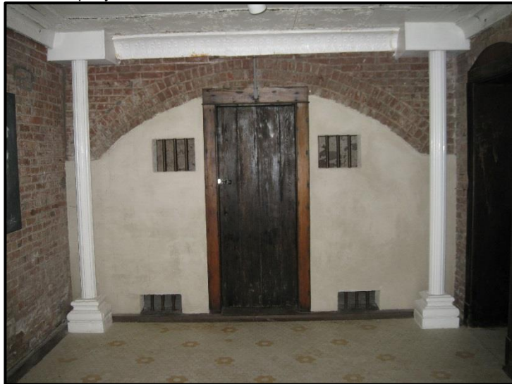
Figure 6. Basement Ammunition Storage, 2016.
