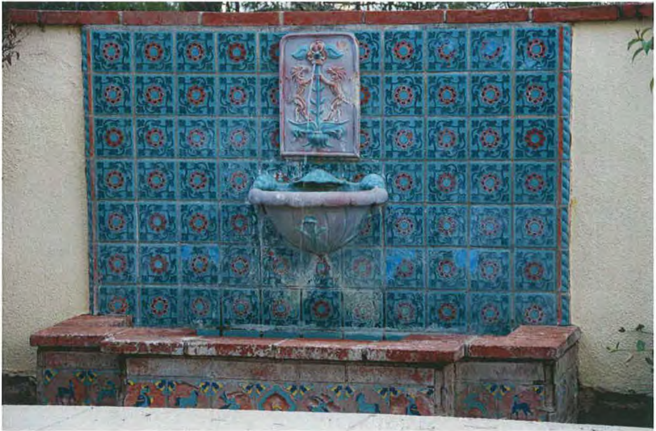
AZ_PimaCounty_BauderHouse_0017: Rear yard original wall fountain detail
