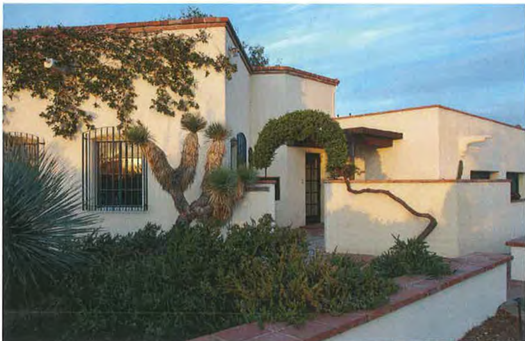
AZ_PimaCounty_BauderHouse_0014: Service entrance facing west
