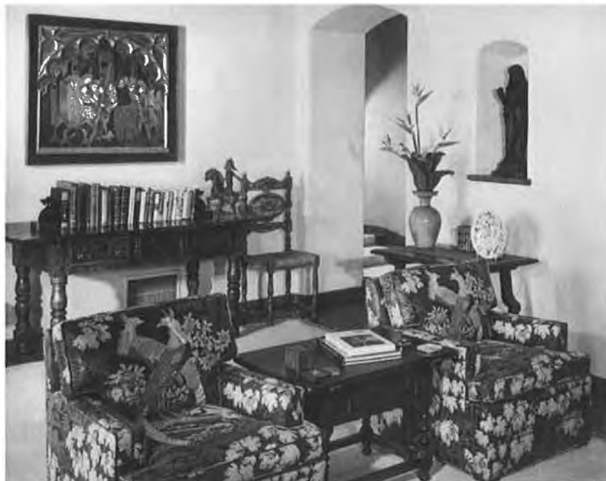
AZ_PimaCounty_BauderHouse_0004: Living room facing southeast towards living quarters hall
