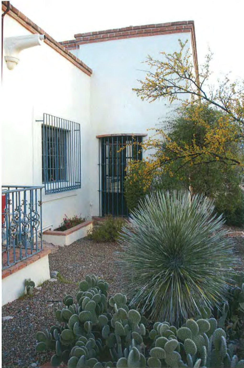
AZ_PimaCounty_BauderHouse_0015: Front view of library and living room facing north
