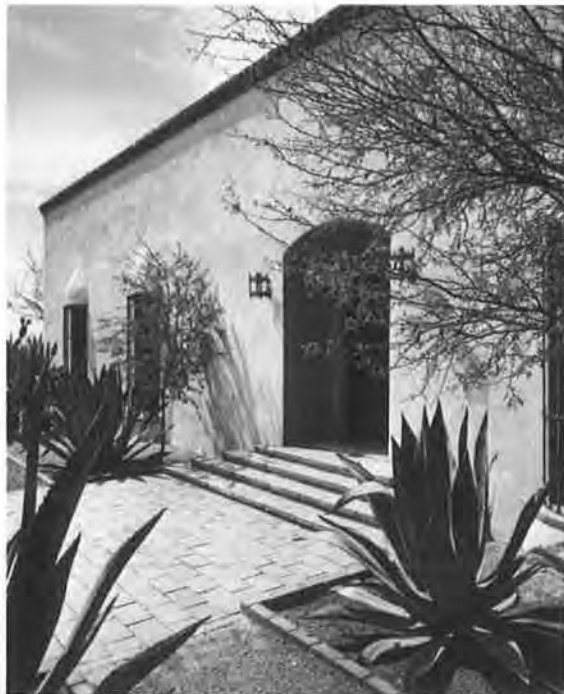
AZ_PimaCounty_BauderHouse_0003: Front entry facing southeast
