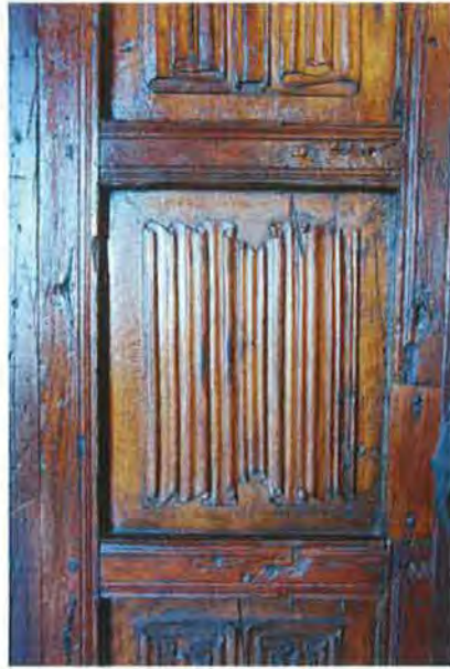
Fig. 27, salvaged 14th century panel doors in dining room
