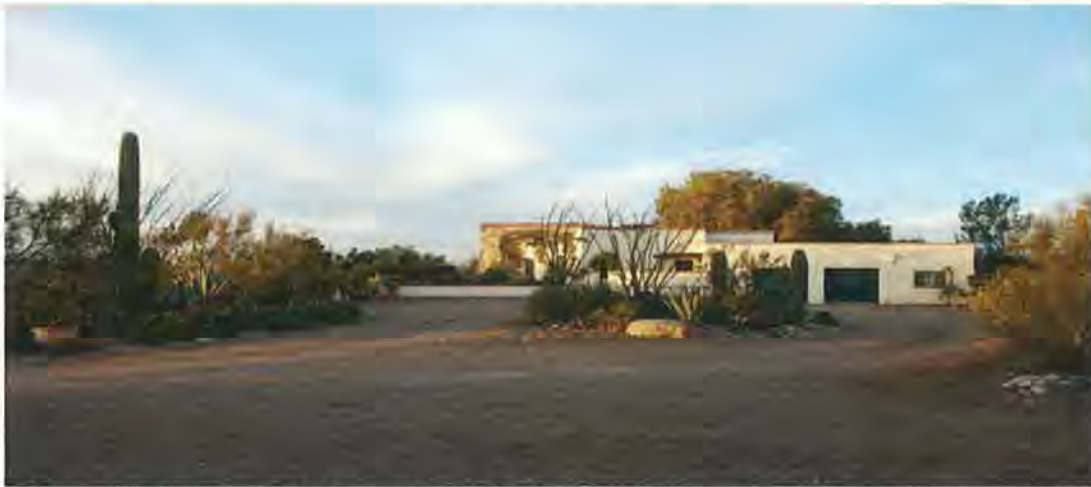
Fig. 3, Entrance drive, camera facing south towards north elevation
