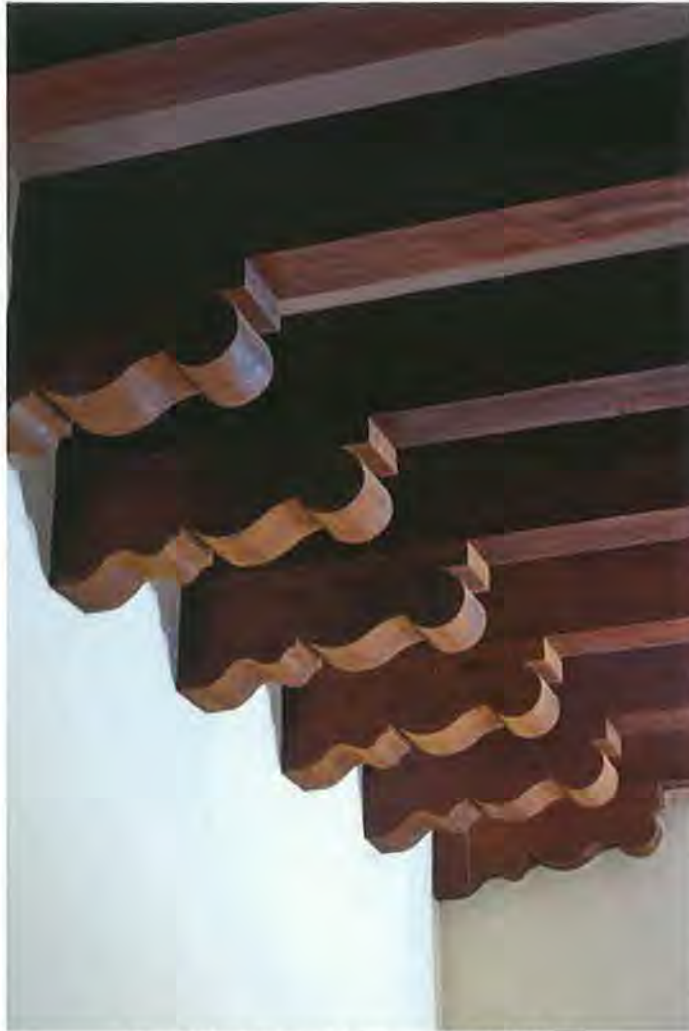
Fig. 34, living room beam and corbel detail
