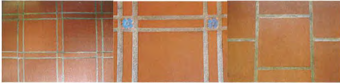
Fig. 22, 23 & 24, Floor details in library, dining and living rooms
