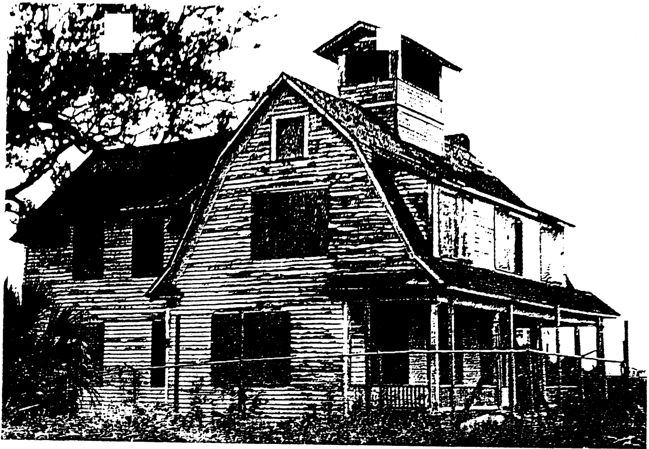
P 1. Northwest corner of house (camera faces southeast) Jan. 1989
