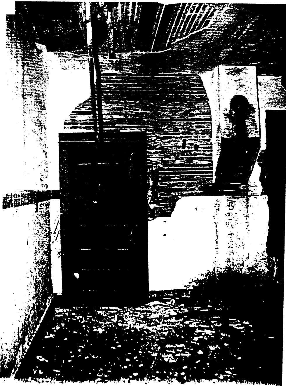
P7. Kitchen; note deteriorated condition of ceiling, wall and door. Also note physical damage caused by fallen limb and moisture damage from rain entering the house. (camera faces east) March 1990
