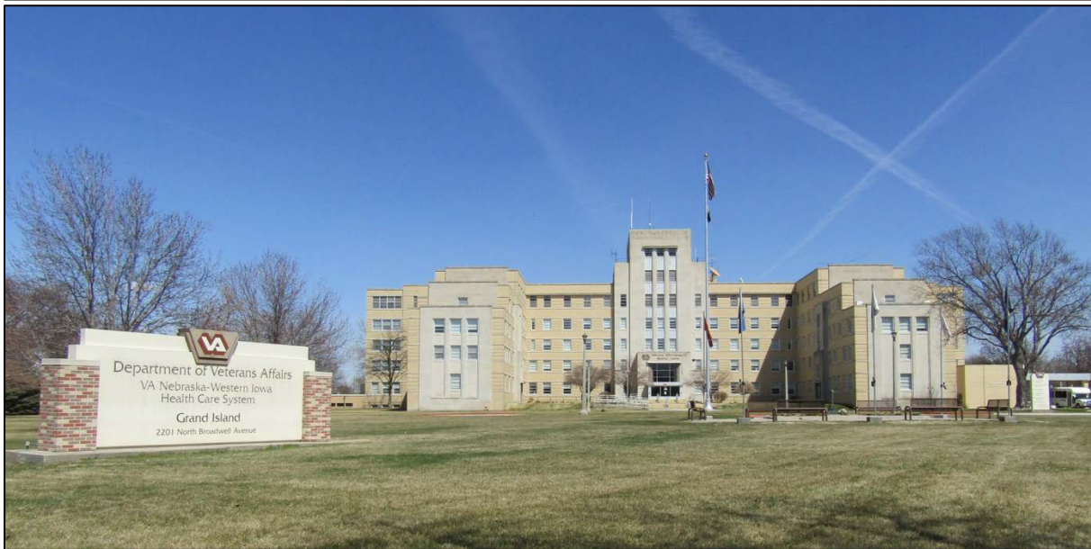
Figure 5. (above) View looking east to the main hospital, 1950 (VA), and view of the southwest (front) façade, 2018 (Linda E. Williams, Engineering Technician, COR VA).
