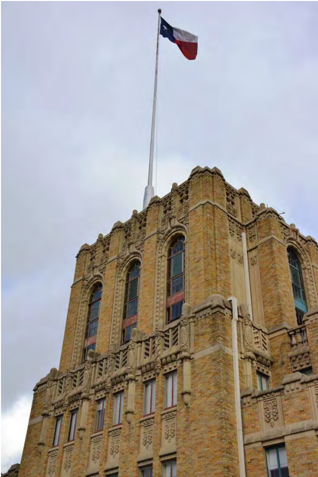
TX_Bexar County_Milam Building_0009.tif 21st floor looking northwest
