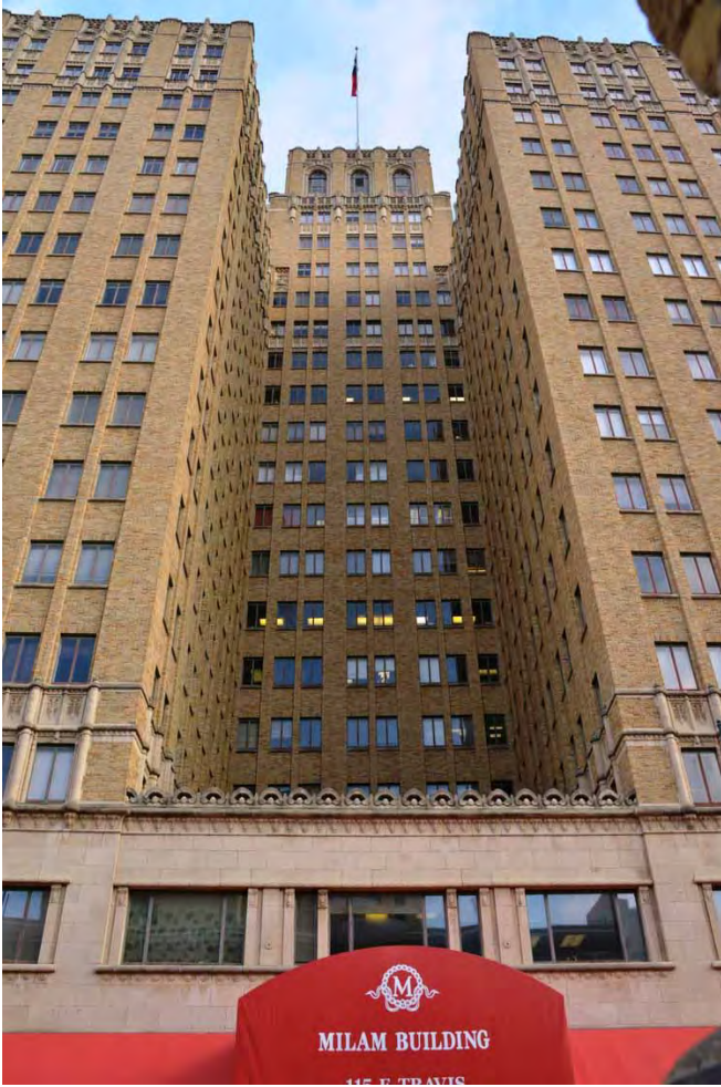
TX_Bexar County_Milam Building_0002.tif south elevation looking north
