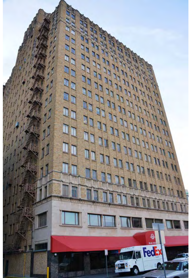
TX_Bexar County_Milam Building_0003.tif west elevation looking southeast
