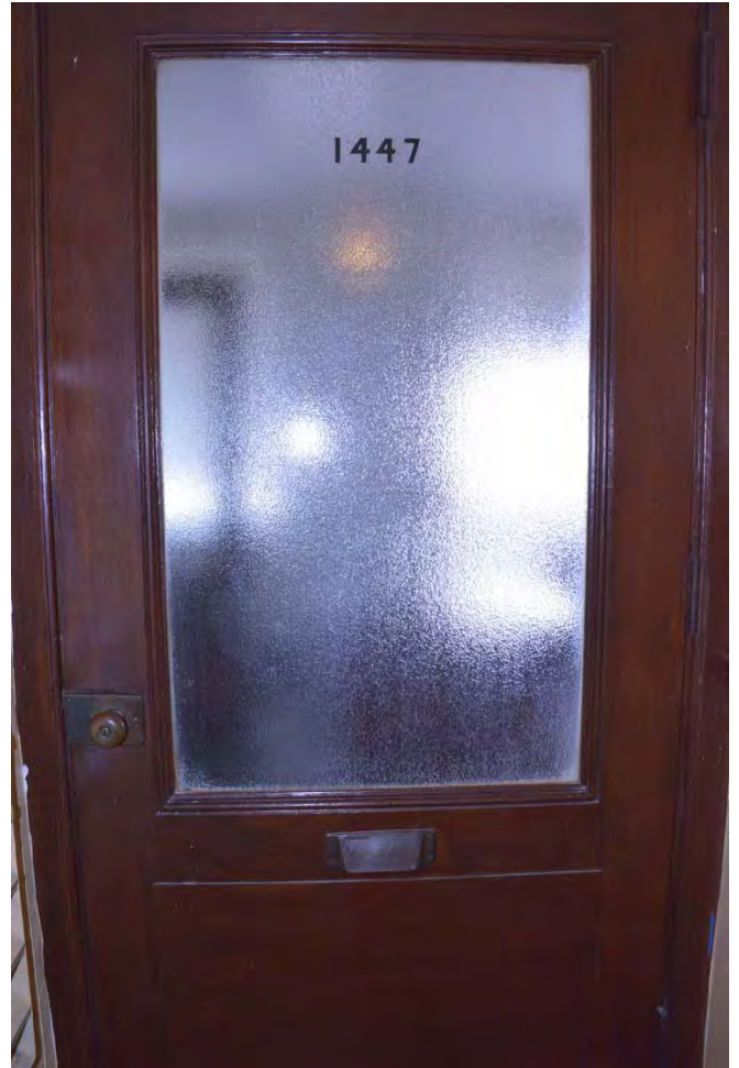
TX_Bexar County_Milam Building_0022.tif original office door and hardware
