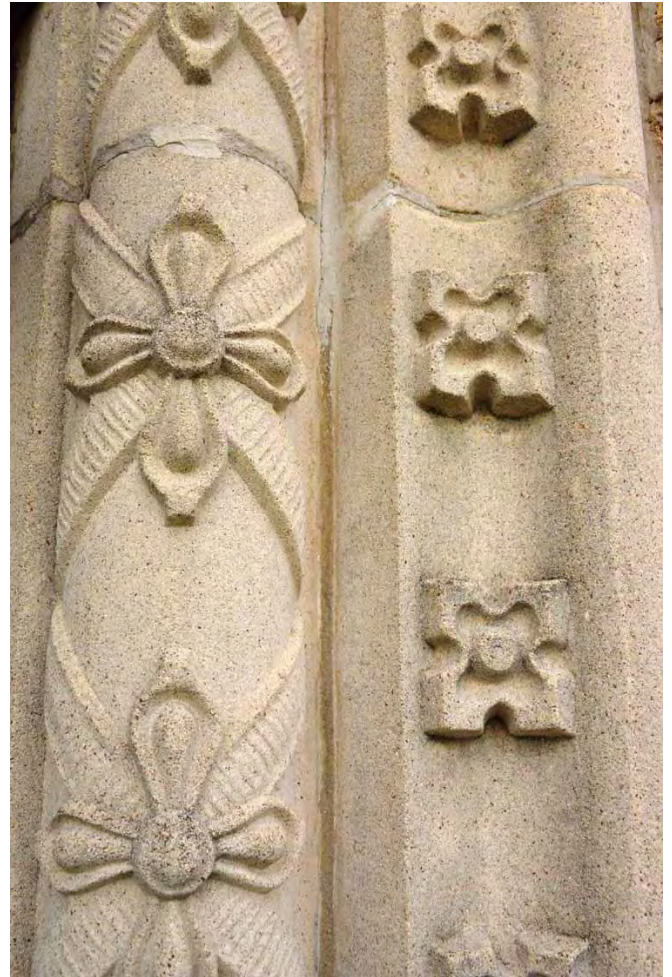
TX_Bexar County_Milam Building_0010.tif cast stone detailing
