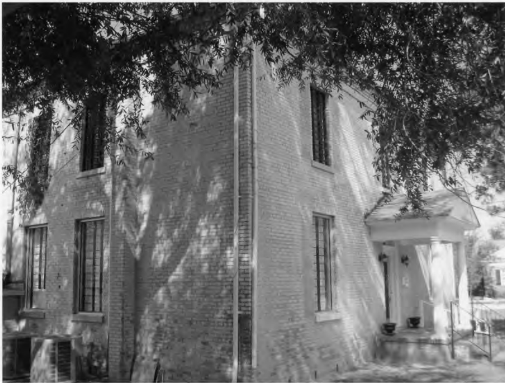
3. Hampton County Jail 701 1 st Street West, Hampton Hampton County, South Carolina
