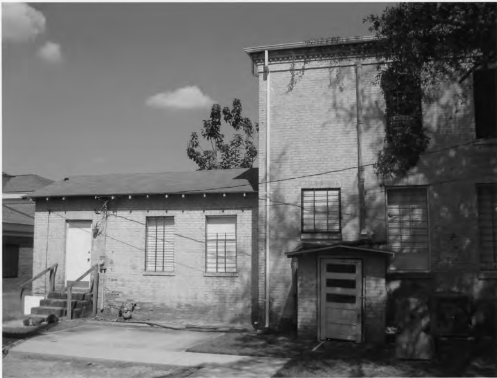
4. Hampton County Jail 701 1 st Street West, Hampton Hampton County, South Carolina
