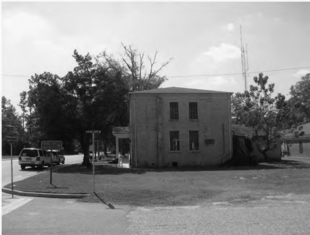
11. Hampton County Jail 701 1 st Street West, Hampton Hampton County, South Carolina
