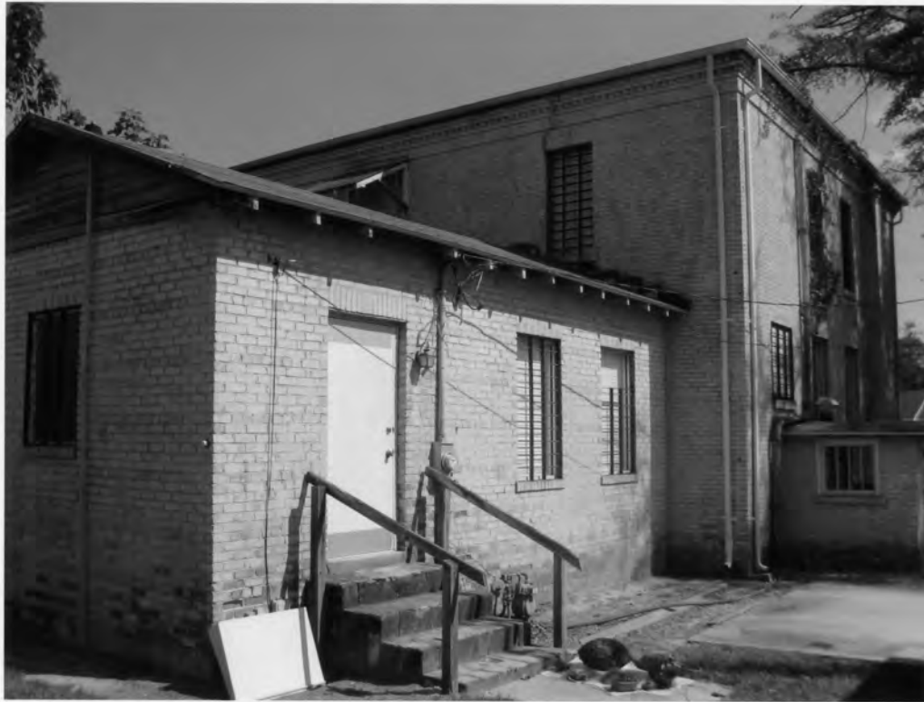
6. Hampton County Jail 701 1 st Street West, Hampton Hampton County, South Carolina
