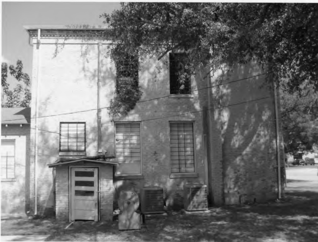
5. Hampton County Jail 701 1 st Street West, Hampton Hampton County, South Carolina
