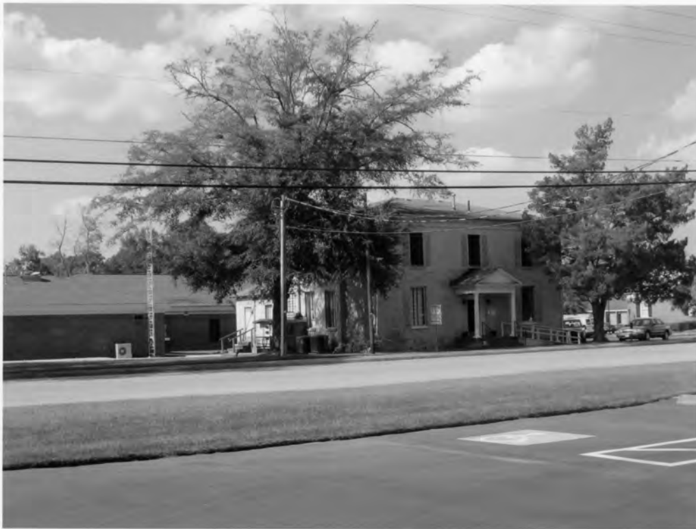
30. Hampton County Jail 701 1 st Street West, Hampton Hampton County, South Carolina
