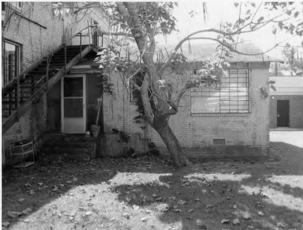
8. Hampton County Jail 701 1 st Street West, Hampton Hampton County, South Carolina
