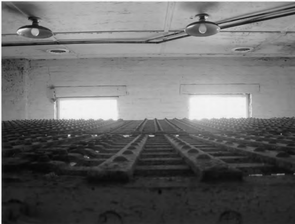
26. Hampton County Jail 701 1 st Street West, Hampton Hampton County, South Carolina
