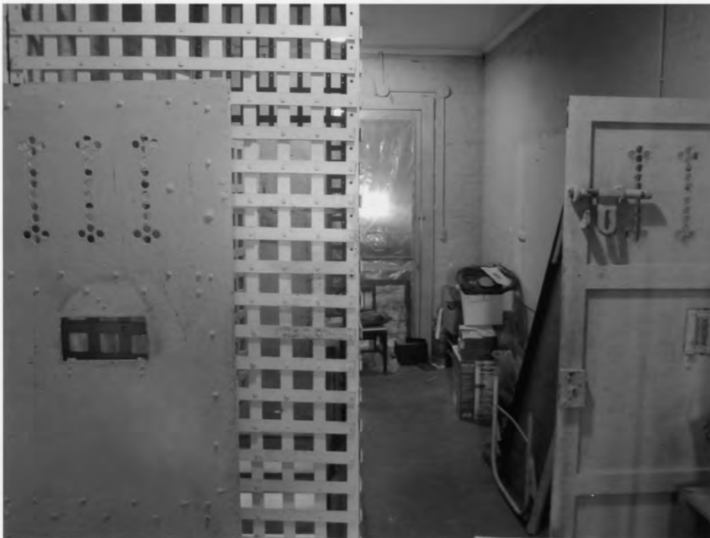
27. Hampton County Jail 701 1 st Street West, Hampton Hampton County, South Carolina
