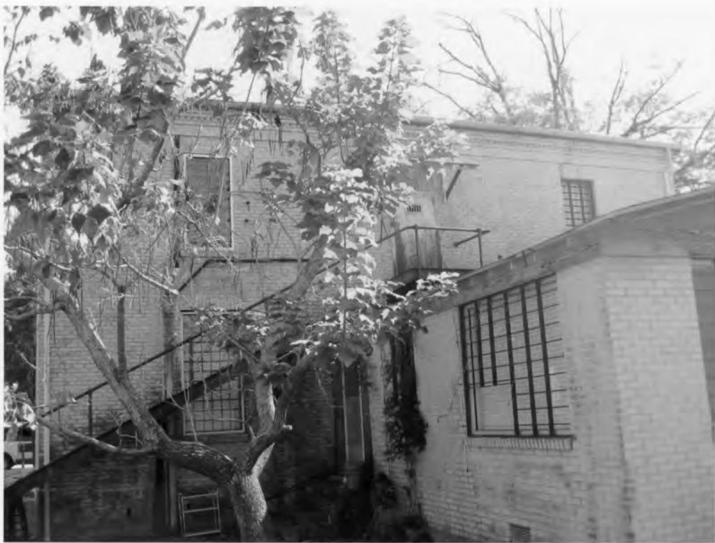
7. Hampton County Jail 701 1 st Street West, Hampton Hampton County, South Carolina
