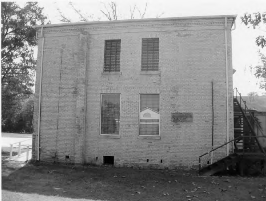
9. Hampton County Jail 701 1 st Street West, Hampton Hampton County, South Carolina
