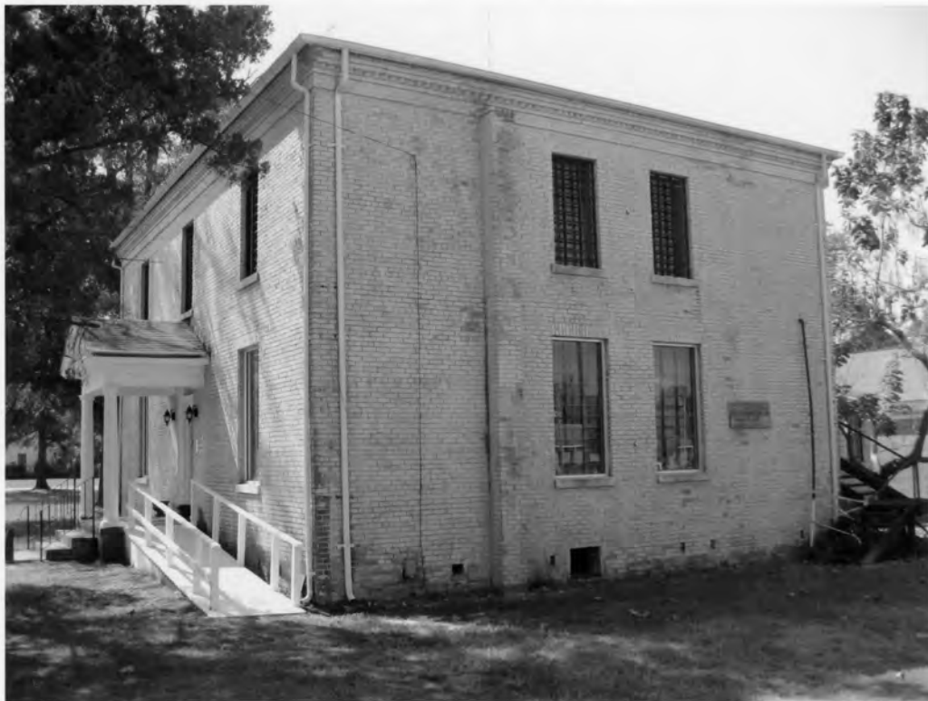
10. Hampton County Jail 701 1 st Street West, Hampton Hampton County, South Carolina
