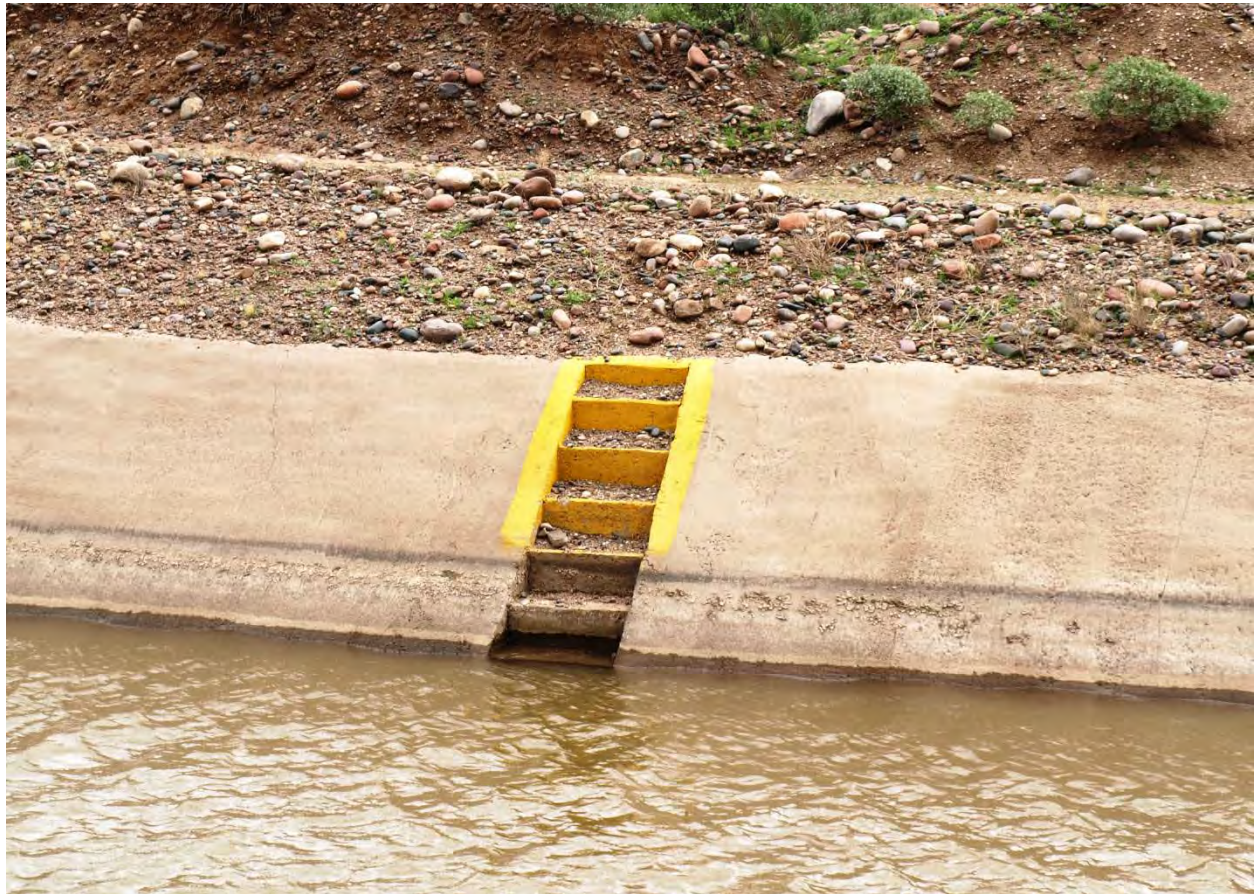
Photo 32. South Canal "horsesteps" detail (same location as Photo 33).
