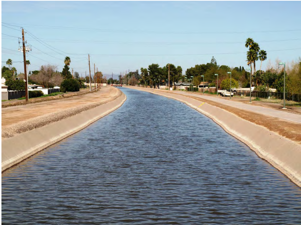
Photo 35. Consolidated Canal at 8 th Street, Mesa looking northwest.
