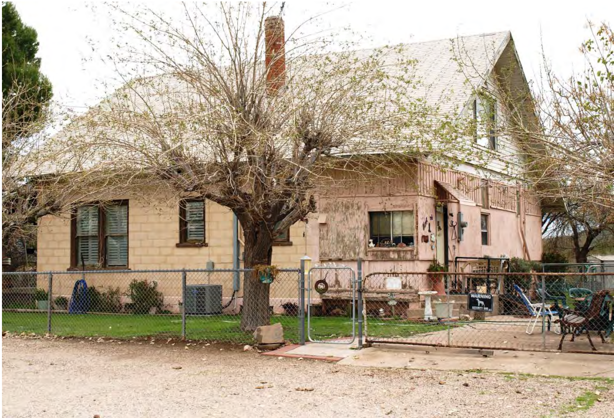
Photo 7. Granite Reef Diversion Dam dam tenders house looking east.
