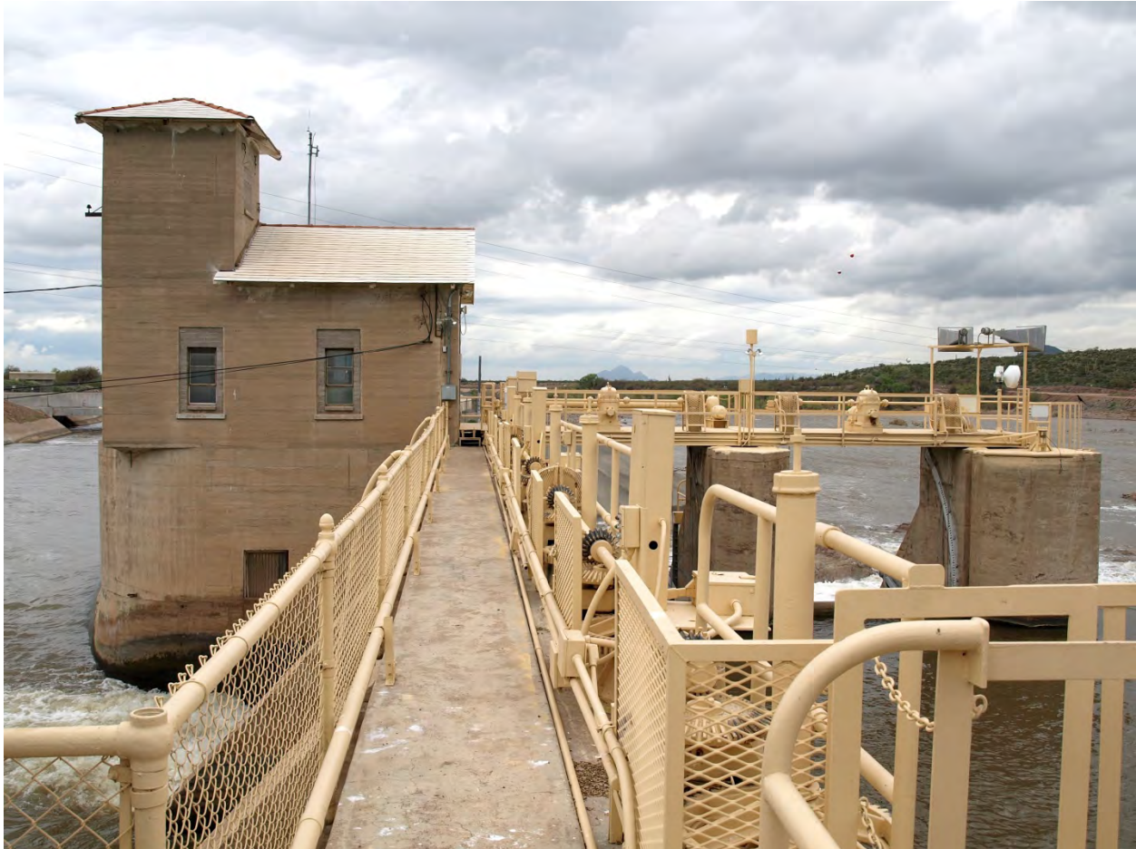
Photo 5. Granite Reef Diversion Dam south side gate structure looking west.
