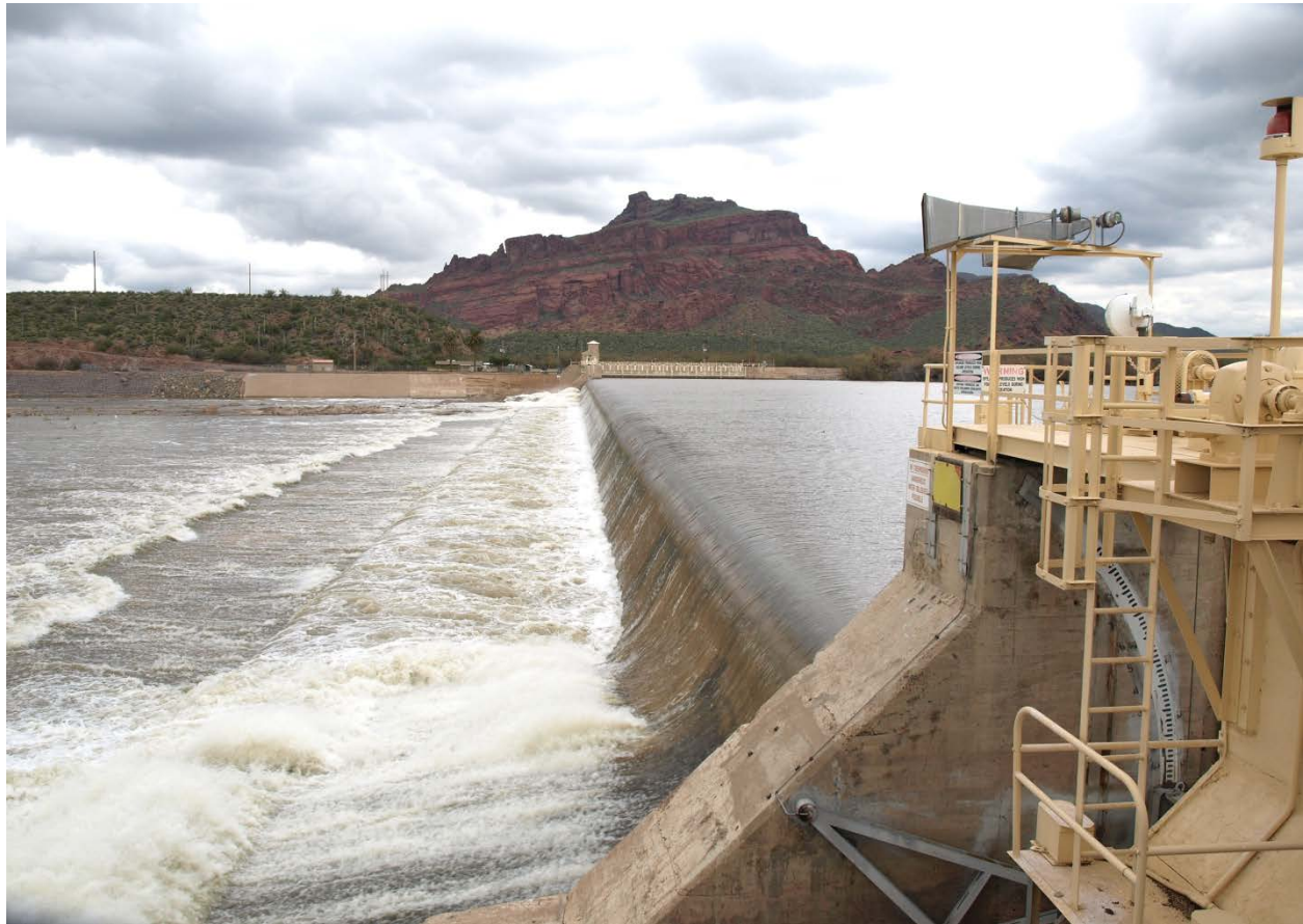
Photo 2. Granite Reef Diversion Dam crest looking north.
