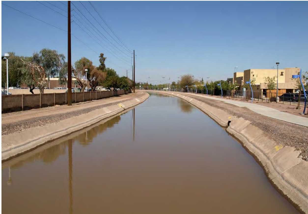
Photo 53. Western Canal at Guadalupe Road looking north.
