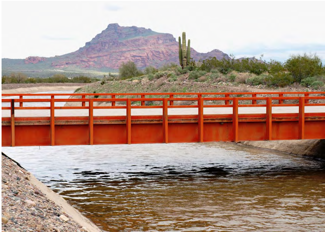
Photo 31. South Canal at Thomas Road in Mesa, looking northeast.
