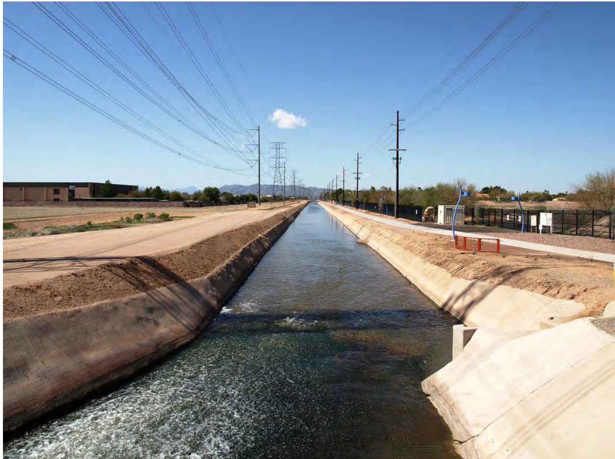
Photo 52. Western Canal at Tempe water treatment plant looking west.
