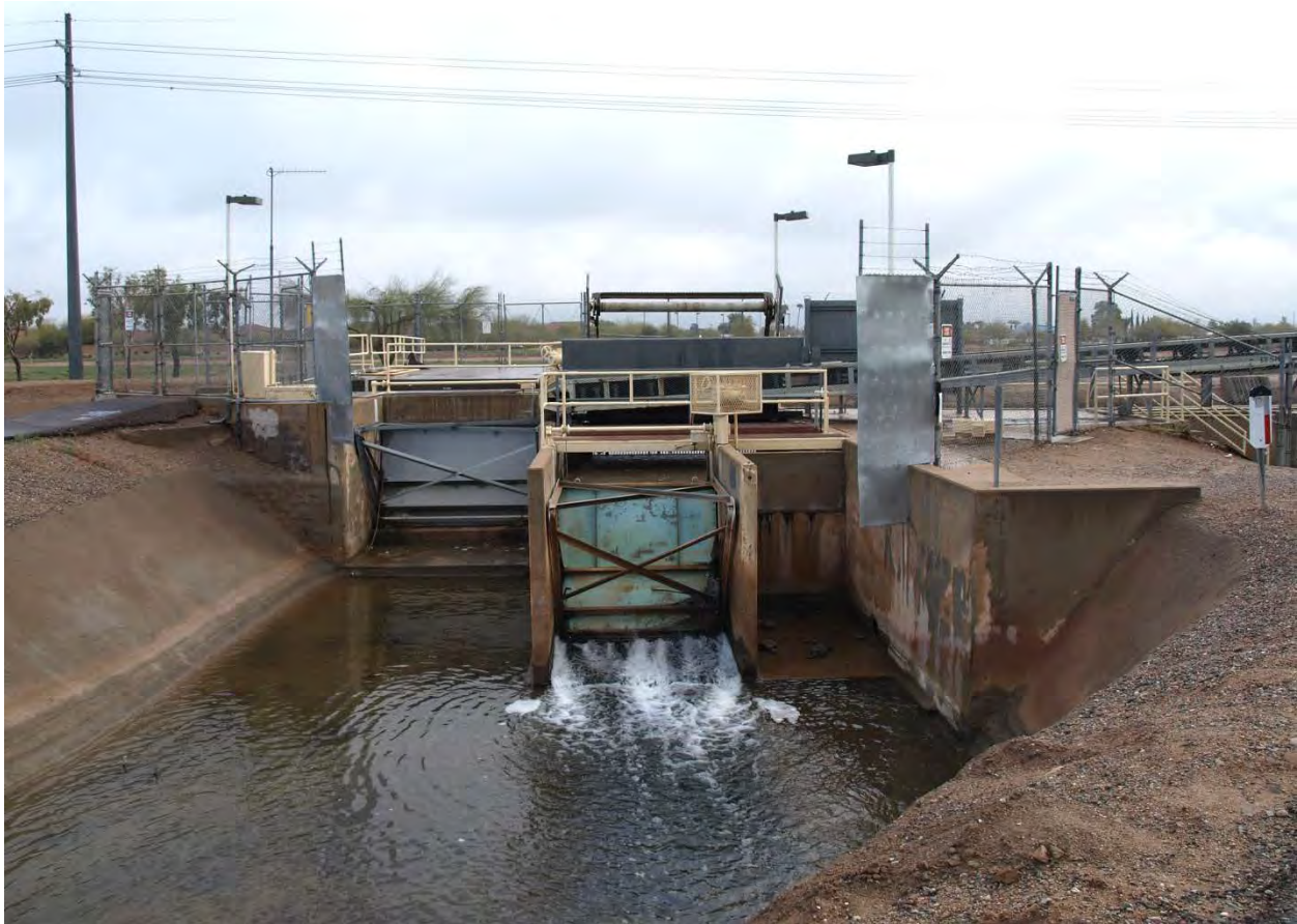
Photo 15. Arizona Canal toe looking northwest.
