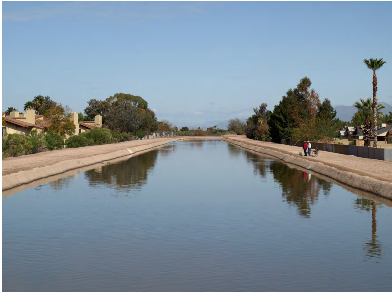
Photo 34. South Canal at Tempe/Consolidated/South canals juncture looking north.
