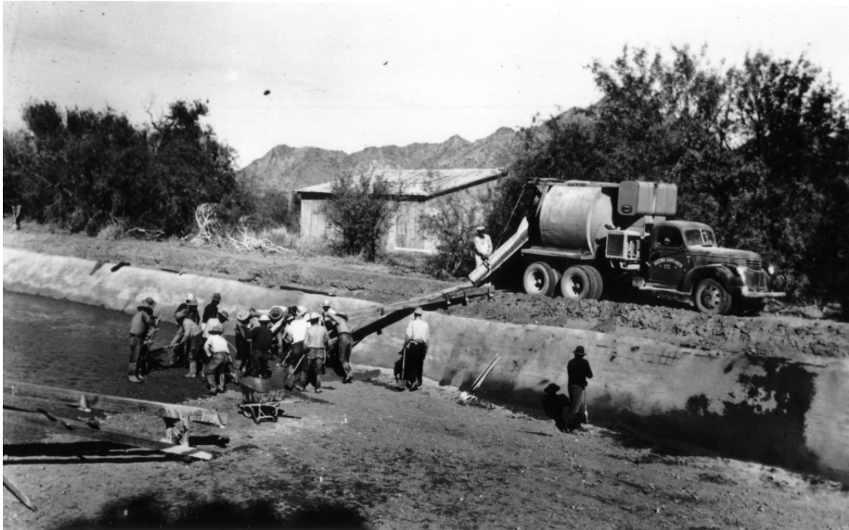
Historic Photo 4. Workers lining the Arizona Canal with concrete, December 1943. Photo courtesy of the SRP.
