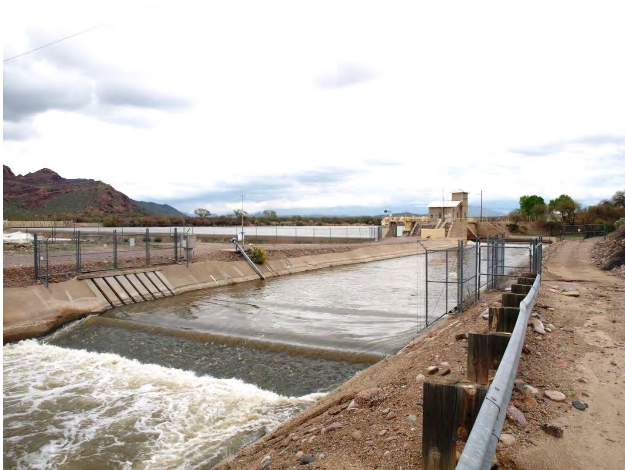
Photo 30. South Canal turnout at Granite Reef Diversion Dam.
