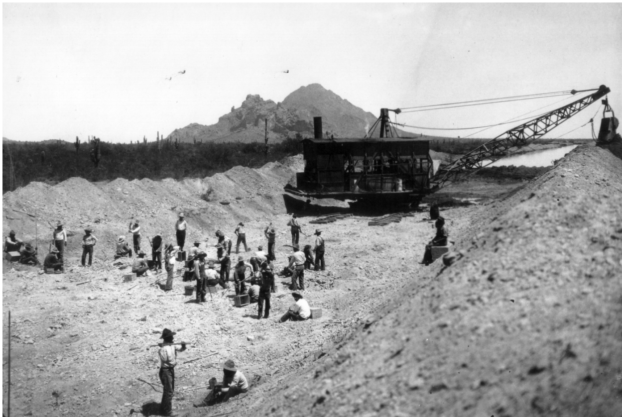
Historic Photo 3. Arizona Canal excavation, eight miles northeast of Phoenix. Undated photo by Walter J. Lubken.
