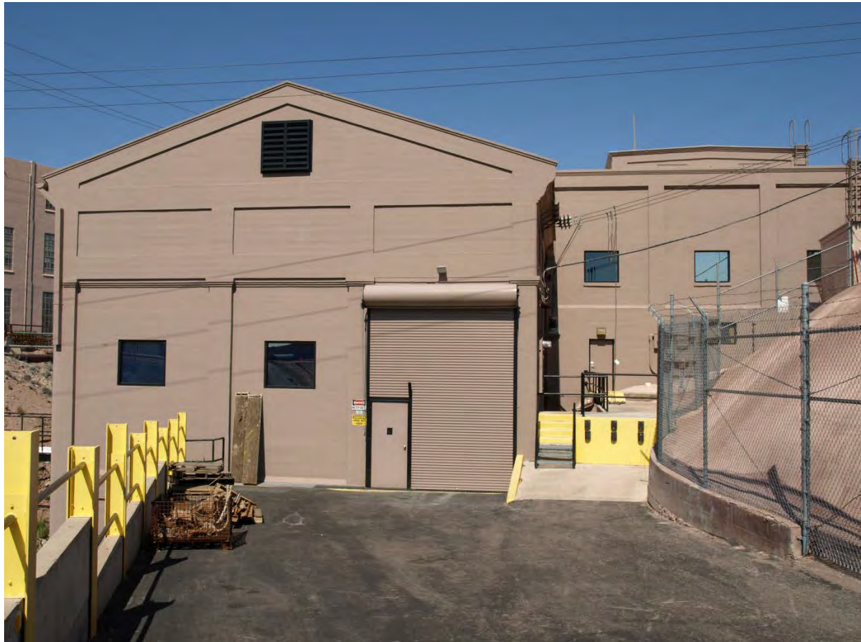
Photo 19. Crosscut Hydro Plant looking north (see site drawing).
