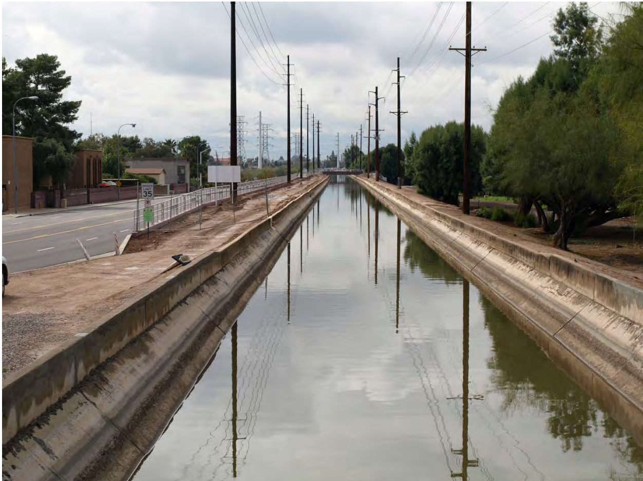
Photo 17. Crosscut Canal at Arizona Canal looking south.
