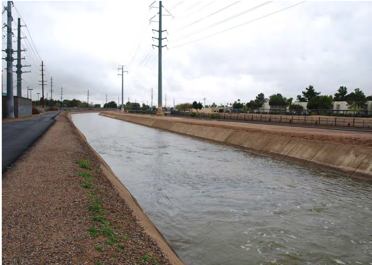
Photo 14. Arizona Canal west of Metrocenter looking west.
