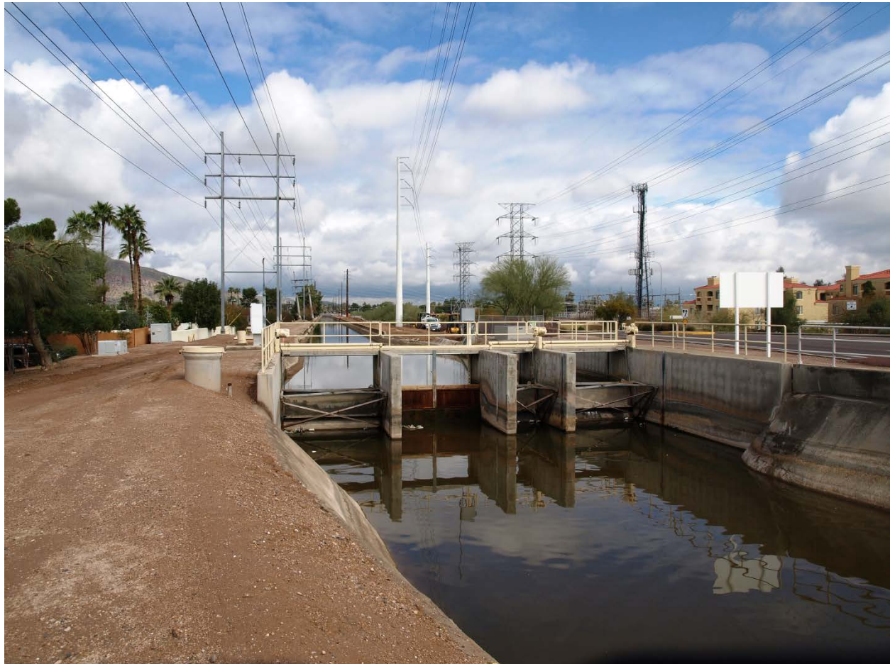
Photo 18. Crosscut Canal check at 64 th Street and Thomas Road looking north.
