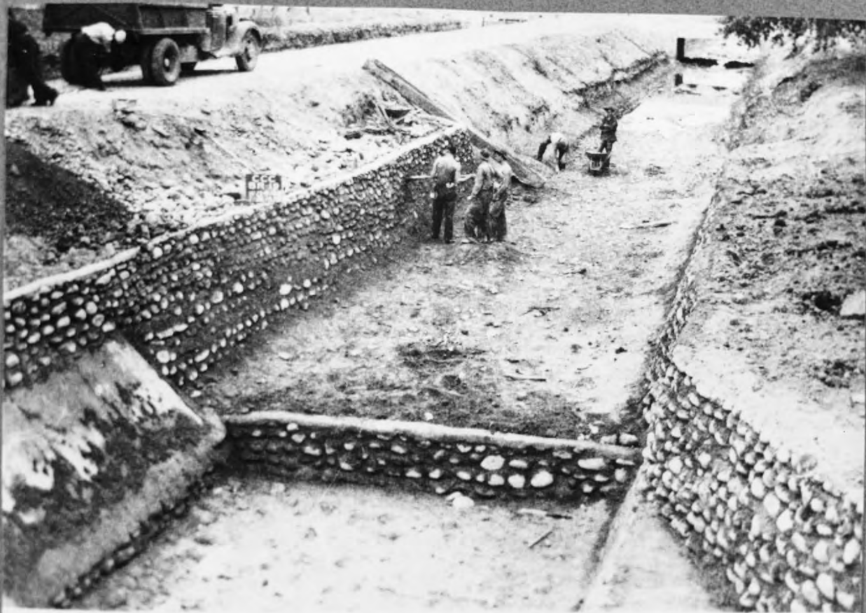
Rubble paving job in Grand Canal at 4E - 10N - January 18, 1938
