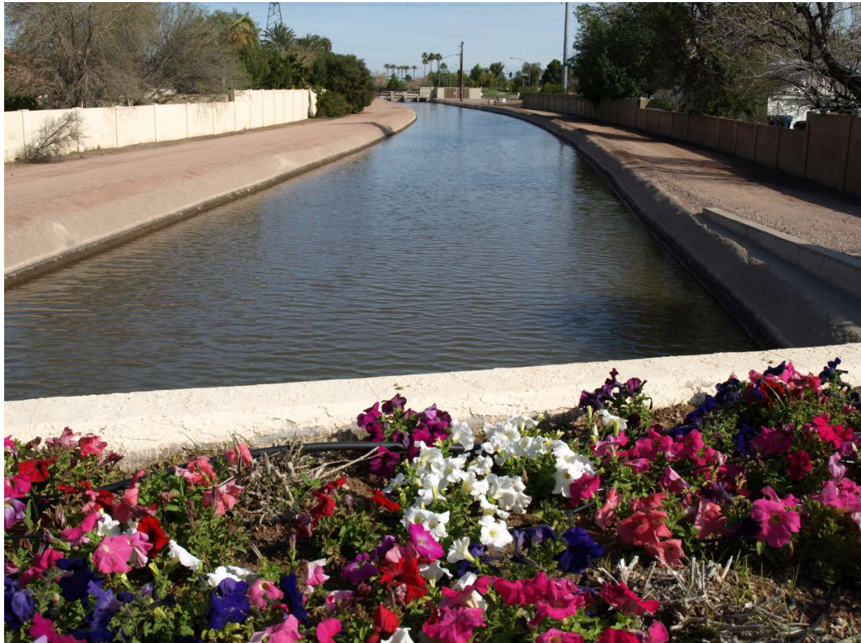
Photo 36. Consolidated Canal at Lindsey Trail, looking north.
