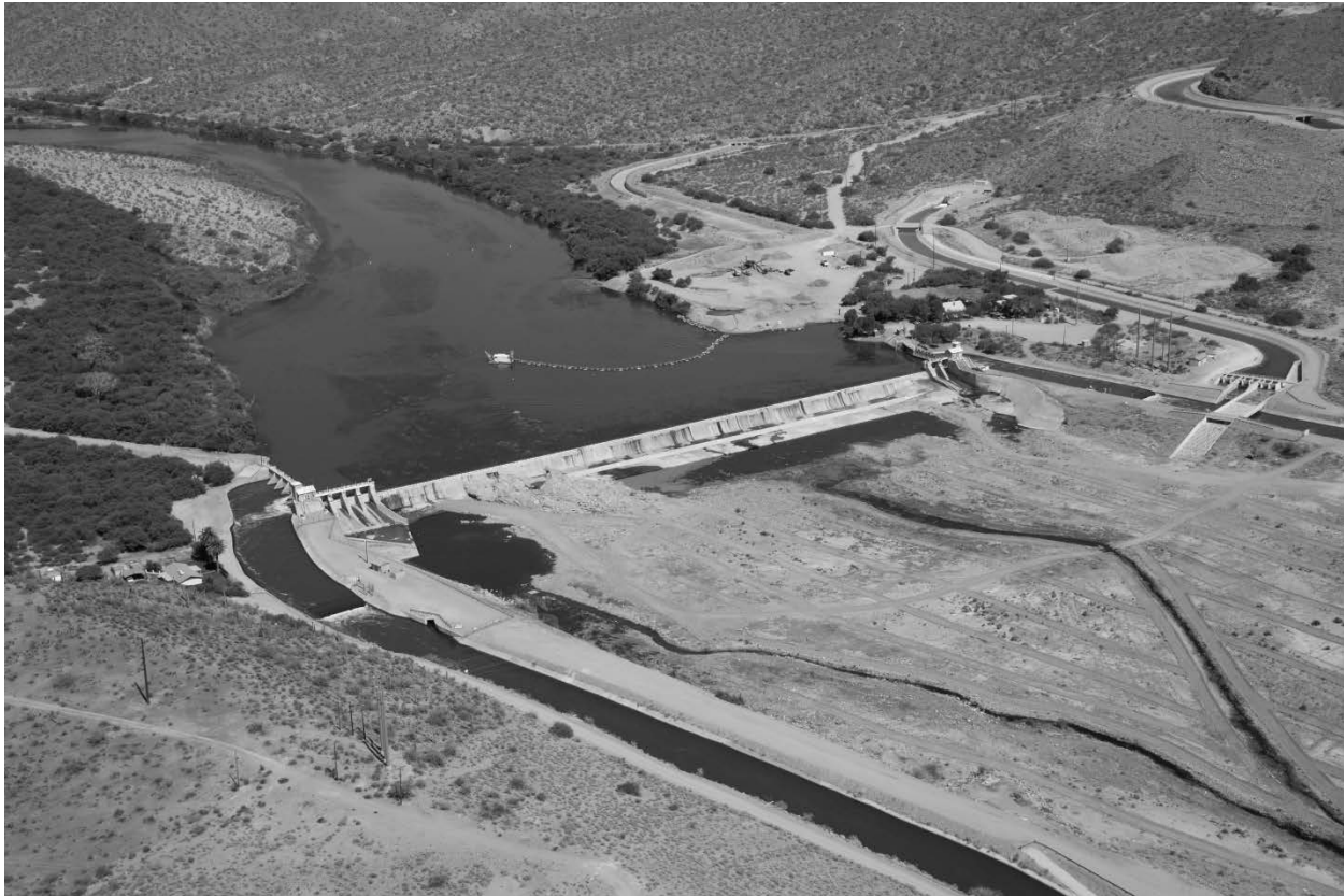
Photo 1. Granite Reef Diversion Dam aerial, 2009. Photo courtesy of the SRP.
