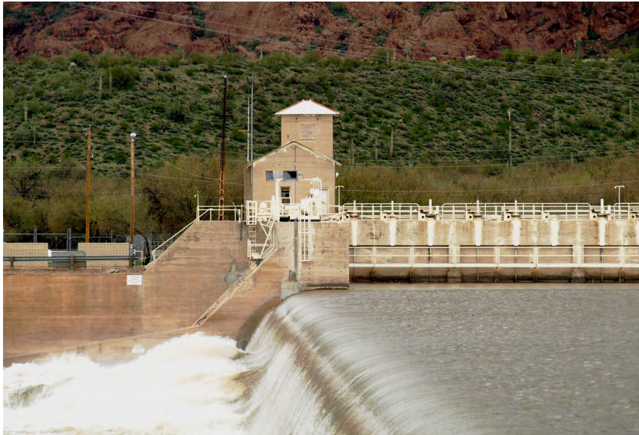
Photo 3. Granite Reef Diversion Dam north side turnout looking north.
