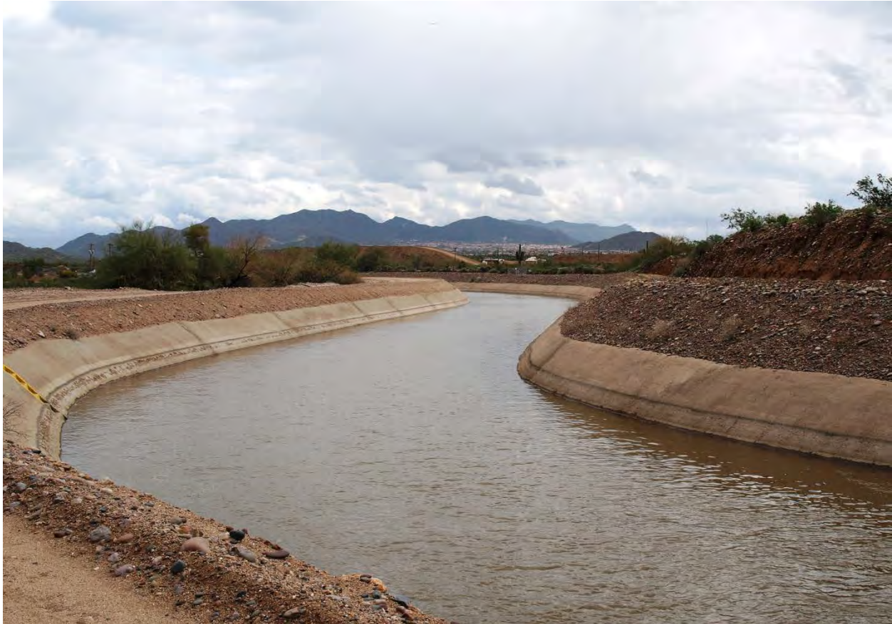
Photo 33. South Canal near McDowell Road looking northeast.
