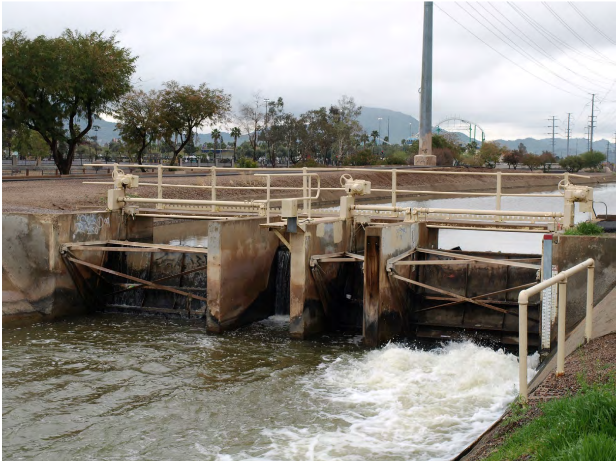
Photo 13. Arizona Canal west of Metrocenter looking east.
