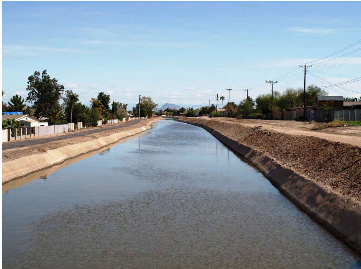
Photo 47. Tempe Canal at Dobson Road looking northeast.
