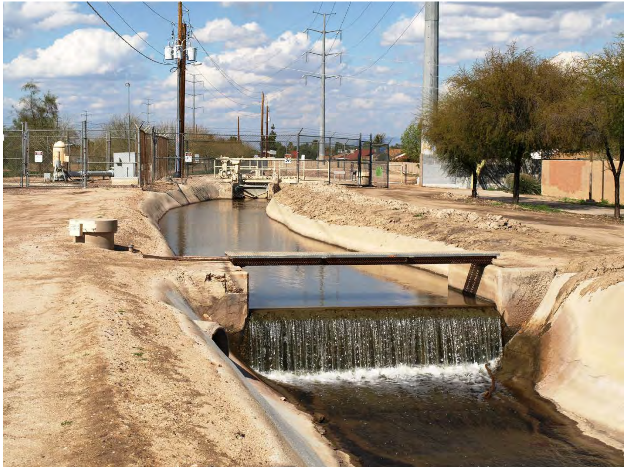
Photo 57. South Highline at Grove Parkway looking north.
