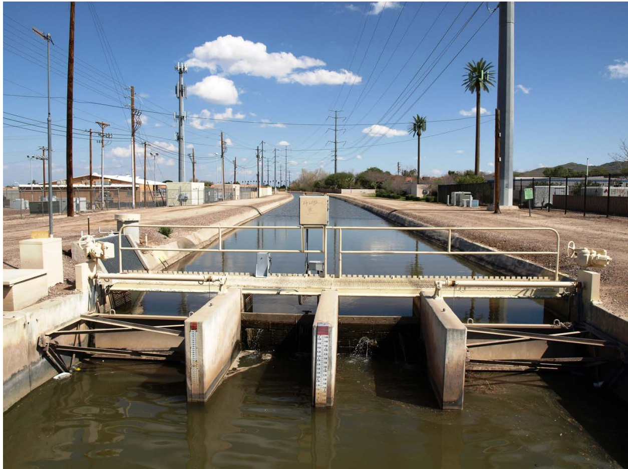
Photo 54. Western Canal check at 16 th Street, Phoenix, looking east.
