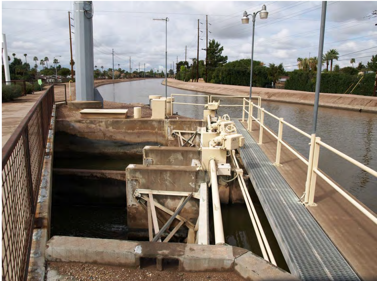
Photo 16. Crosscut Canal turnout at Arizona Canal looking west.
