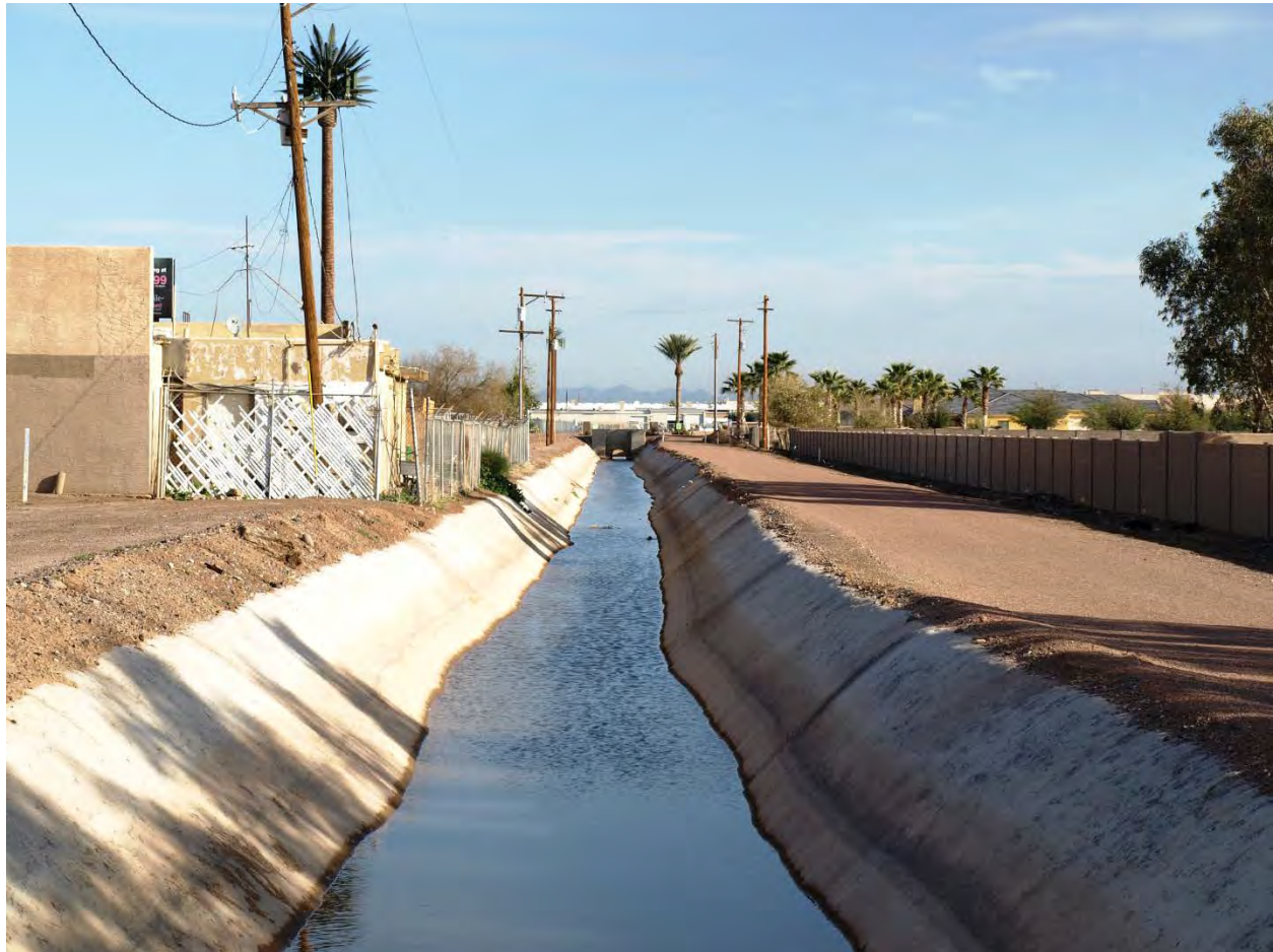
Photo 40. Consolidated Canal toe at Arizona State Route 87 looking north.
