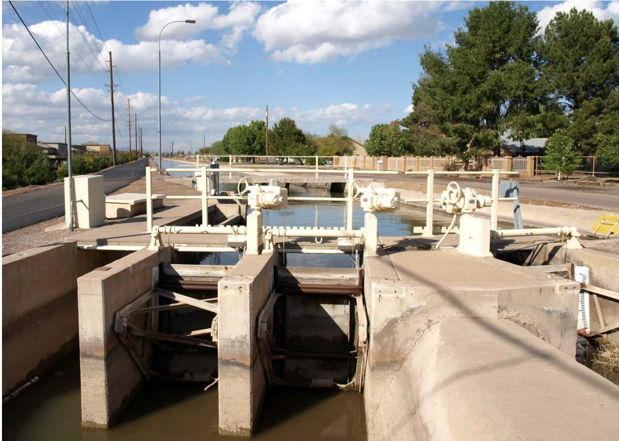
Photo 45. Eastern Canal toe at Pecos Road looking north.
