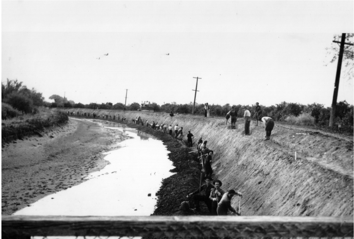
Historic Photo 5. Italian prisoners of war working on the Arizona Canal, December 1943. Photo courtesy of the SRP.
