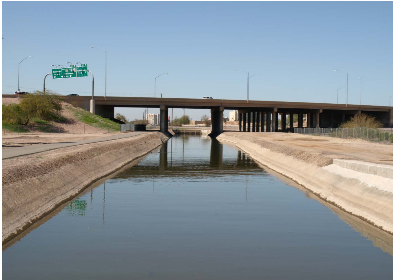
Photo 24. Grand Canal at Hohokam Expressway looking west.
