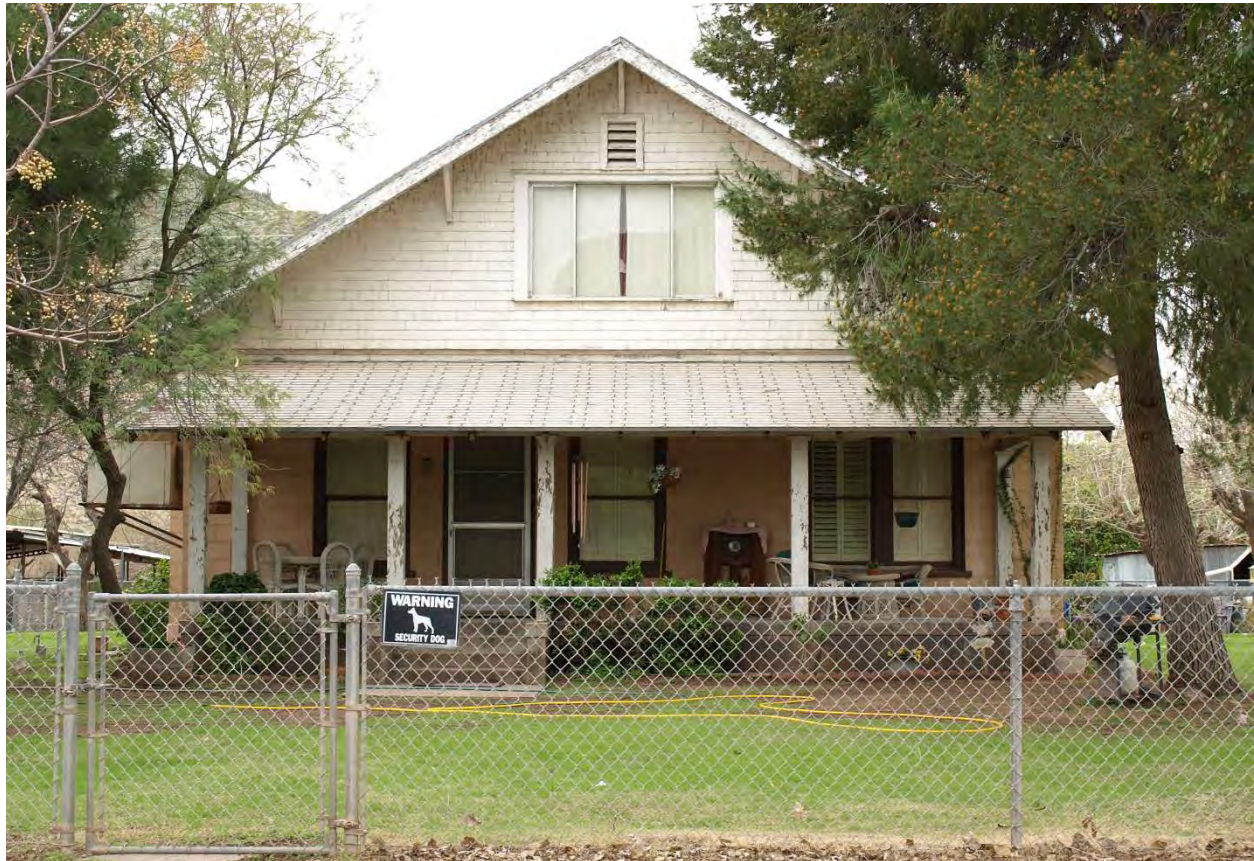
Photo 8. Granite Reef Diversion Dam dam tenders house looking south.
