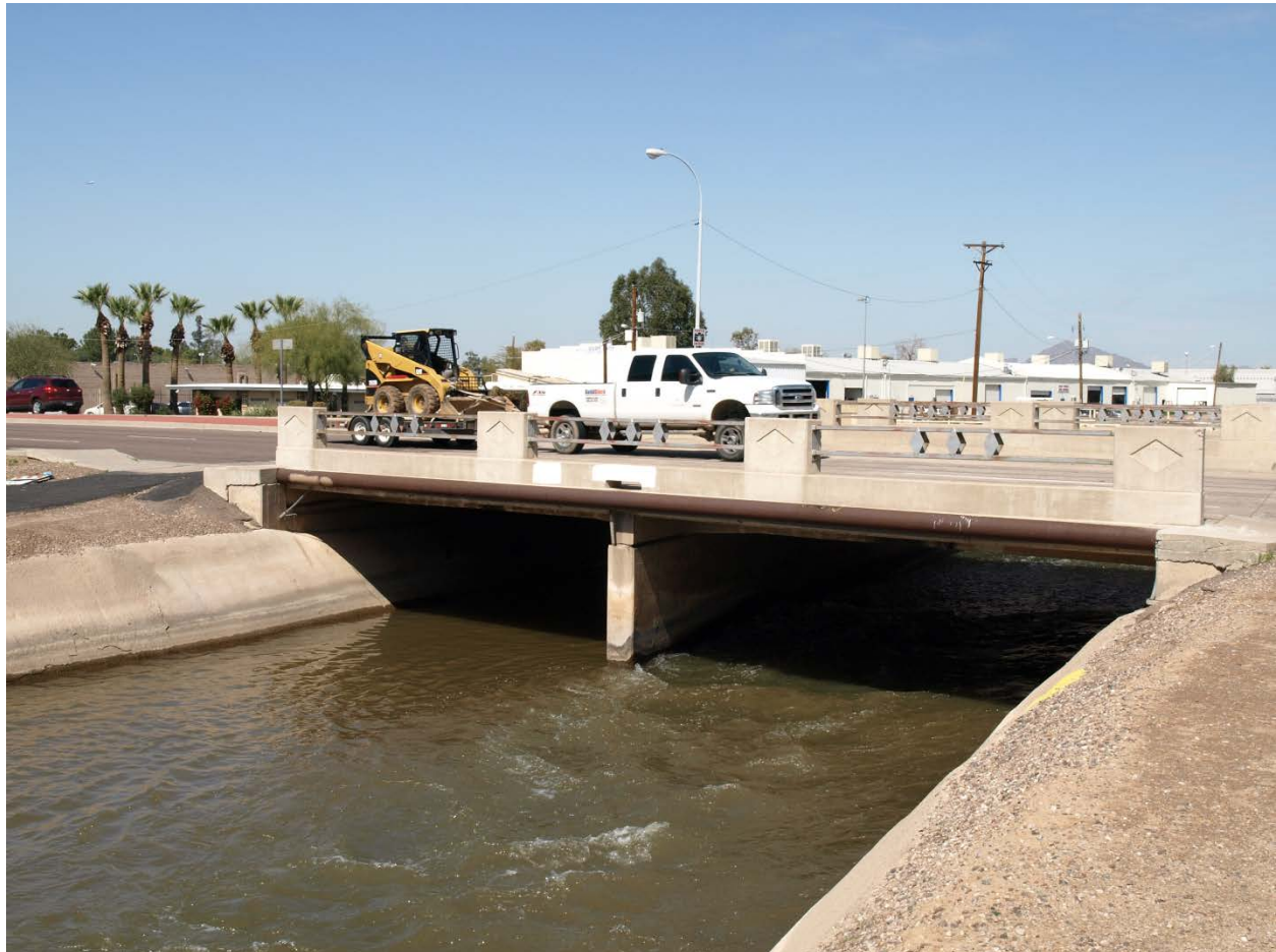
Photo 48. Tempe Canal at Broadway Road looking northwest.
