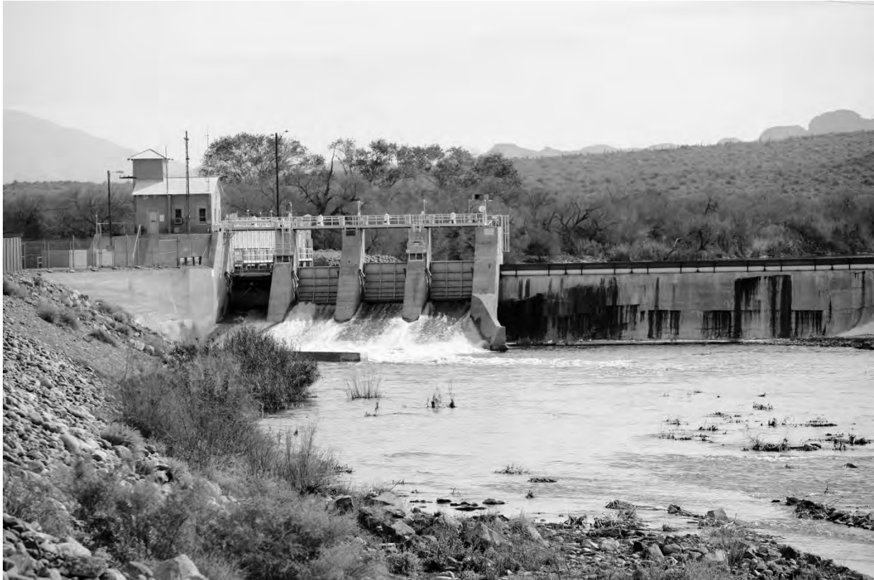
Photo 4. Granite Reef Diversion Dam north side turnout structures looking east. Photo courtesy of the SRP.
