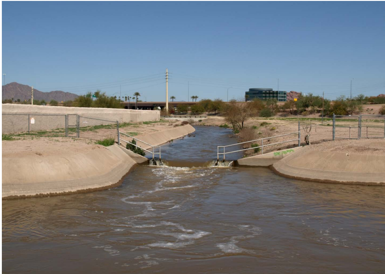
Photo 23. Grand Canal (foreground) at Old Crosscut Canal toe looking north.
