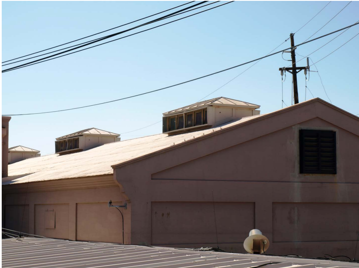
Photo 22. Crosscut Hydro Plant roof detail.
