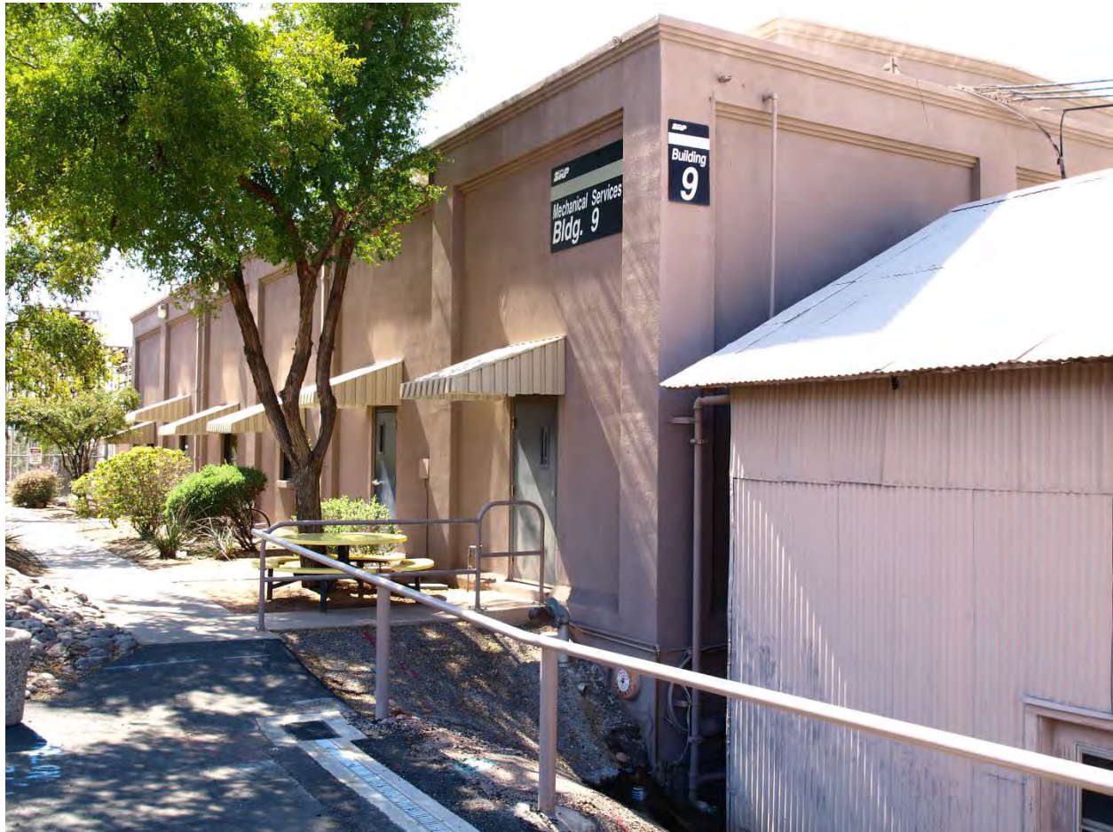
Photo 21. Crosscut Hydro Plant looking southwest.
