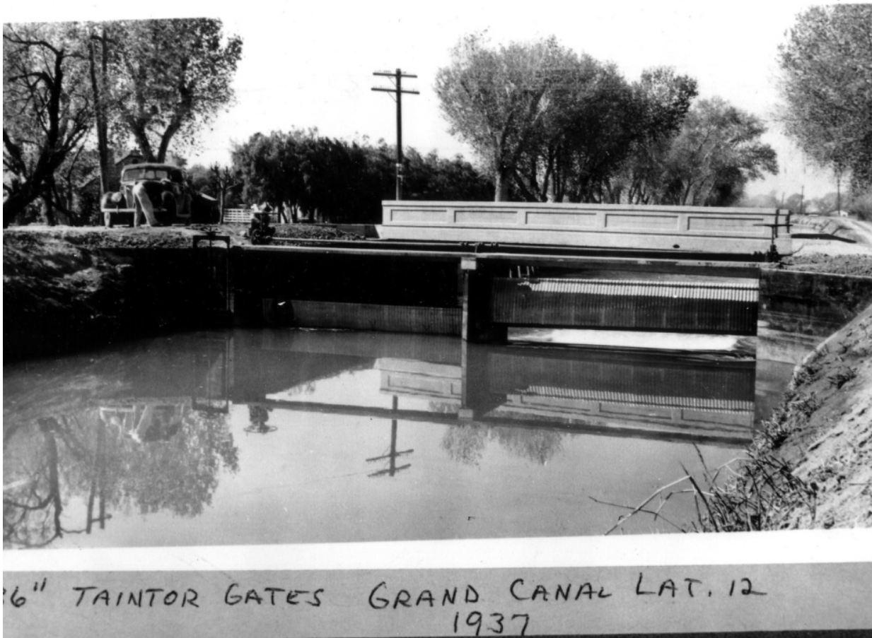
Historic Photo 9. Taintor gates on the Grand Canal at 7 th Avenue, 1937. Photo courtesy of the SRP.
