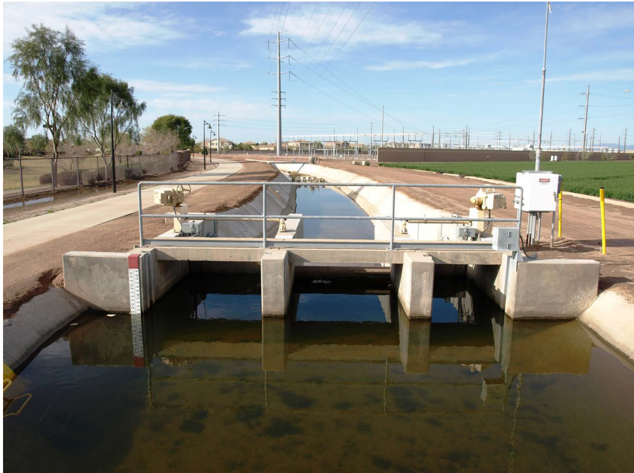
Photo 39. Consolidated Canal check at Ocotillo Road looking north.
