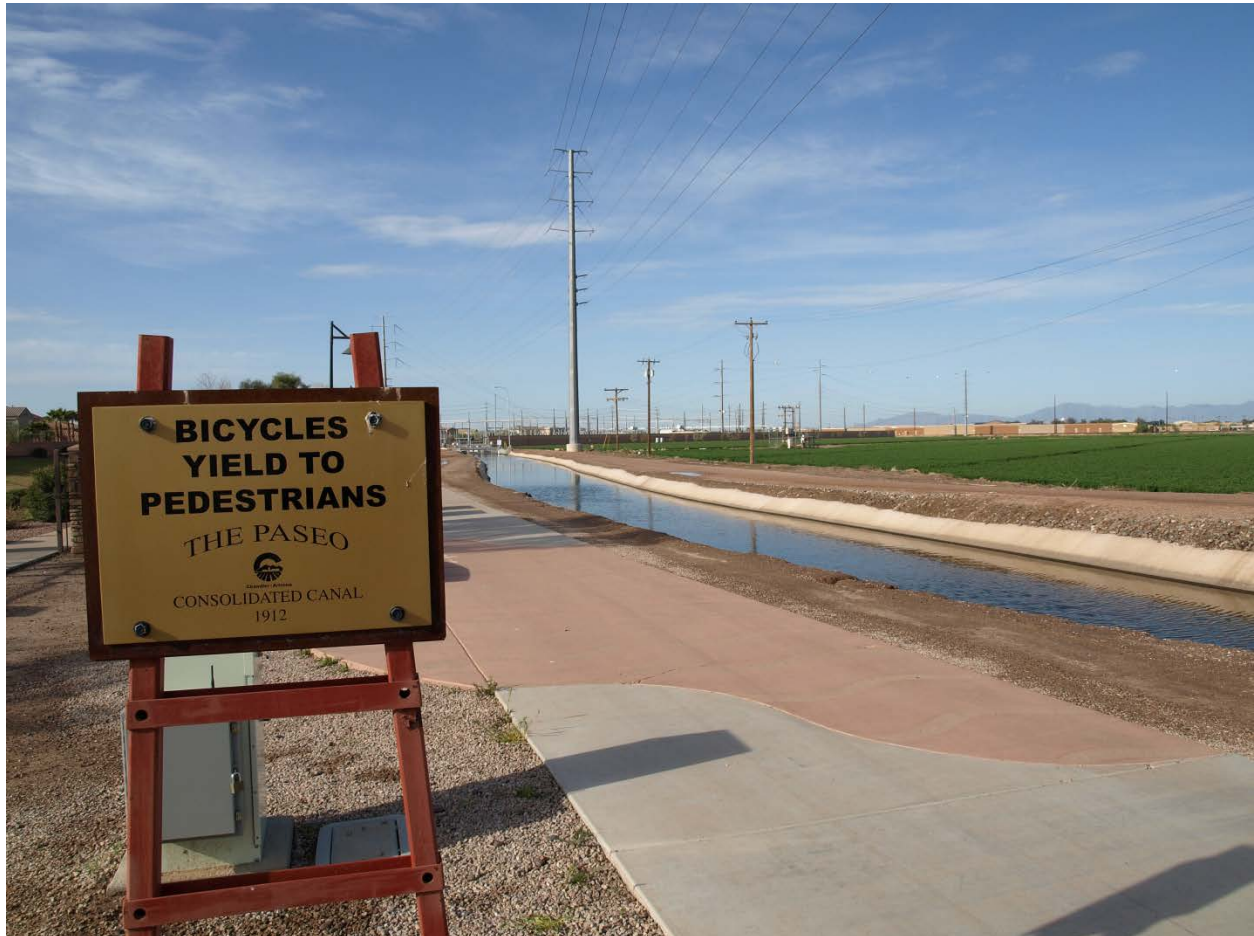
Photo 38. Consolidated Canal at Ocotillo Road looking south.
