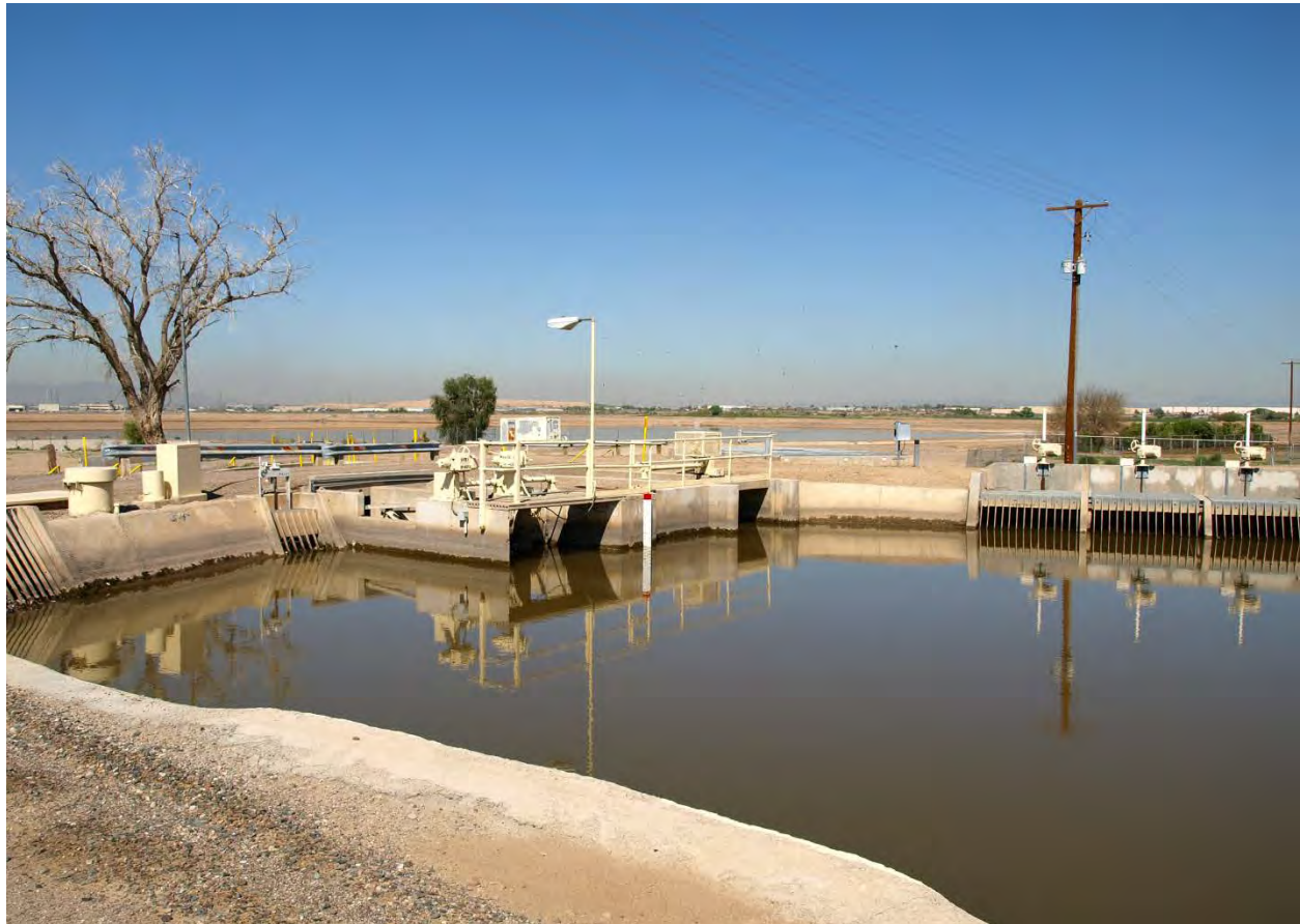
Photo 29. Grand Canal toe drain looking northwest.
