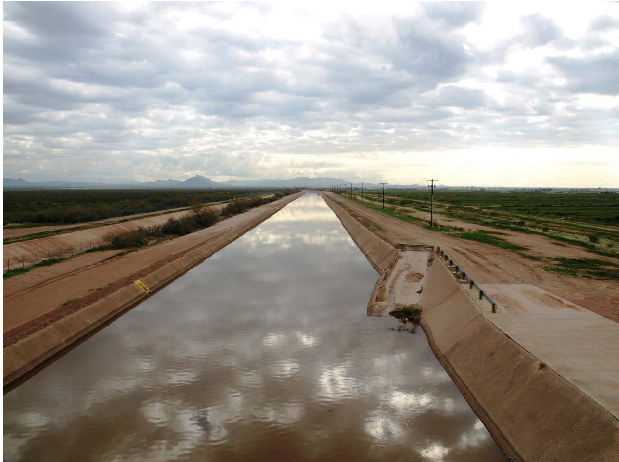
Photo 9. Arizona Canal at Arizona State Route (Loop) 101 looking east.
