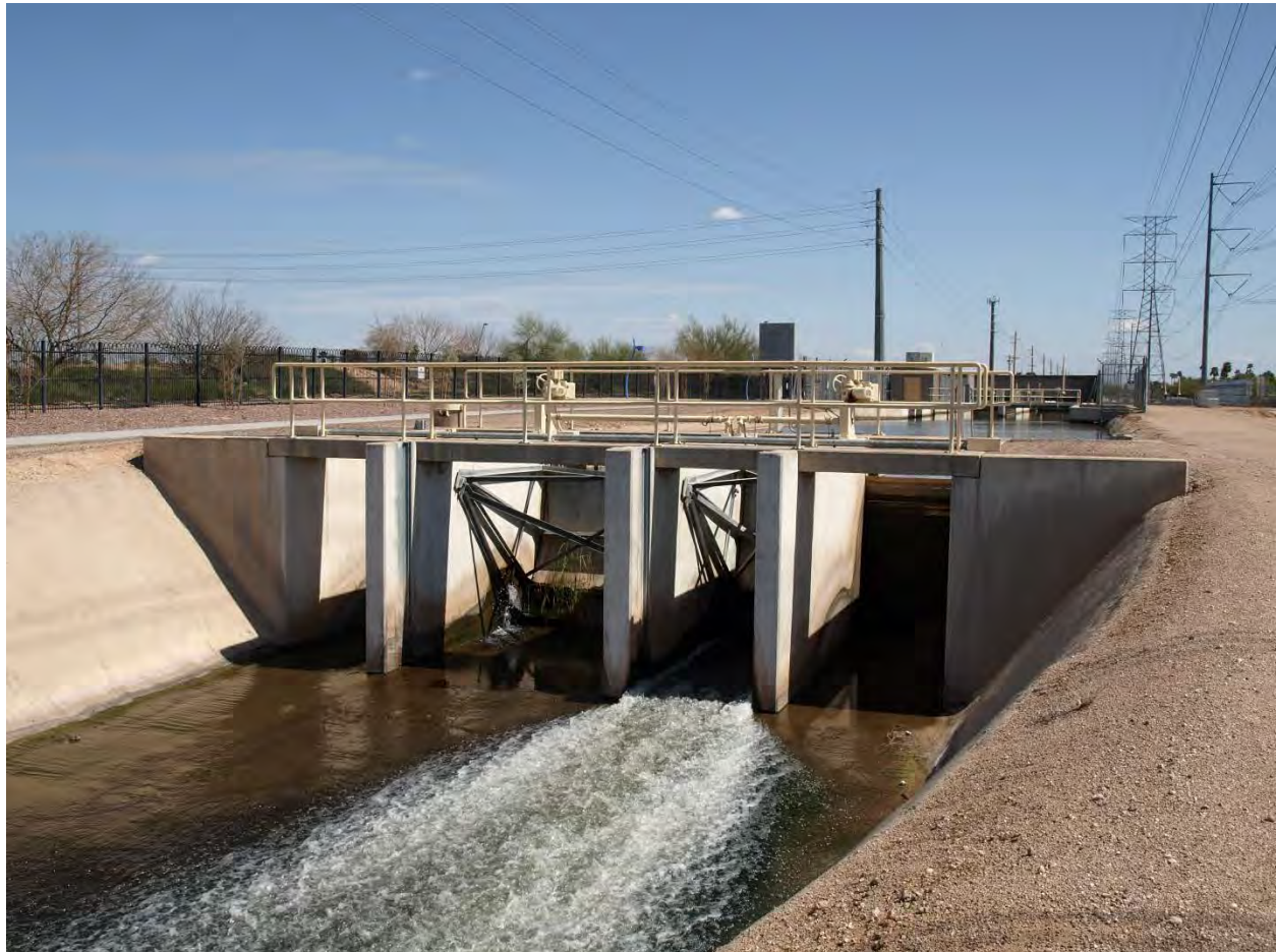
Photo 51. Western Canal at Tempe water treatment plant looking east.
