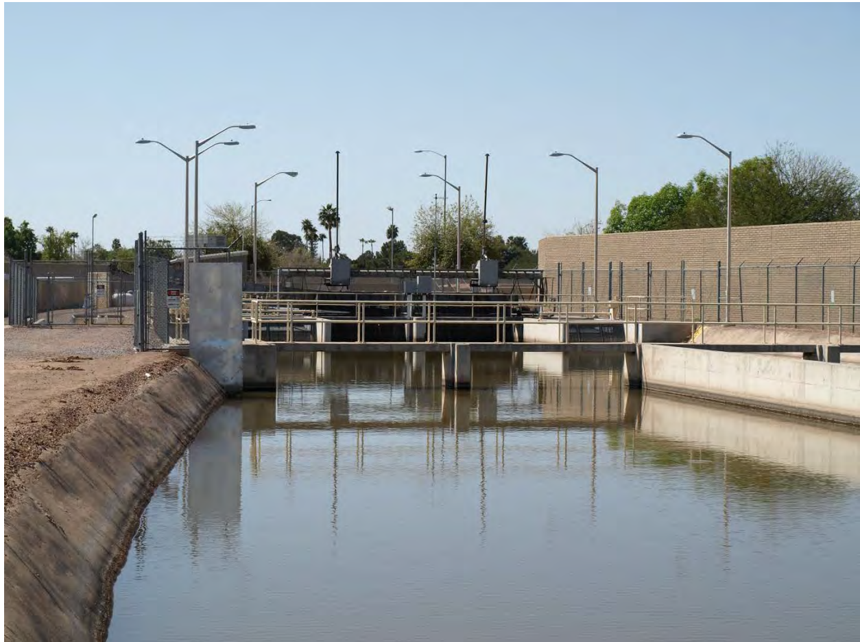
Photo 50. Tempe Canal piped section intake looking south.
