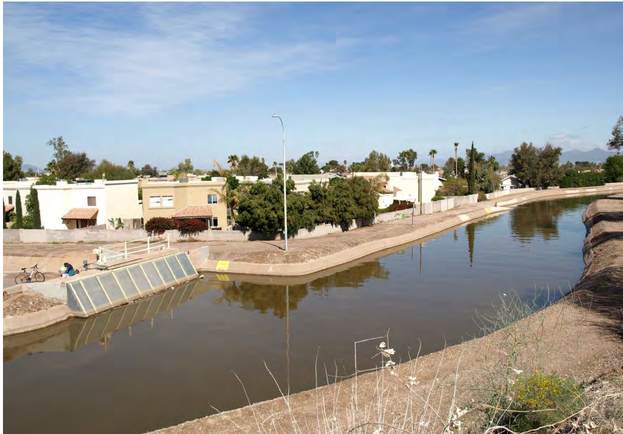
Photo 46. Tempe Canal at Tempe Draw gates looking northwest.
