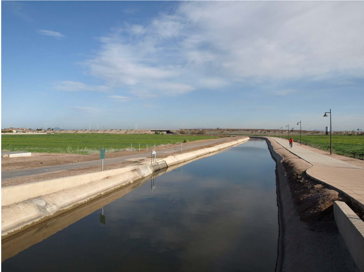
Photo 37. Consolidated Canal at Arizona State Route (Loop) 202 looking north.
