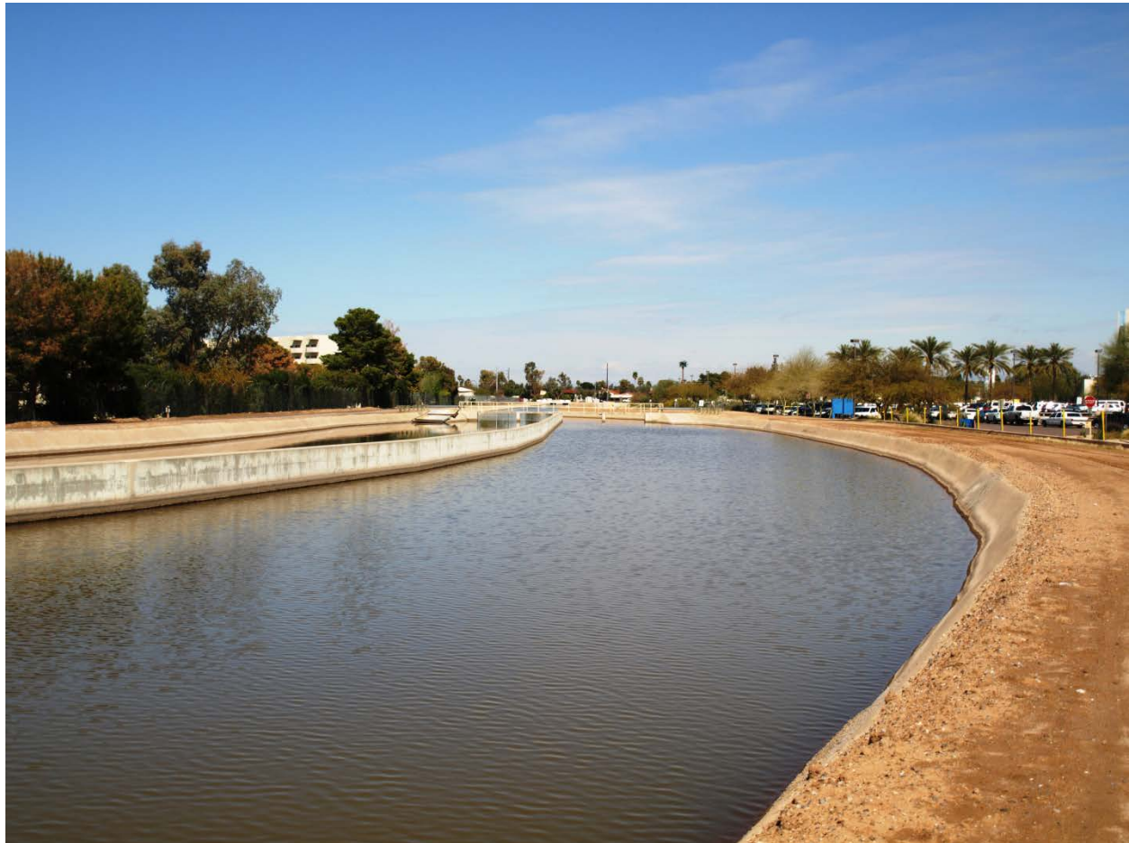
Photo 49. Tempe Canal just north of piped section looking north.
