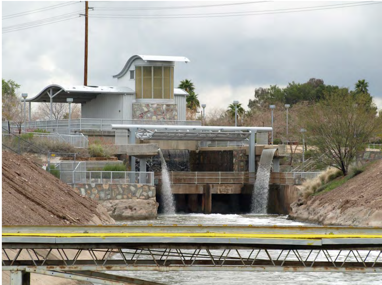
Photo 11. Arizona Canal at Old Arizona Falls power plant looking east.
