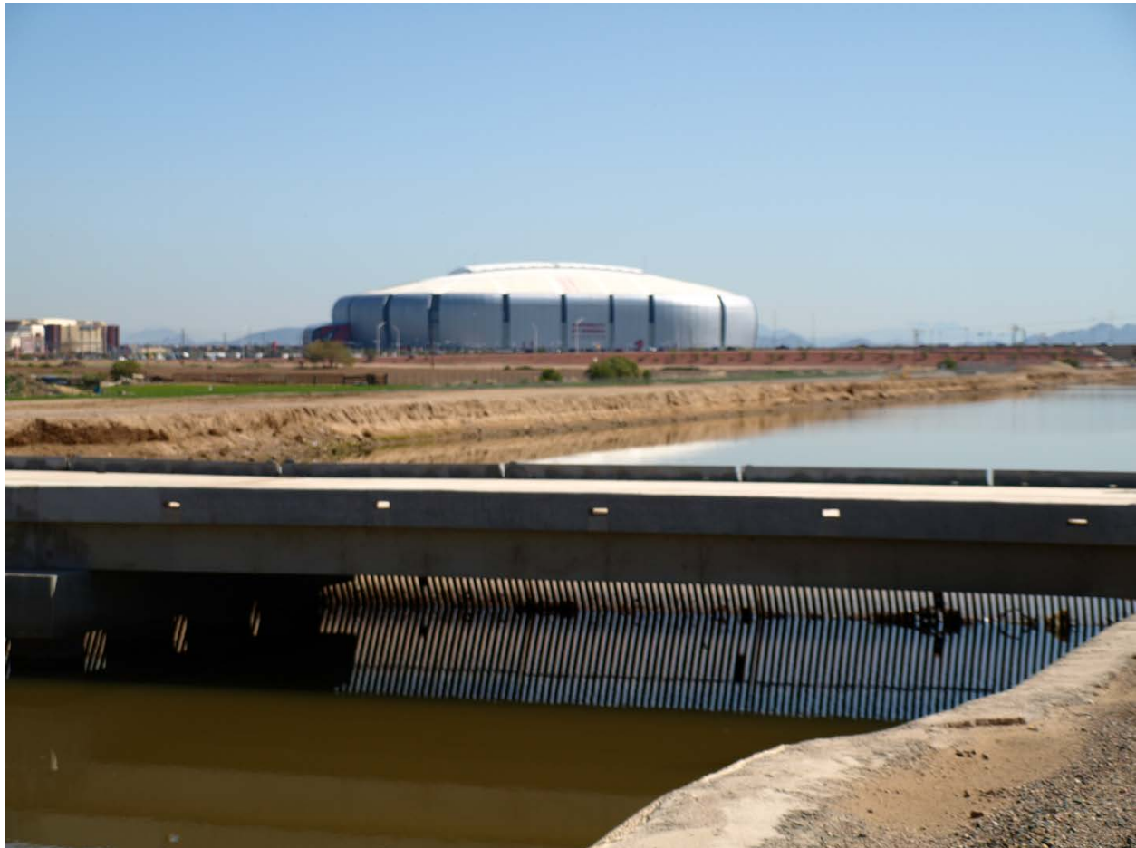
Photo 28. Grand Canal west of University of Phoenix (Cardinals) Stadium looking northeast.
