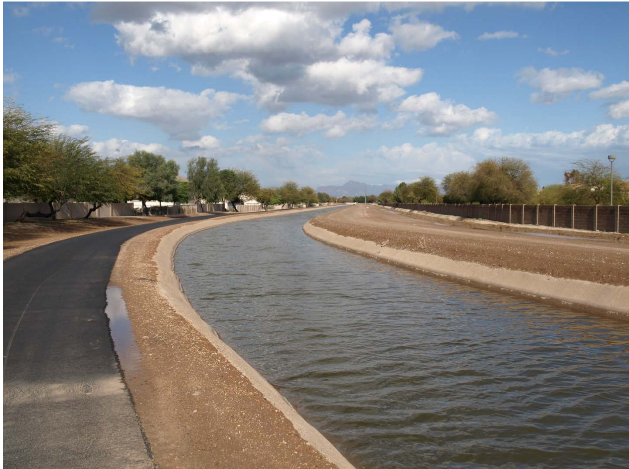
Photo 44. Eastern Canal at Williams Field Road looking north.
