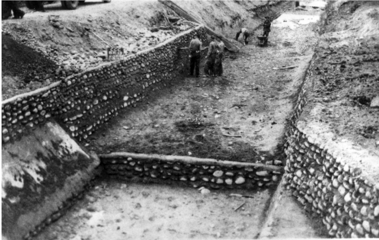
Rubble paving job in Grand Canal at 4E - 10N - January 18, 1938
