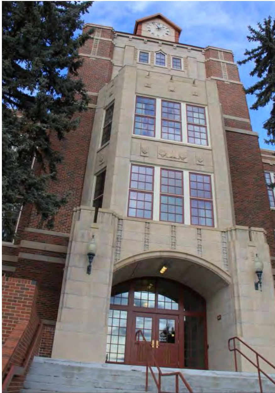
0009 Photo of the tower and front entry area. View to north.
