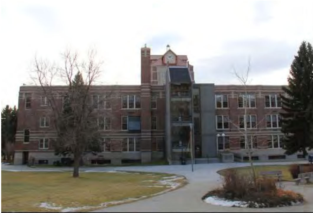
0004 Photo of the north side of McMullen Hall. View to south.
