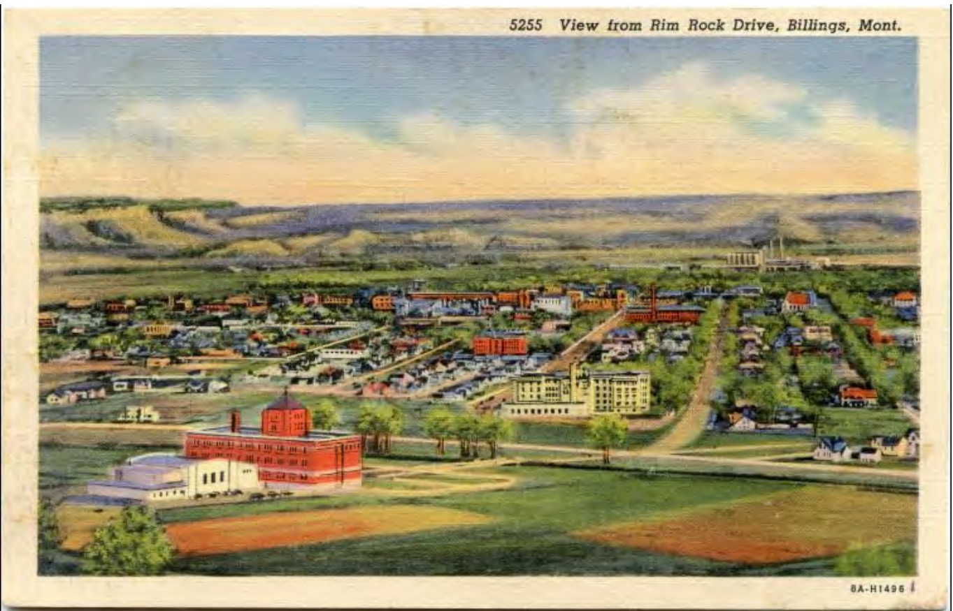
Post card of Billings of the late 1930s looking over the new Administration & Educational with attached gymnasium/auditorium looking from the northwest to the southeast.
