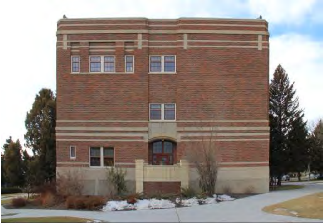
0005 Photo of the east side of McMullen Hall. View to west.
