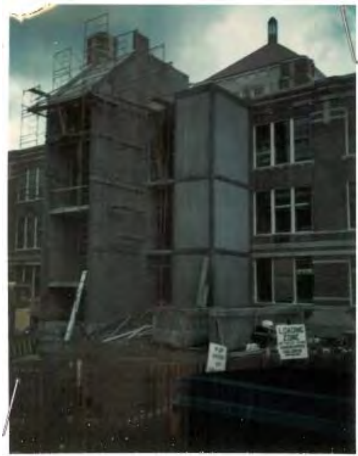
Photo looking from the northwest to the southeast of the construction of the elevator and stair tower at the back of McMullen Hall in 1971.
