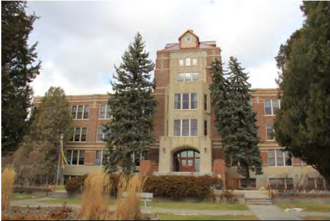
0002 Photo of the front (south elevation) of McMullen Hall. View to north.
