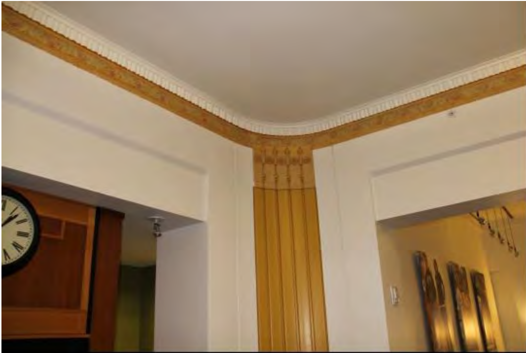
0013 Detail photo in the interior of the main entry. The ornate coving is of original construction.
