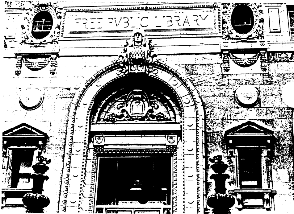
Detail, Main entry
