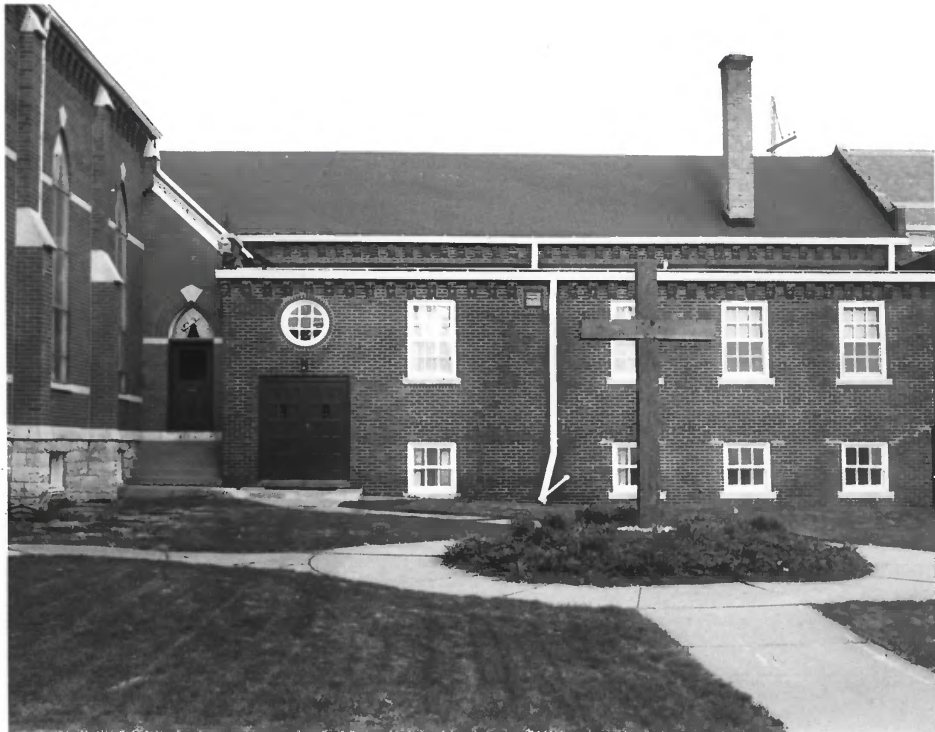
#1 PARISH HALL FRONTING WASHINGTON STREET, VALPARAISO
