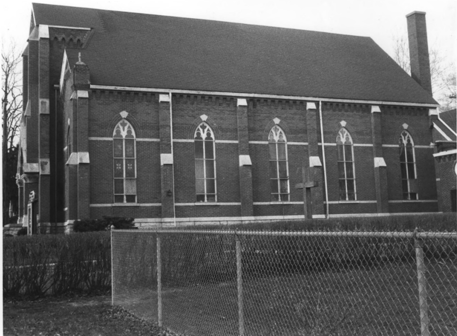
#2 - SOUTH SIDE CHURCH BLDG ATTACHED TO PARISH HALL AT RIGHT (See #1)
