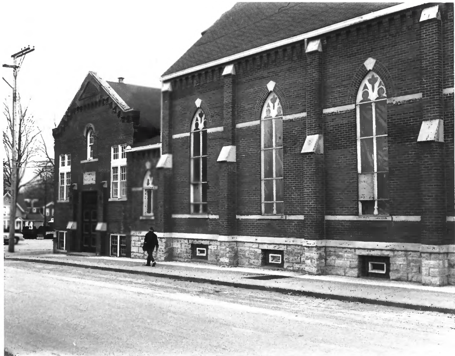
#5 Entrance Parish Hall faces north
