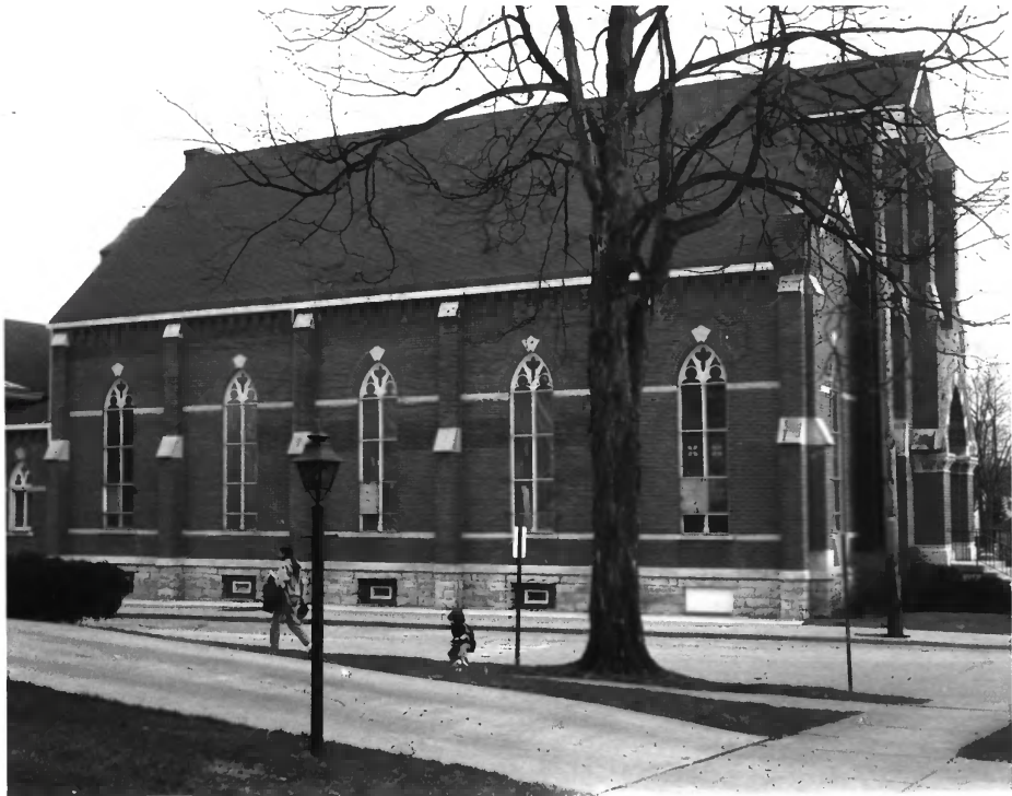
#4 SIDE OF CHURCH ALONG INSTITUTE STREET (North Side Bldg)
