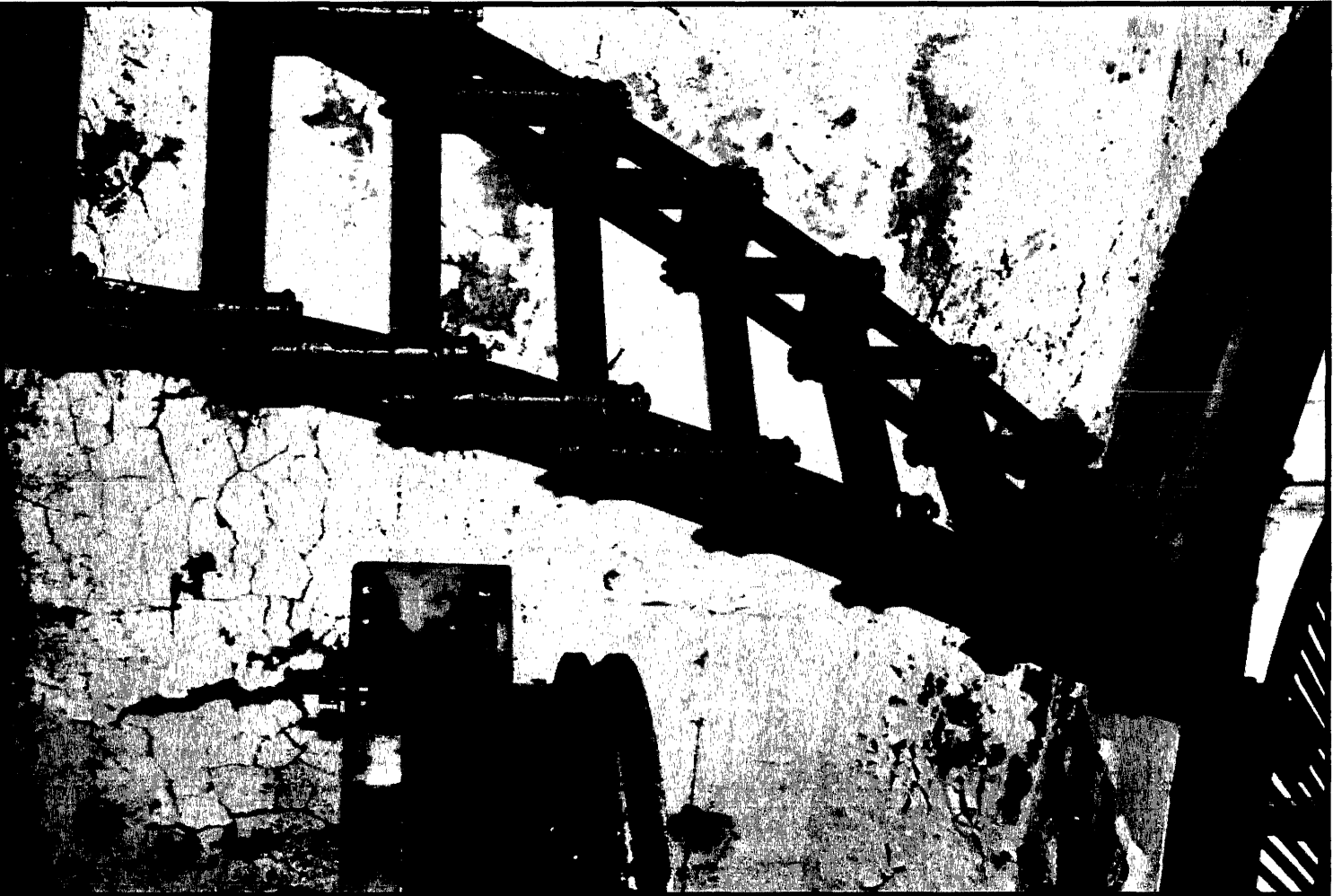
Lantern House Stairs
