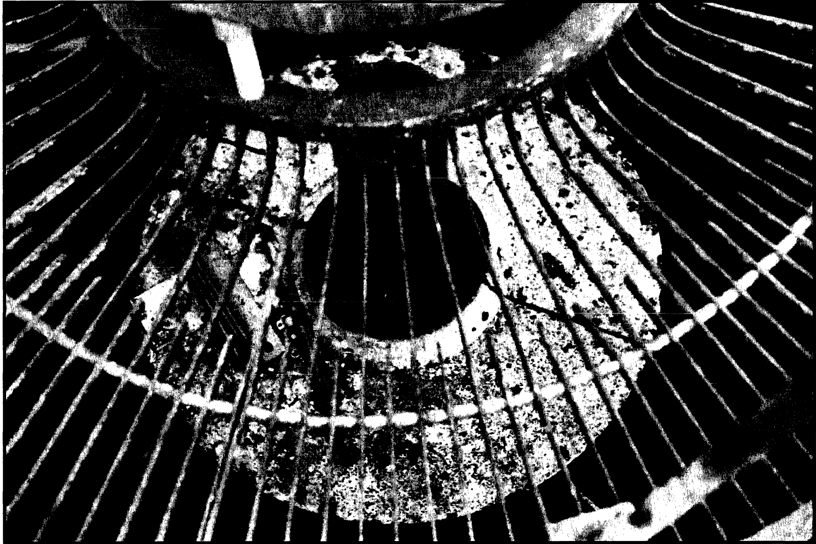
Grate between Lamp and Rotating Machinery
