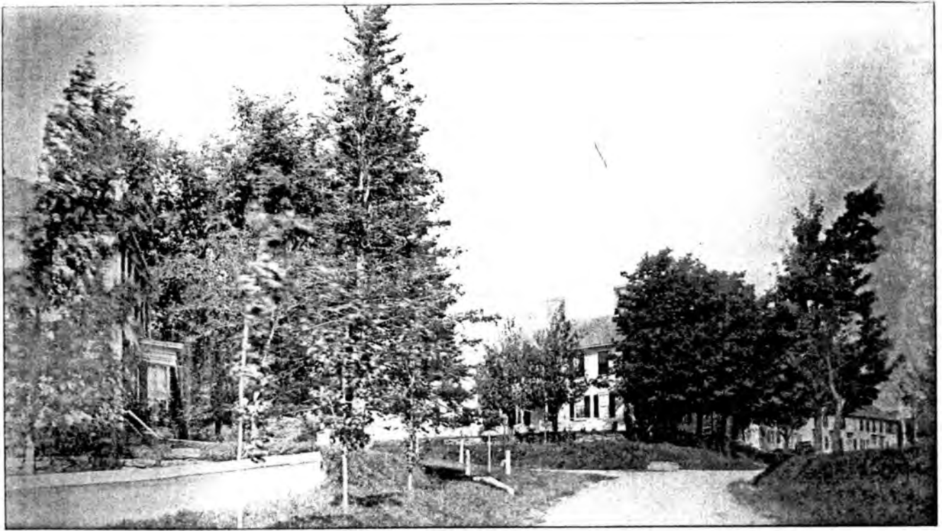
C. View east, with 52, 48, 46 and 44 Hubbardston Road, c. 1900.
