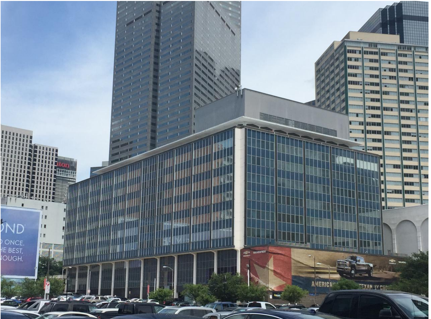
Figure 21. Mayflower Building, Dallas, Texas, 1964–1965. Source: Dallas Morning News .
