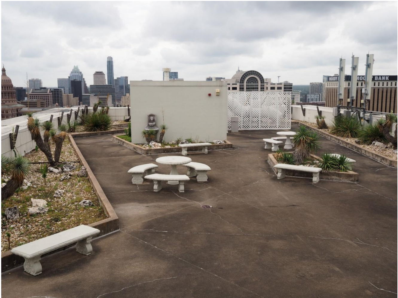
Photo 11. Current photograph (facing south) of the roof garden.
