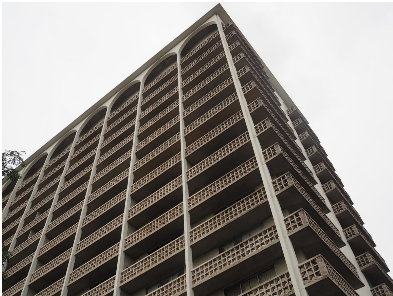
Photo 4. Current photograph of the northeast corner of the building.
