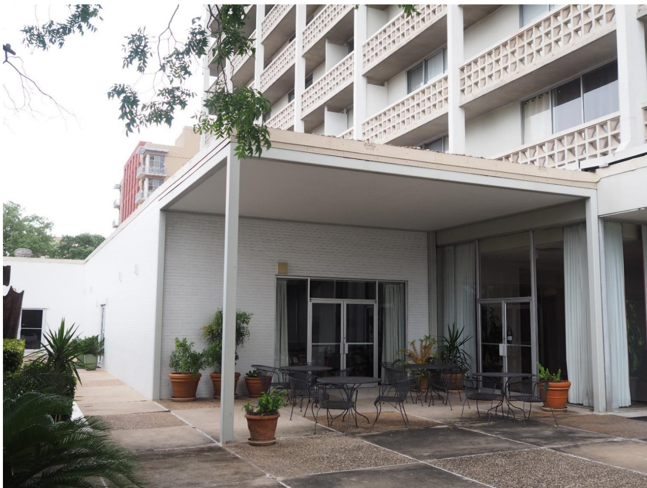
Photo 8. Current photograph (facing south) of the covered patio at the rear of the building.
