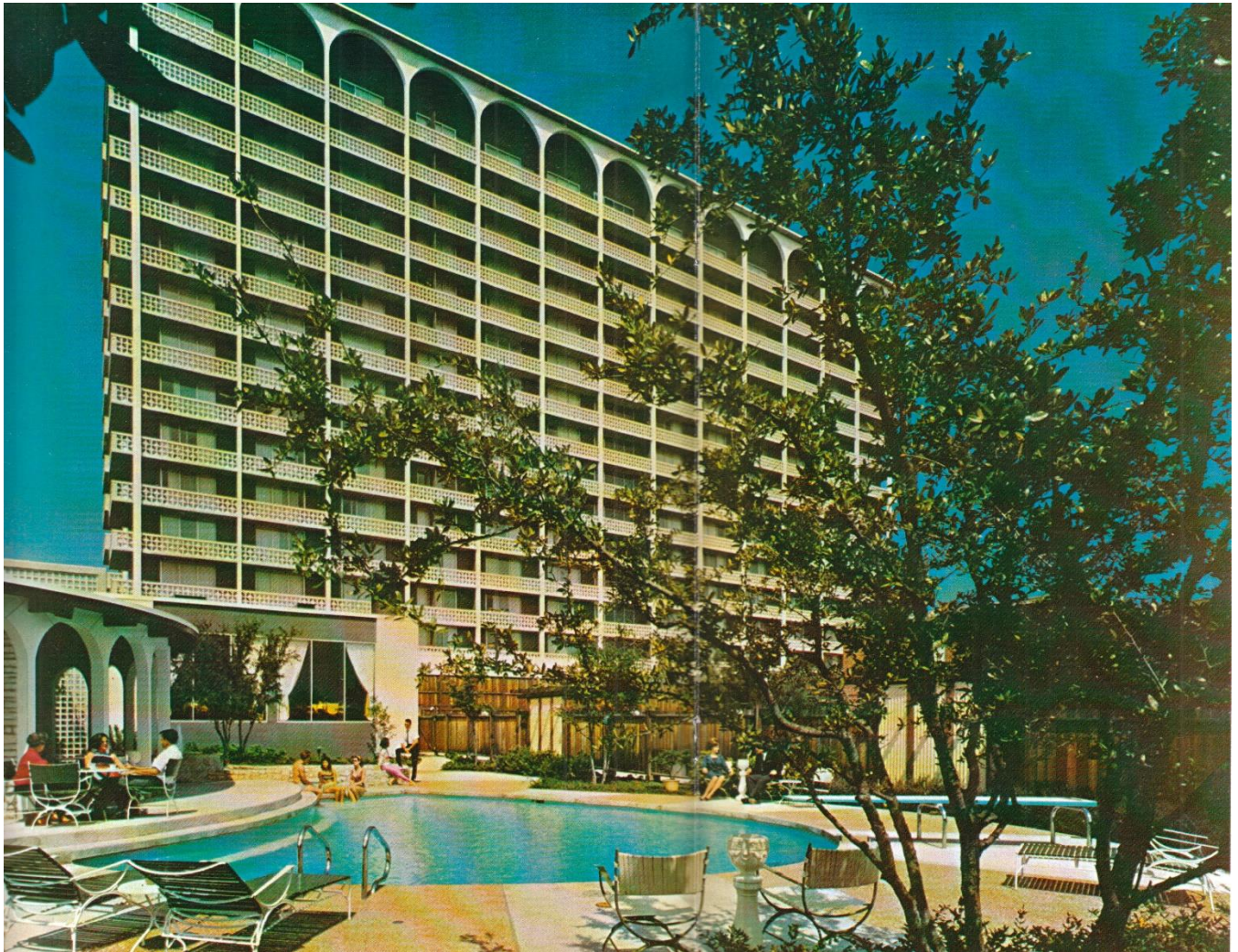
Figure 4. Photograph of east elevation and pool area of Cambridge Tower, ca. 1975. Source: Cambridge Tower.
