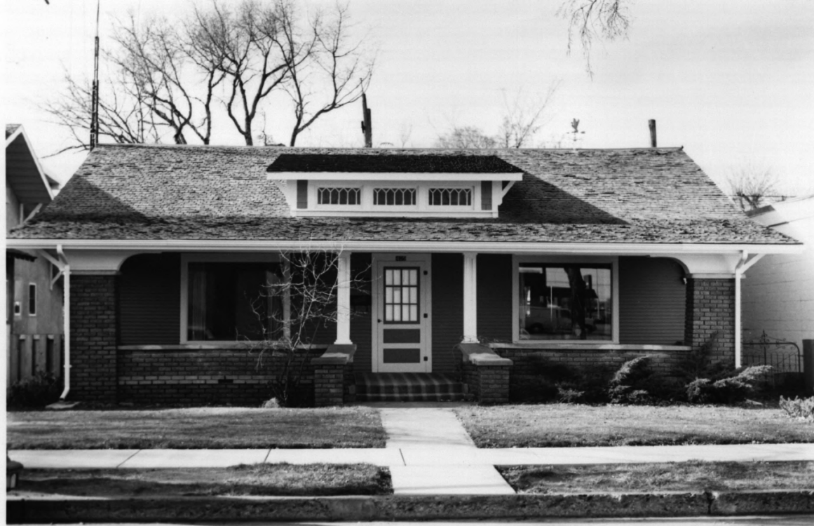
Brown-Evans House, Walworth County, S.D., No. 1
