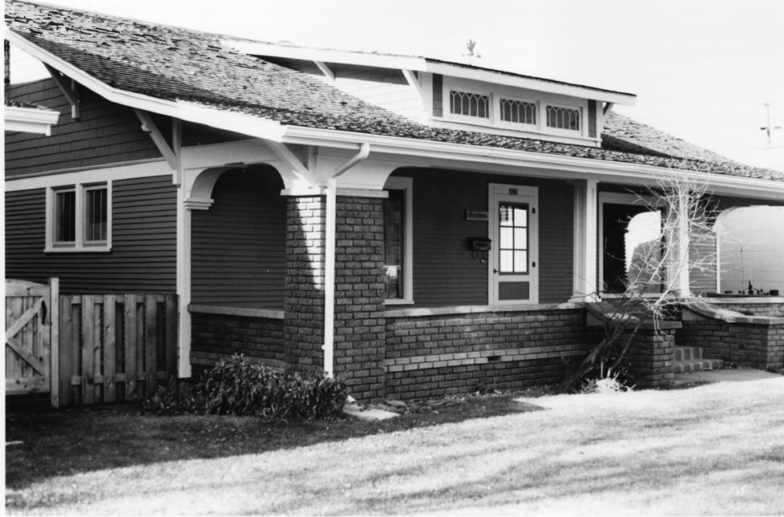
Brown-Evans House, Walworth County, S.D., No. 2
