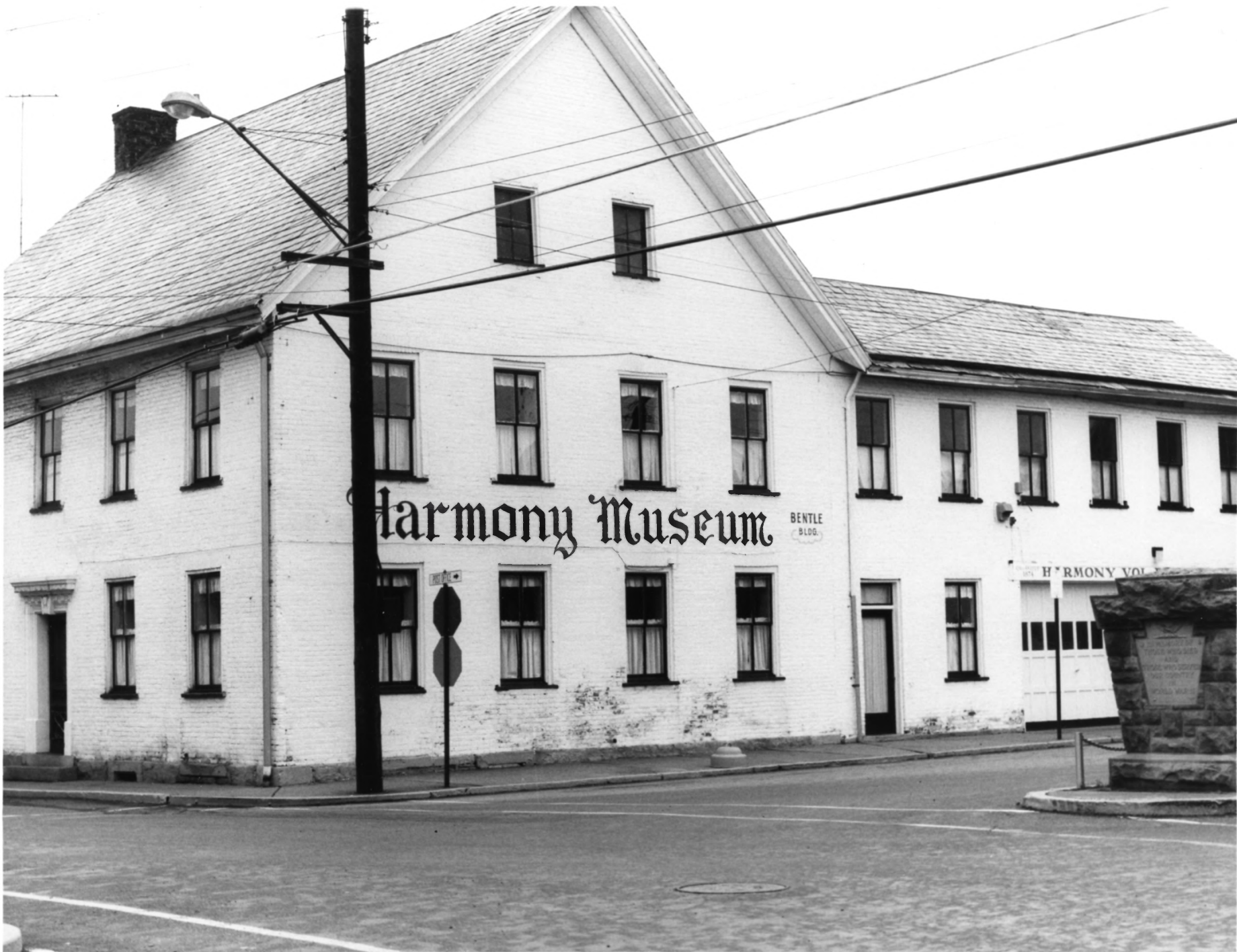
Great House, or Bentle Building, Harmony, Pennsylvania
