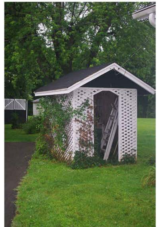
Photo 15: Well house looking southwest.
