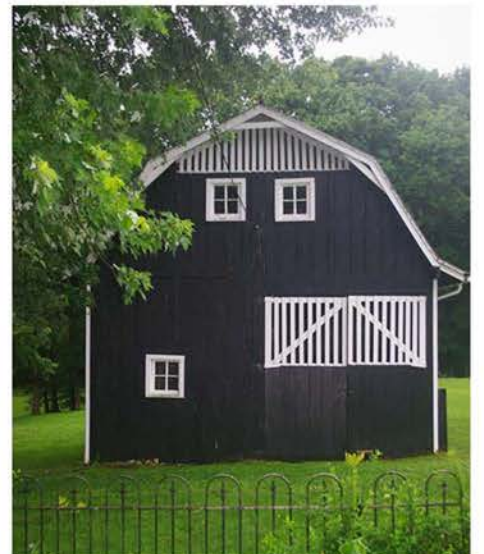
Photo 12: Right – barn, north face.
