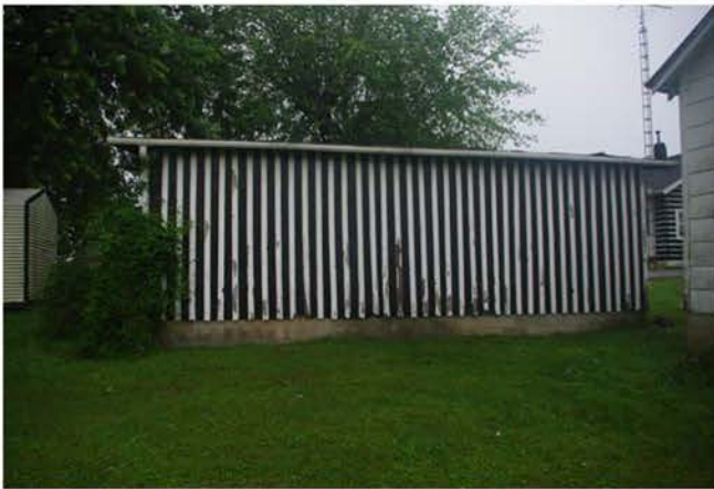
Photo 8: East face of garage.
