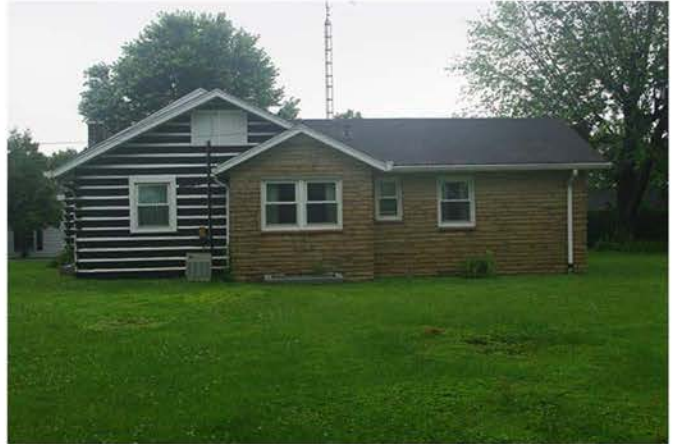
Photo 5: 1952-53 addition, west face.
