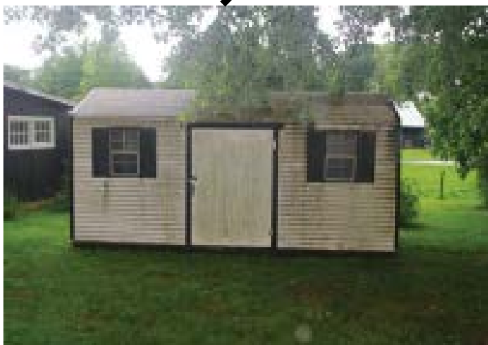
White Metal Shed, west face
