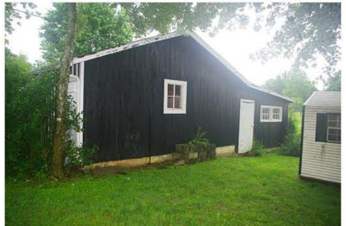
Photo 11: Garage, south face.
