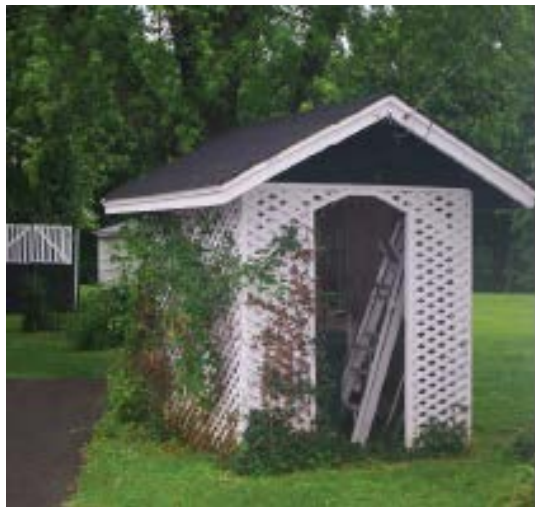
Well House, looking southwest
