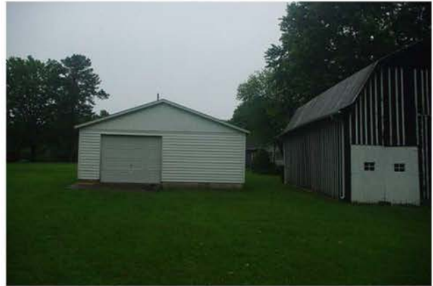
Photo 17: White vinyl storage building, south face.
