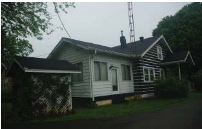
Main Dwelling, enclosed screen porch
