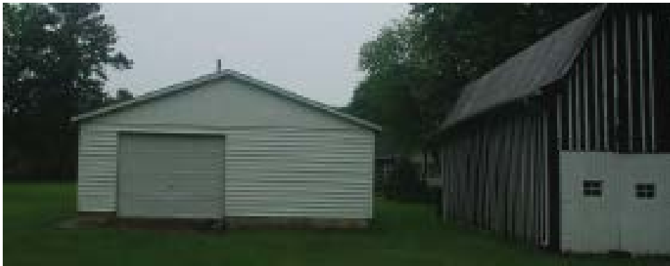
White Metal Storage Building, south face
