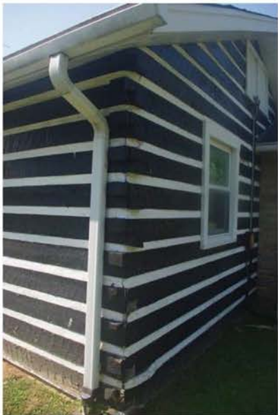
Photo 19: Northwest corner of faux-log addition.
