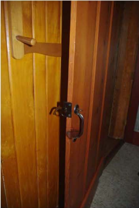
Photo 9: Door latch mechanism on original interior doors.
