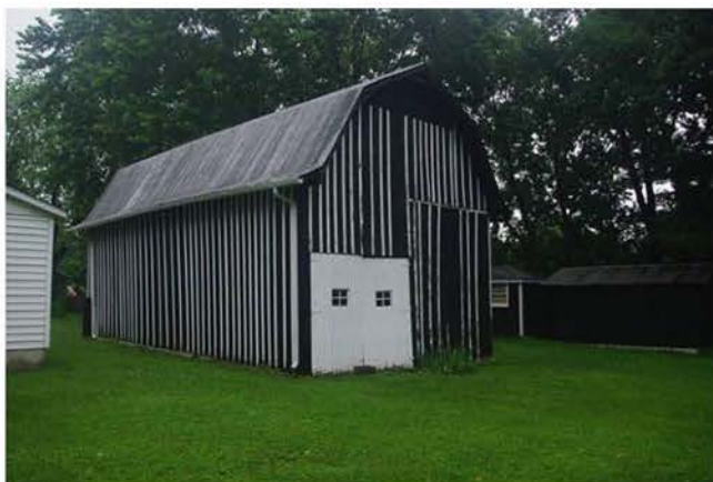
Photo 7: Left – barn, west and south faces.
