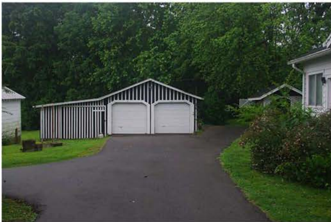
Photo 2: Garage, north face.
