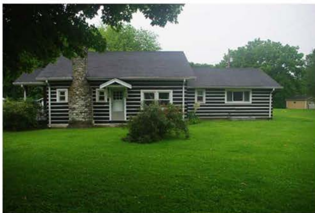
Photo 1: View of Halcomb house from Franklin Road.
