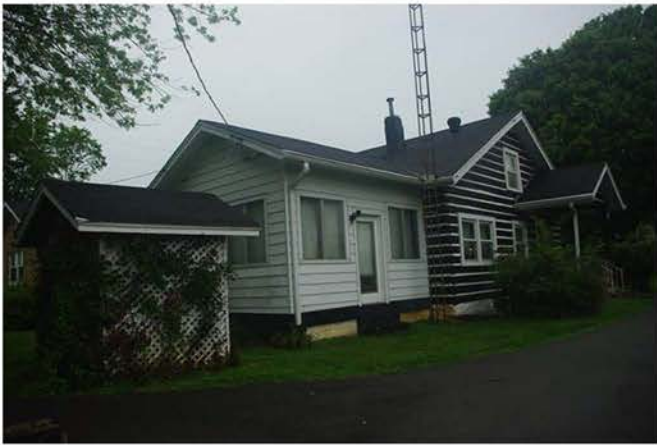
Photo 6: East face of screened porch/office.
