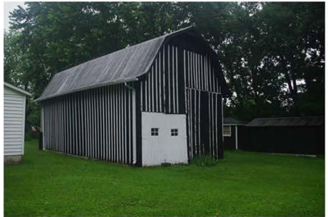
Photo 7: South and west face of barn.
