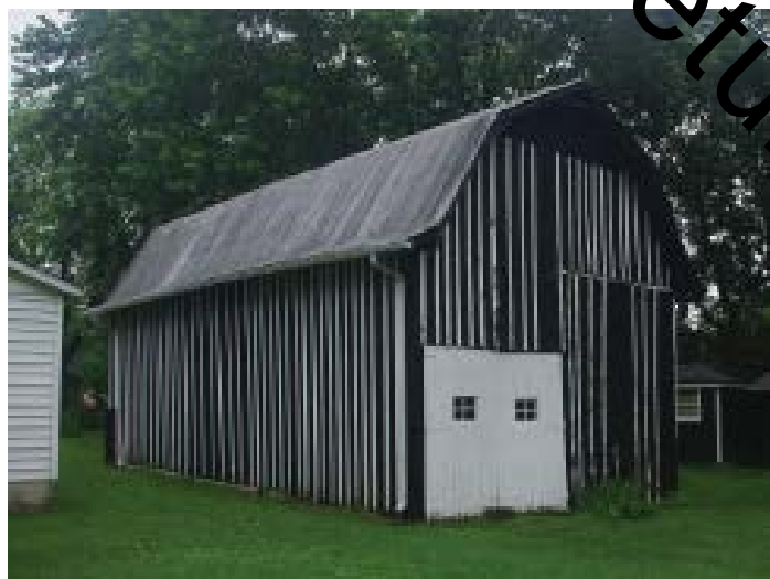
Garage, West and South faces
