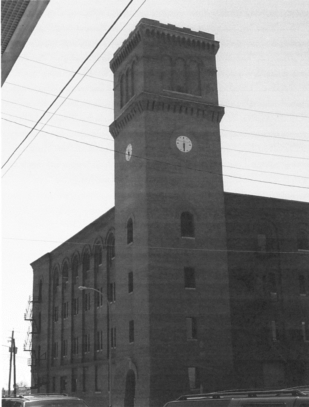
Figure 4 A number of notable building features are seen in this view, including the tower's battered base, the roofline's outward slope (best seen in the upper left corner), and the recessed, round-arched window bays. The masterful work of the building's brick masons is showcased at the top of the tower, above the clock faces, with corbels, blind arcades, and the crenellations. Author's photograph, April 2005.
