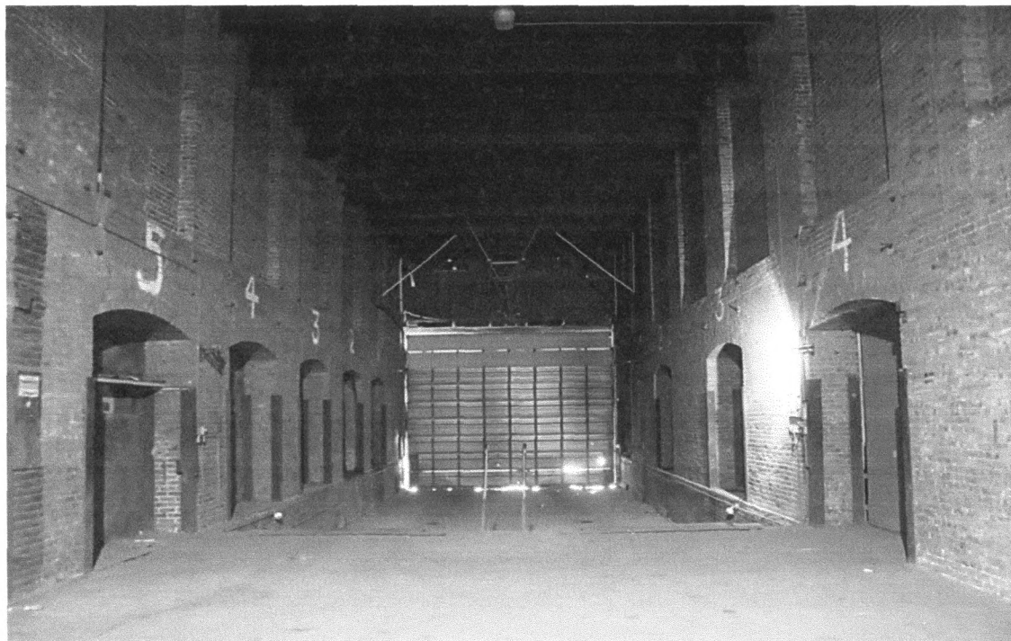
Figure 13 The south railroad portal, now covered by a modern door, is visible in the center of this photograph, with numbered loading bays in the masonry walls on either side of two sets of tracks. The loading doors are elevated to the same height as a rail car. Doors to the left lead into the larger section of the building, toward Water Street and the clock tower. Doors to the right lead to the smaller west part of the building. Not visible but behind the camera is a masonry wall that was a handwritten revision added to the plans. Without it, access between the two sides of the building would have necessitated crossing through this railroad loading bay. Mike Whye photograph, 2007.
