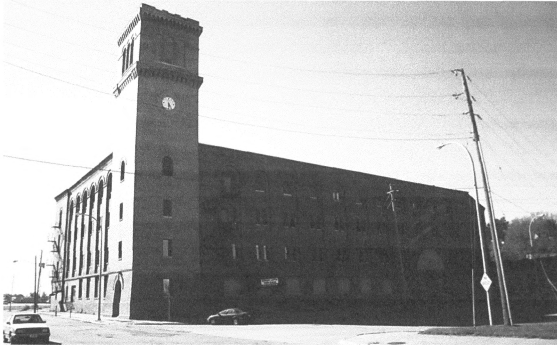
Figure 10 The long north side of the Simmons Hardware Company warehouse is seen here, with the single-story appendage wing at the far right. Mike Whye photograph, 2007.
