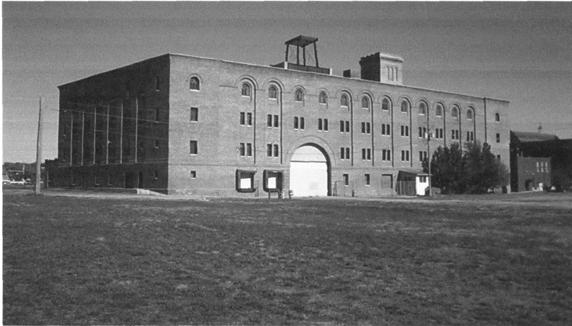
Figure 8 The rail siding portal is a prominent feature of the Simmons warehouse's south elevation seen here, along with the shaded west side. The grassy yard in the foreground once was bisected by the main tracks of the Milwaukee rail line through town. Compare this view to the historic image in Figure 17. Mike Whye photograph, 2007.
