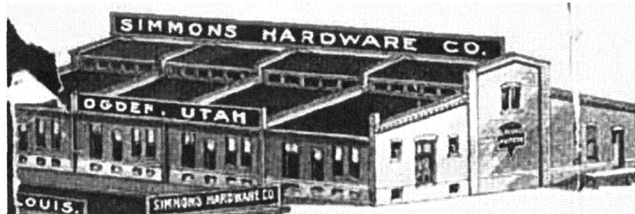
Figure 20 This monitor-roof warehouse in Utah is unusual for its departure from the standard Simmons building appearance. Note the logo on the front of the tall, middle bay. Nothing is known about the building today.
