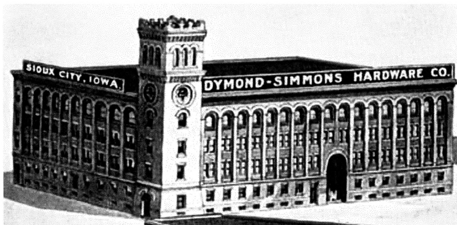
Figure 18 This image of the planned Sioux City warehouse already had a sixth story on the tower, suggesting that the addition of a sixth floor to hold a water tank may not have been a design revision as the local paper suggested. Also, the image shows many more window bays than were actually built and the tower lacks its clock faces. Barely discernible where the clock faces should be is the axe shaped Simmons logo. The 1904 catalog claimed the building would include "150,485 square feet, or 3 1/3 acres" of storage space. Unless otherwise noted, this and the following images are from the Hardware Companies Collectors Klub website ( www.thcck.org on December 7, 2004).
