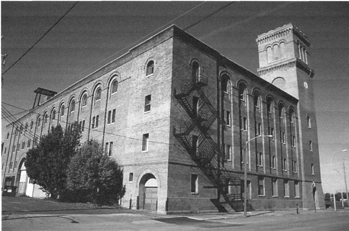
Figure 7 The warehouse's east, Water Street façade (right) and long south side (left) are seen in this current photograph. This image in particular also suggests some historic accommodations that reflect the ever present danger of fire, namely, a tower intended to hold a water tank, the rooftop legs and platform that mark a former water tank location (at left), and, in the center of the image, the zig-zag metal fire escape. Mike Whye photograph, 2007.
