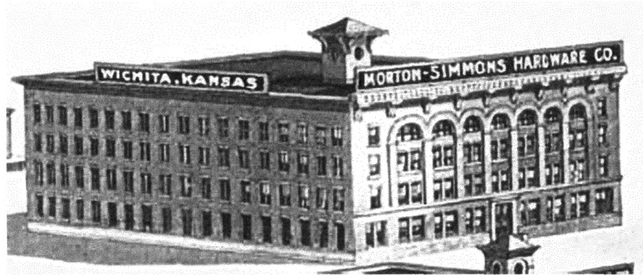
Figure 19 The catalog image of the Wichita warehouse is essentially correct, but the building as constructed has fewer side bays on the left side. After being mothballed and sitting vacant for a number of years, this building was converted to a hotel.
