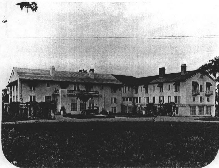
COLONY HOUSE ADDITION — By 1920, Charles R. Wait, an associate of Olmsted's, had been called on to design this addition to the Colony House which was added in 1921.
