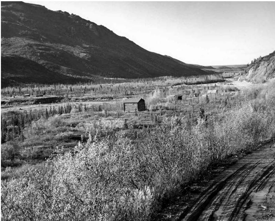
Figure 4 Kantishna roadhouse 1956 (Charles Ott Photo, Denali National Park & Preserve Collection)
