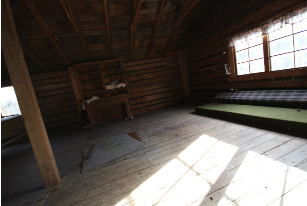
Photo #28 of 37 (AK_Denali Borough_Kantishna Roadhouse_0028) Interior second level, camera facing southwest.
