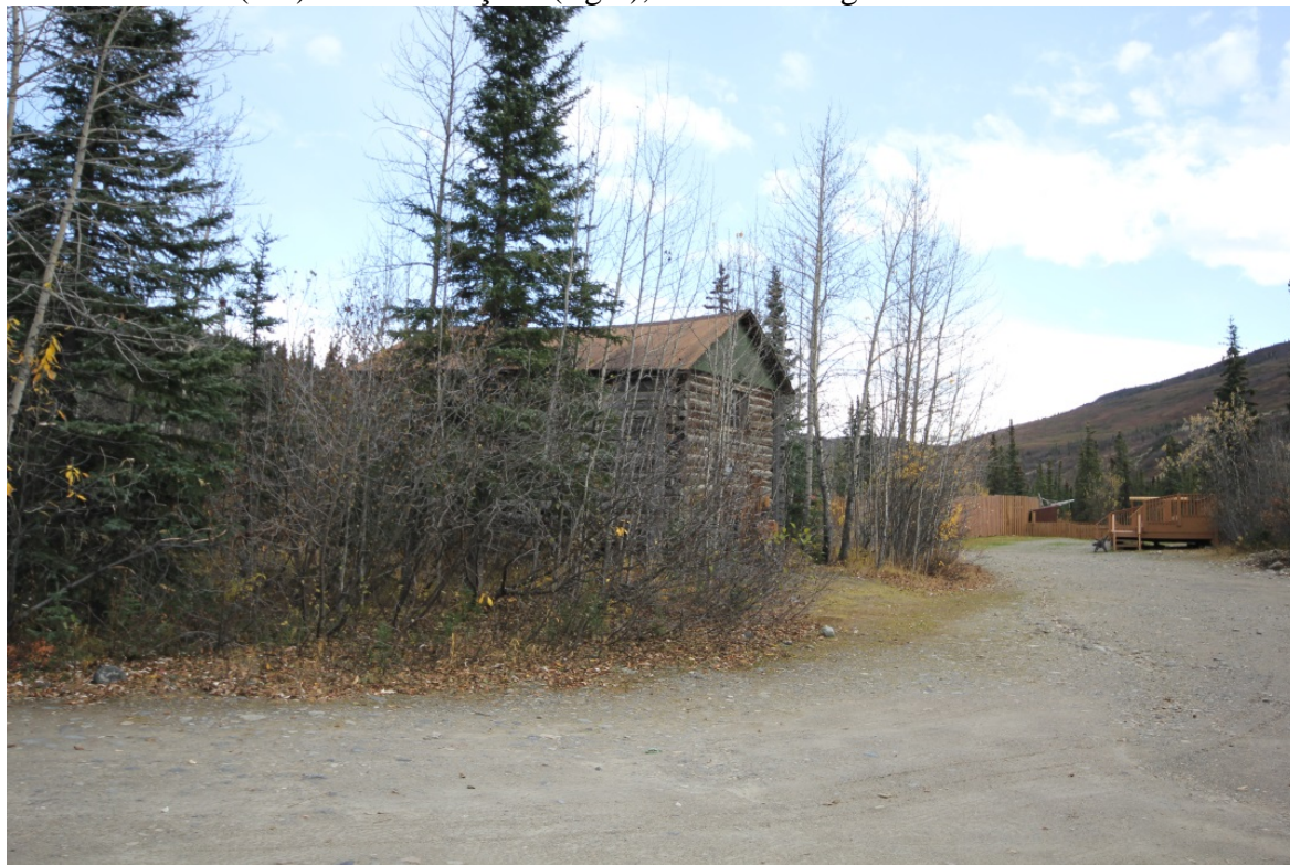
Photo #1 of 37 (AK_Denali Borough_Kantishna Roadhouse_0001) North elevation (left) and west façade (right), camera facing southeast.
