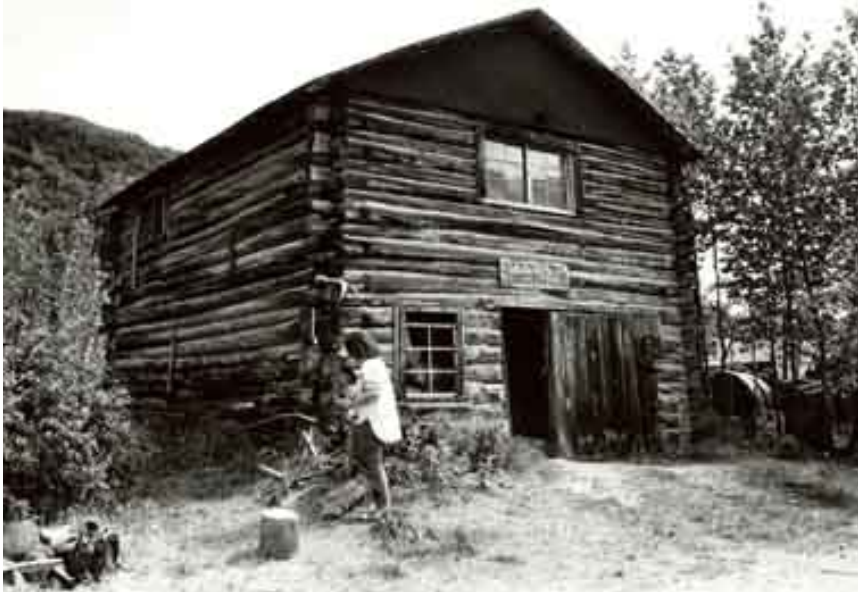
Figure 5. Kantishna Roadhouse in 1988, one year before NPS stabilization (“Kantishna Roadhouse,” Cultural Resources Files, Denali National Park, 1988)
