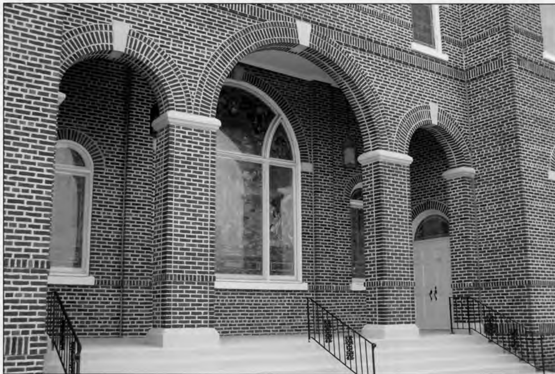
5. Allen Temple A.M.E. Church 109 Green Avenue, Greenville Greenville County, South Carolina
