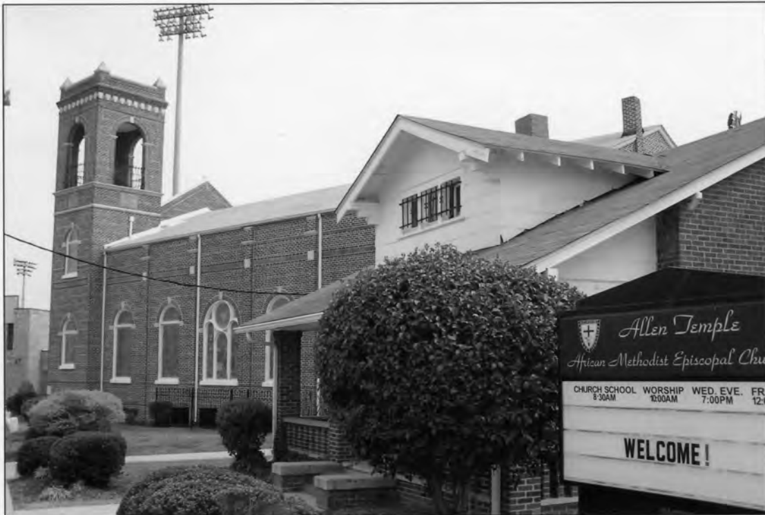
24. Allen Temple A.M.E. Church 109 Green Avenue, Greenville Greenville County, South Carolina
