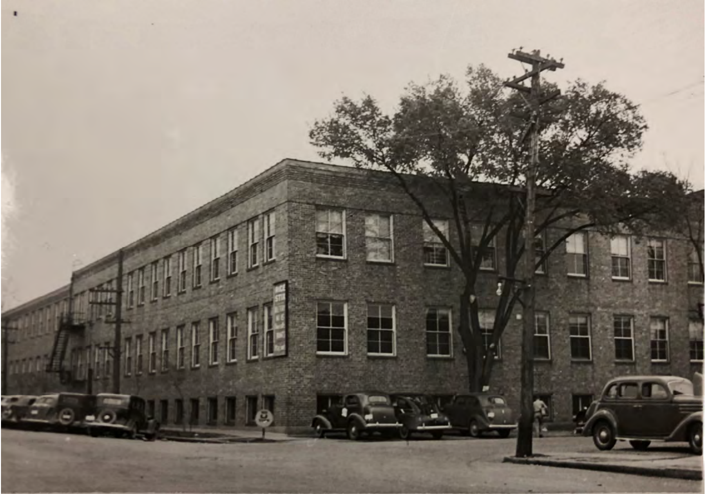
Figure 11. Rice-Stix Building c. 1940. Source: Lebanon Chamber of Commerce Photograph Collection, State Historical Society of Missouri.
