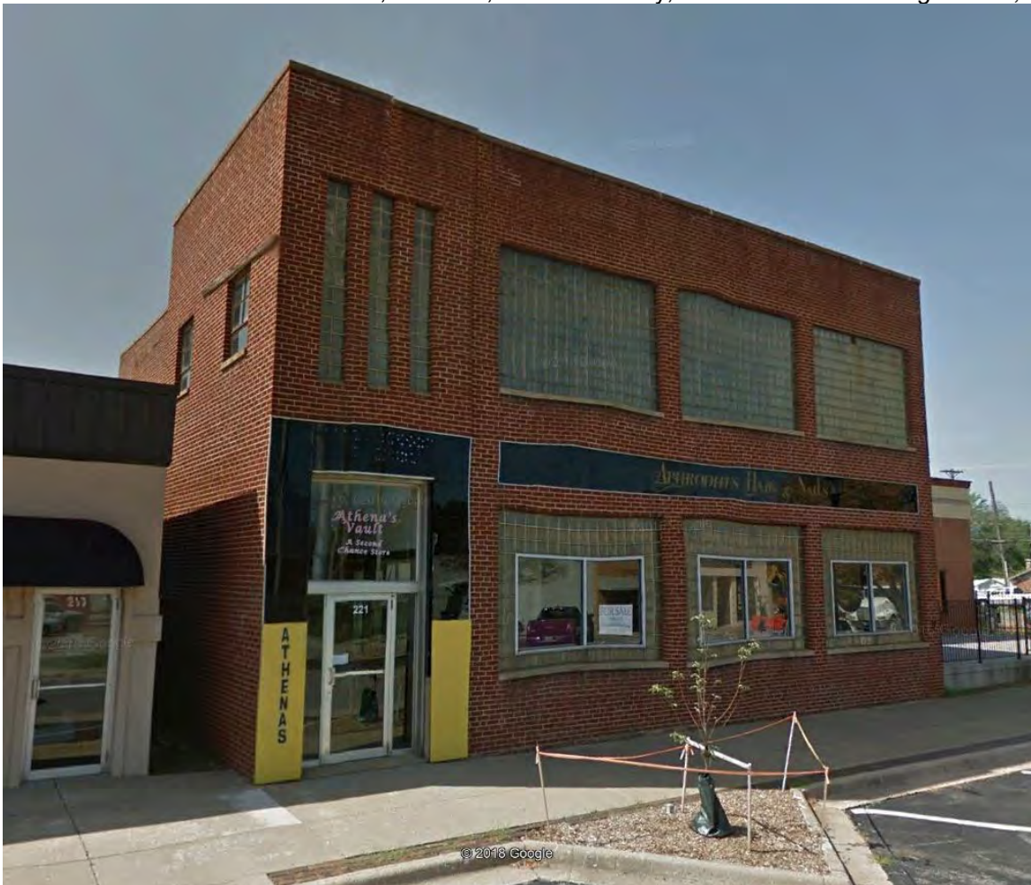
Figure 12. 221 East Commercial Street, Lebanon, Laclede County, Missouri. Source: Google Earth, 2018.
