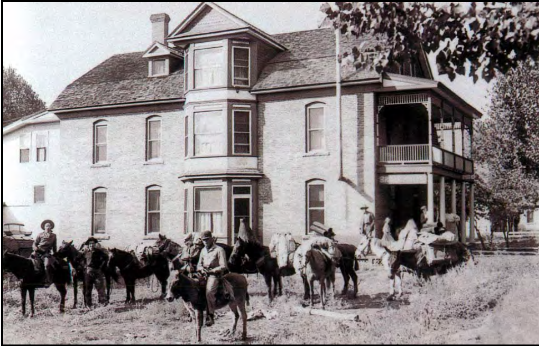
Figure 1 – Bross Hotel looking at south-facing side; Post card reads: “A survey team leaves the Bross Hotel, circa 1913.” (However, the 1912 rear addition has not been constructed) from ColorCards.Com. Inc., 2001 on file at History Colorado
