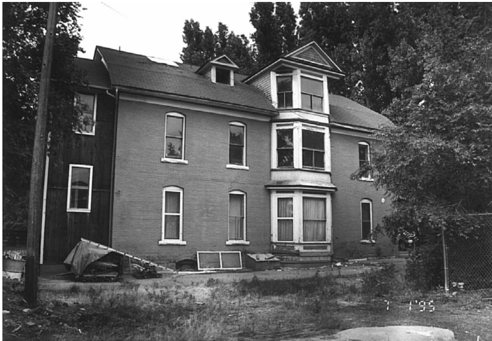
Figure 6 – 1995 Bross Hotel south-facing side; looking north, prior to renovation. On file with the Office of Archaeology and Historic Preservation, Denver, CO.
