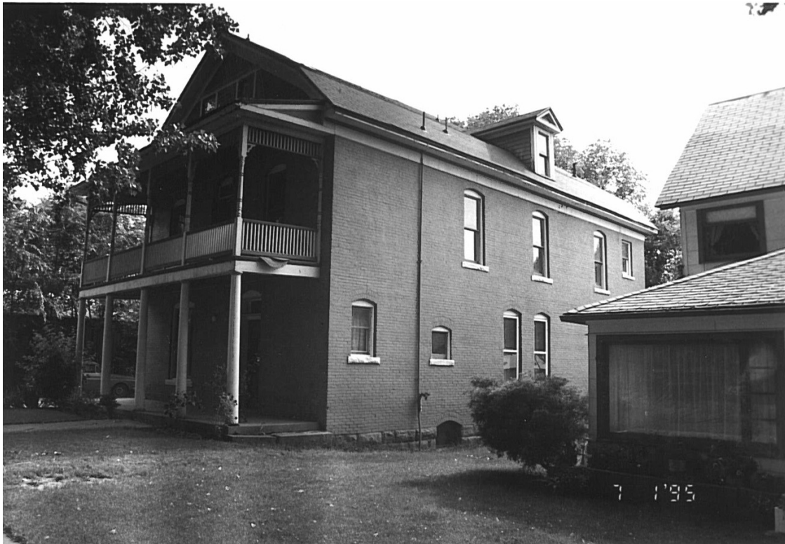
Figure 7 – 1995 Bross Hotel north and east-facing sides; prior to renovation, looking southwest. On file with the Office of Archaeology and Historic Preservation, Denver, CO.
