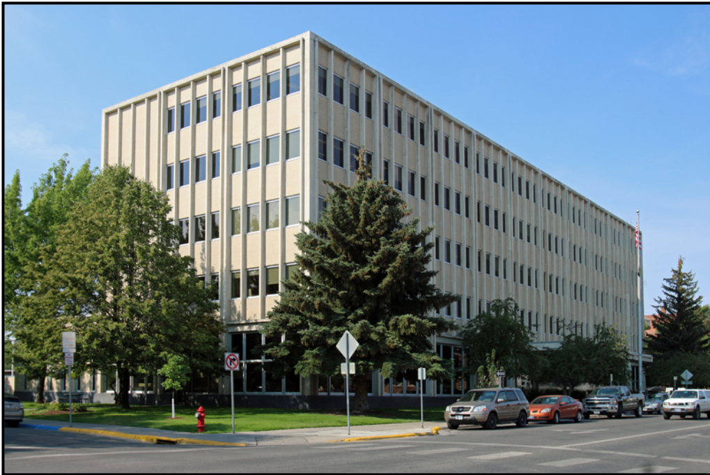
Photograph 1. Overview of the FB&USPO, facing southwest.
