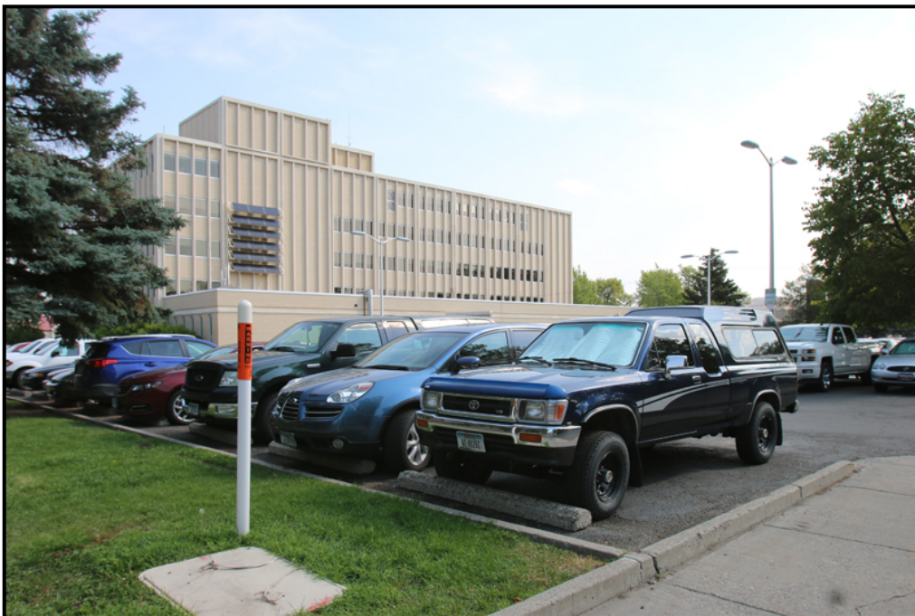
Photograph 2. View from the southwest corner of the property, facing northeast.
