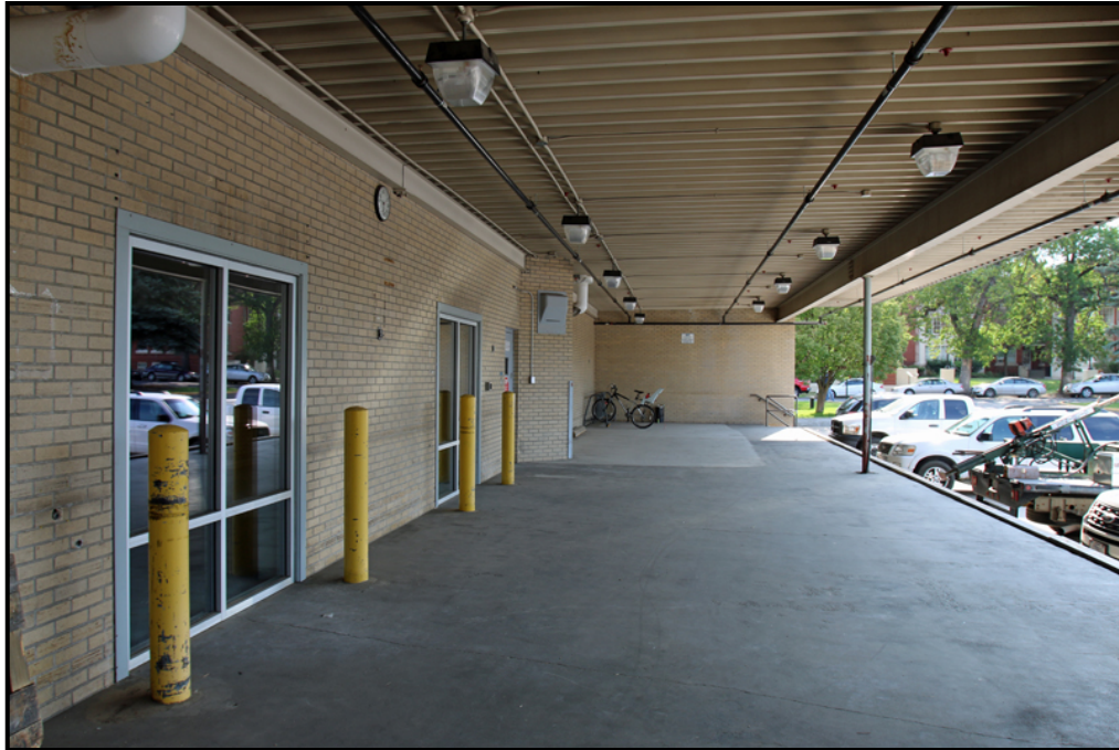
Photograph 7. Overview of the loading platform, facing east.
