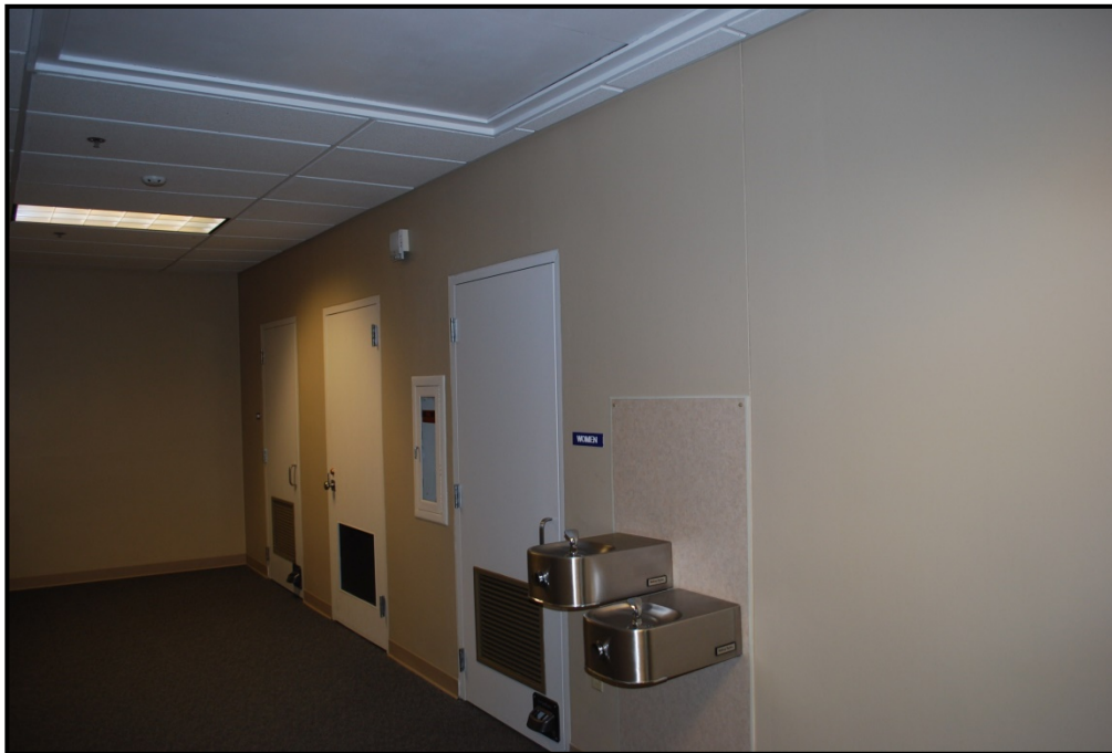
Photograph 20. Widened fifth-floor restroom entries, facing southwest.
