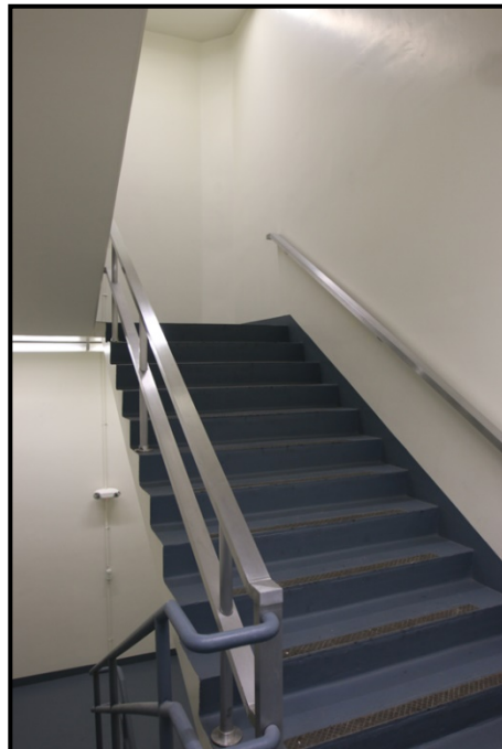
Photograph 18. Stair core at fifth-floor landing, facing southeast.
