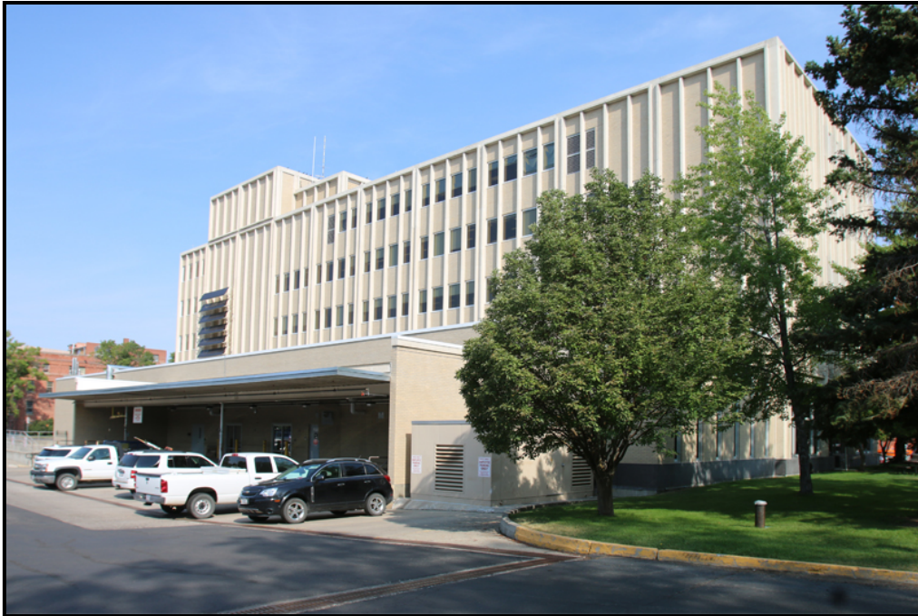
Photograph 3. Overview of the rear (south) elevation, facing northwest.
