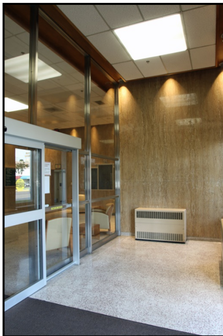
Photograph 8. Overview of the entry vestibule, facing southwest.
