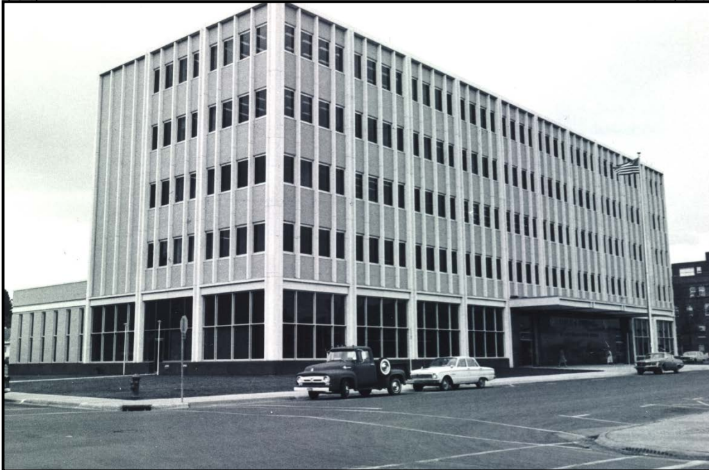
H1. April 1970 view of the façade (north elevation) and east elevation, facing southwest.
