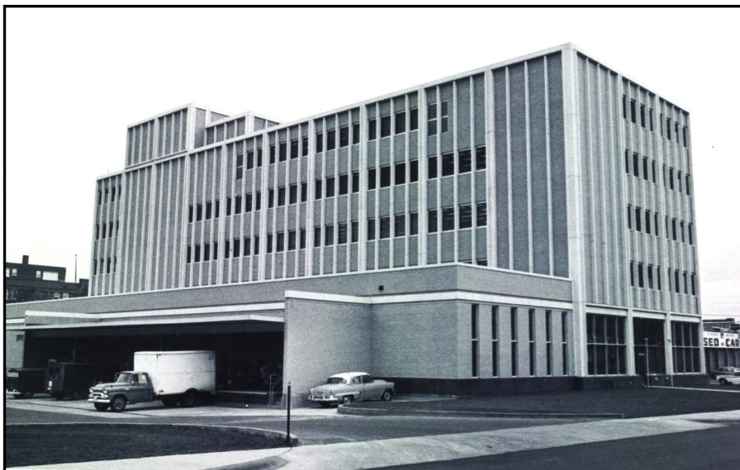
H4. April 1970 view of the rear (south elevation) and east elevation, facing northwest.
