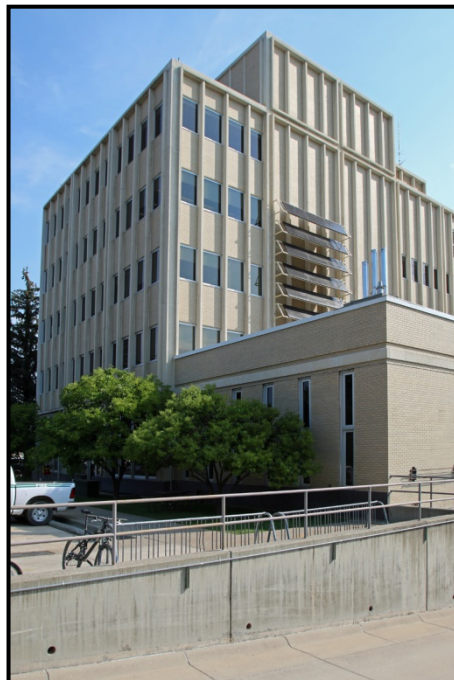
Photograph 4. Overview of the west elevation, facing northeast.
