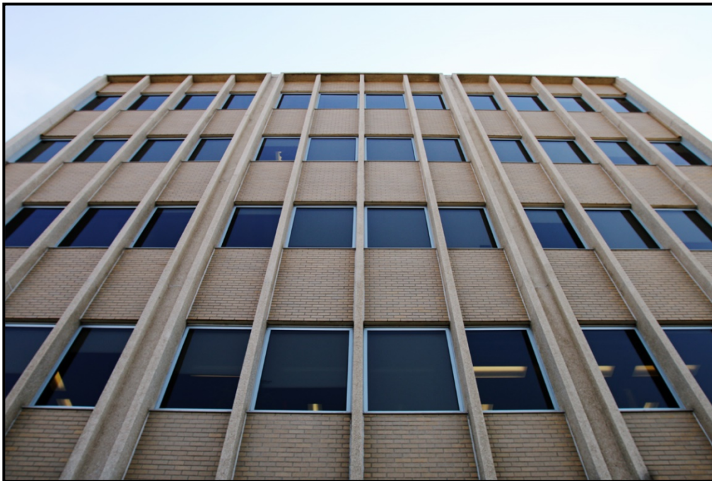
Photograph 6. Overview of the second through fifth floors, facing east.
