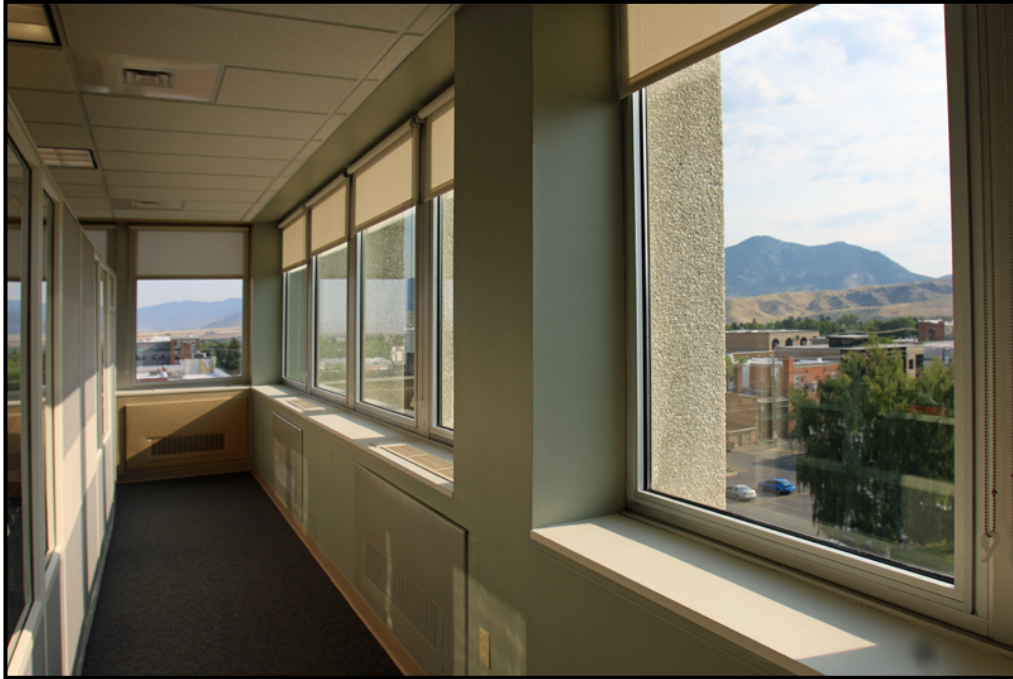
Photograph 17. Office space at the eastern end of the fifth floor, facing north.
