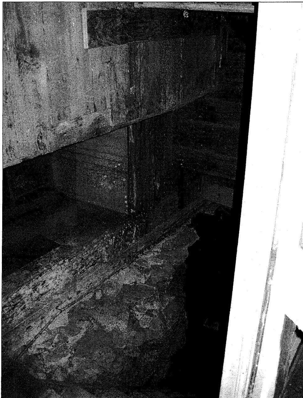
Photo 17 of 22. Stairs leading to cellar.
