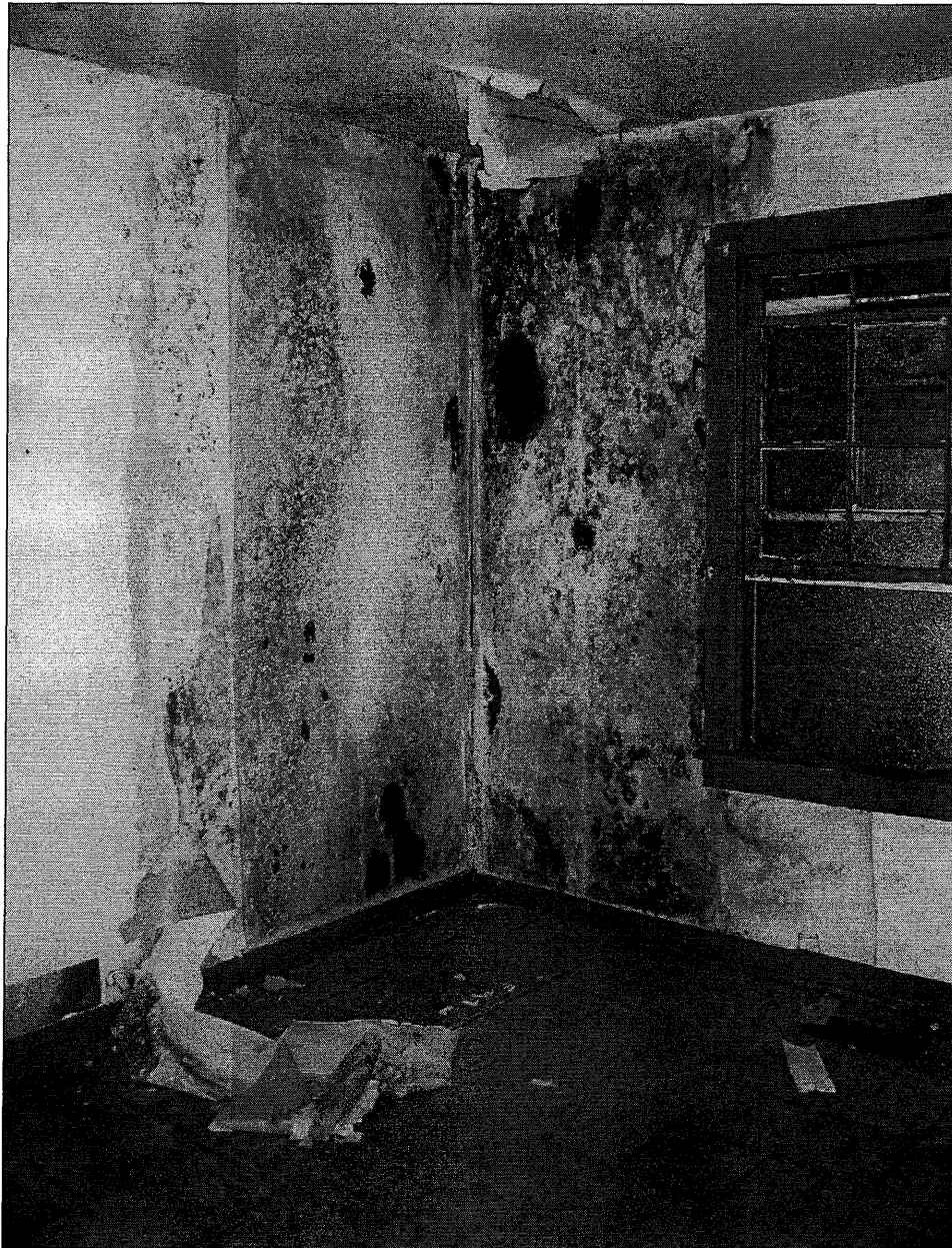
Photo 15 of 22. Main floor bedroom; note original six-over-six window sash. View looking southeast.
