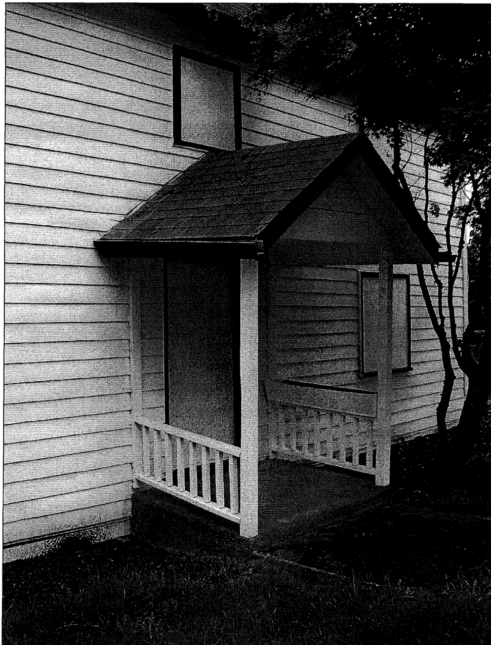
Photo 11 of 22. Front porch detail.
