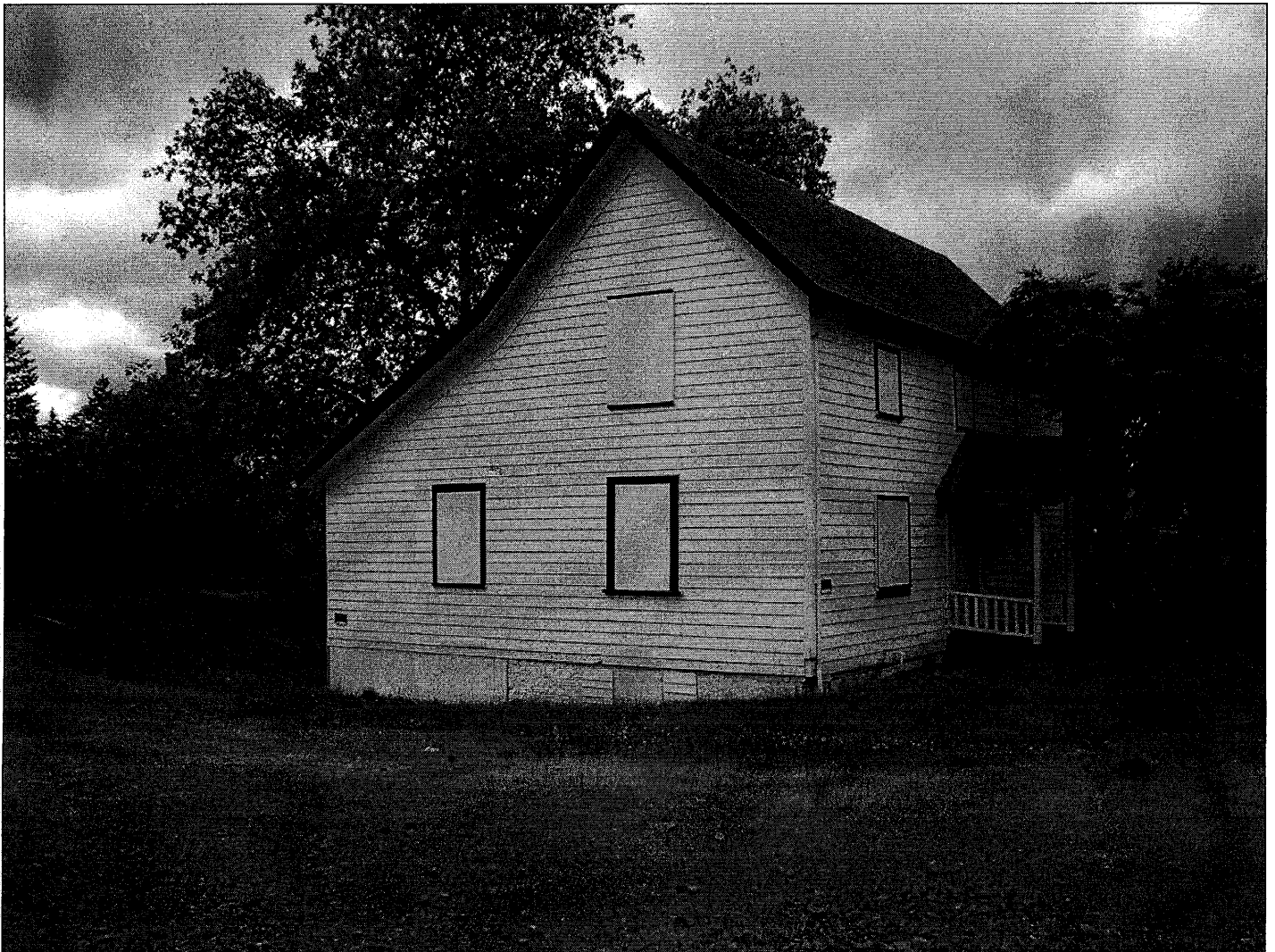
Photo 2 of 22. View of northeast corner, looking southwest.
