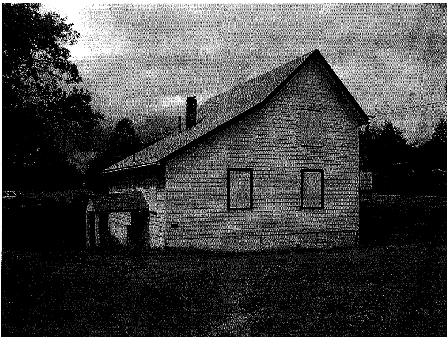
Photo 3 of 22. East elevation, looking west/northwest.
