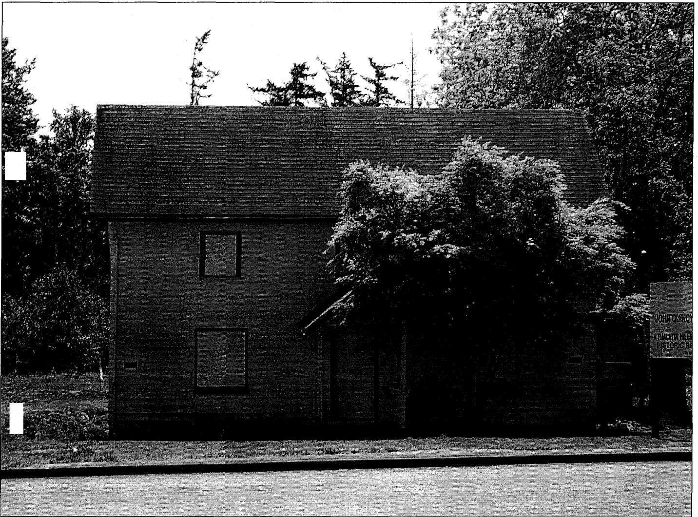
Photo 1 of 22. North (front) elevation from NW Cornell Road.
