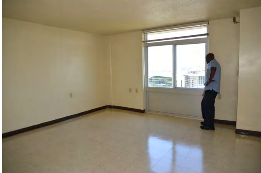
Photo 15. Interior, Ninth Floor, Unit #910, Looking East, Typical
