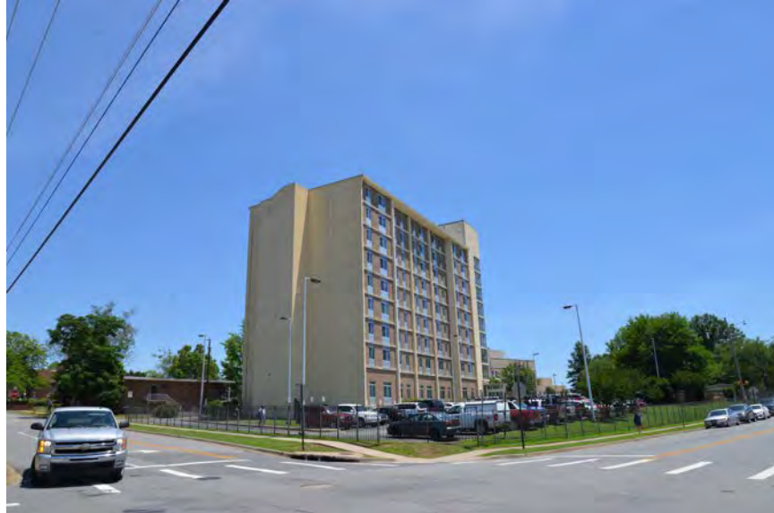
Photo 3. Exterior, West and North Elevations, Looking South
