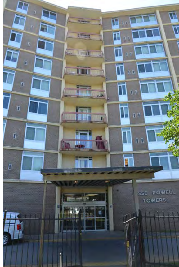
Photo 7. Exterior, East Elevations, Looking West at Entrance
