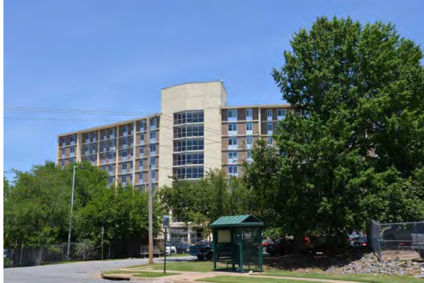
Photo 1. Exterior, West Elevation, Looking East
