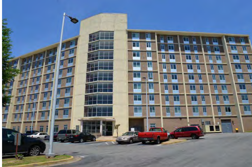
Photo 5. West Elevation, Looking East
