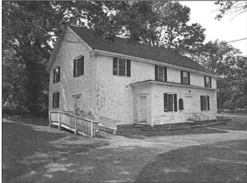
Photo.1. View of exterior from SE.
