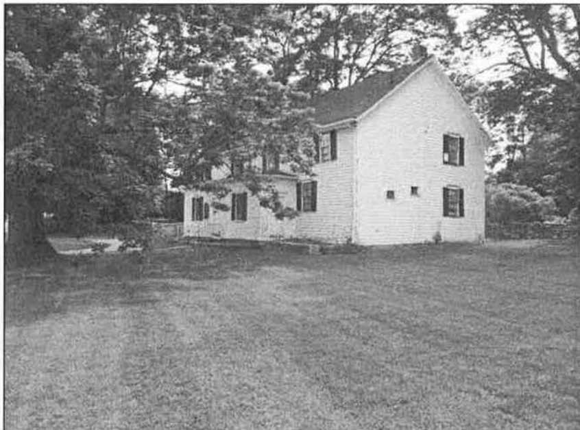
Photo.2. View of exterior from NE.
