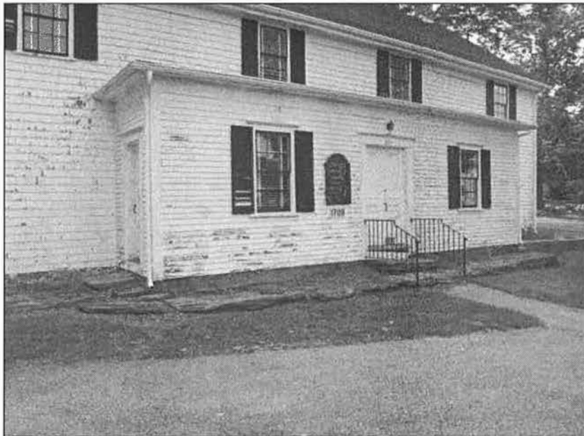
Photo.4. Detail of entrance vestibule on front façade.
