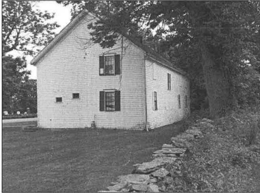
Photo.3. View of exterior from NW.
