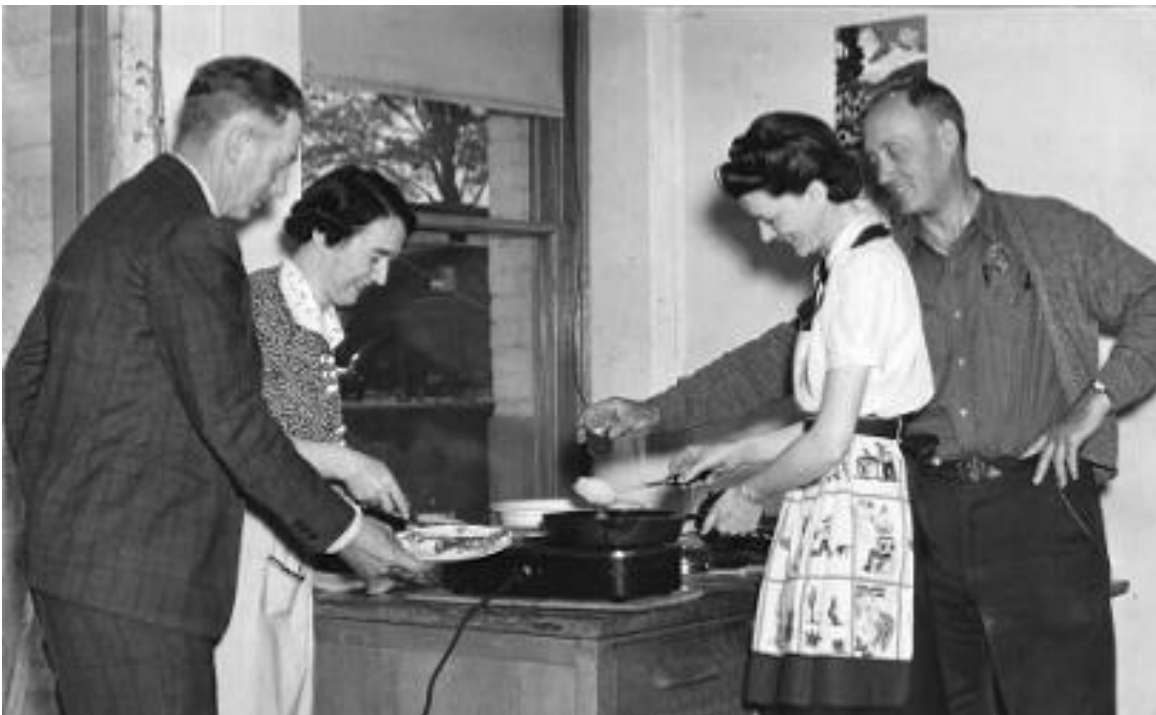
Farewell Breakfast for old County courthouse before demolition, May 16, 1941
