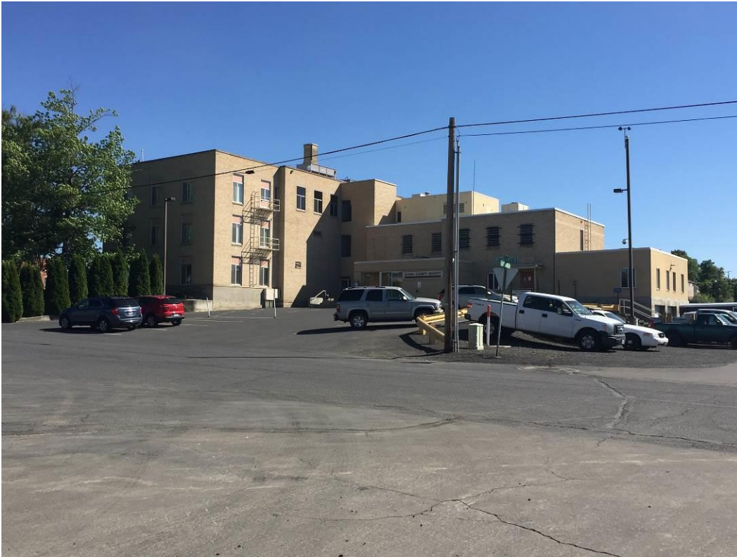
6 of 16 – Northwest corner of building showing north side of building and rear jail wing.
