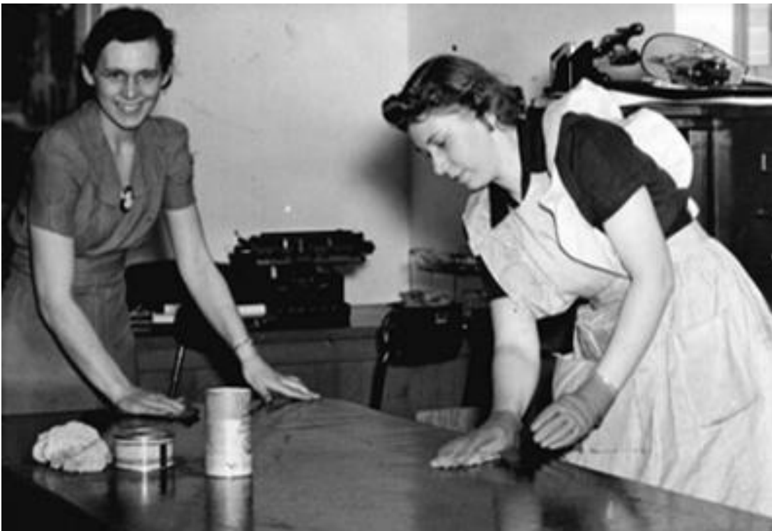
Move in Day to new courthouse building, 1941.
