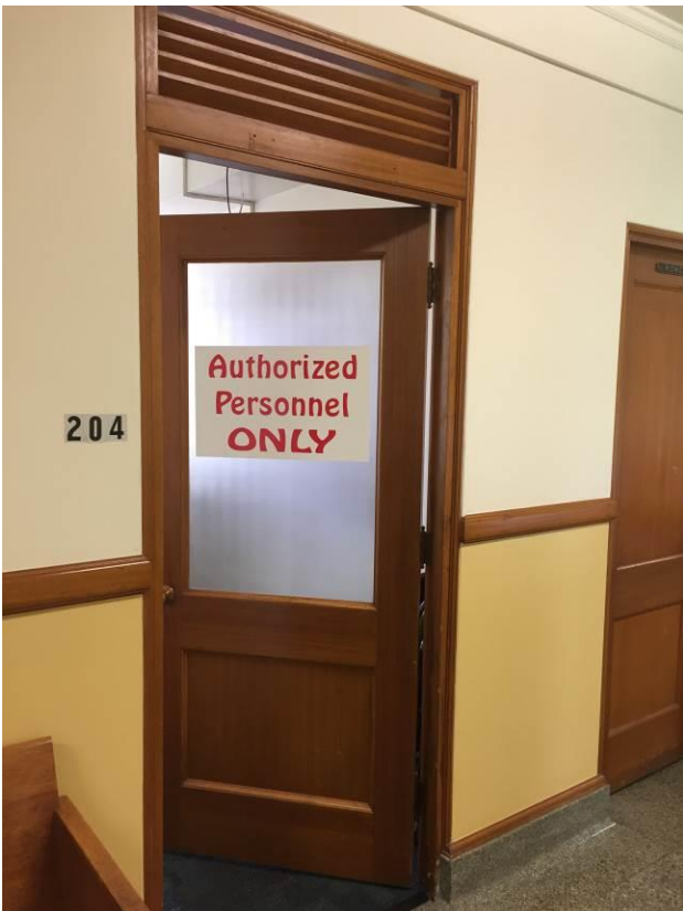
11 of 16 – Typical second floor hallway office door.
