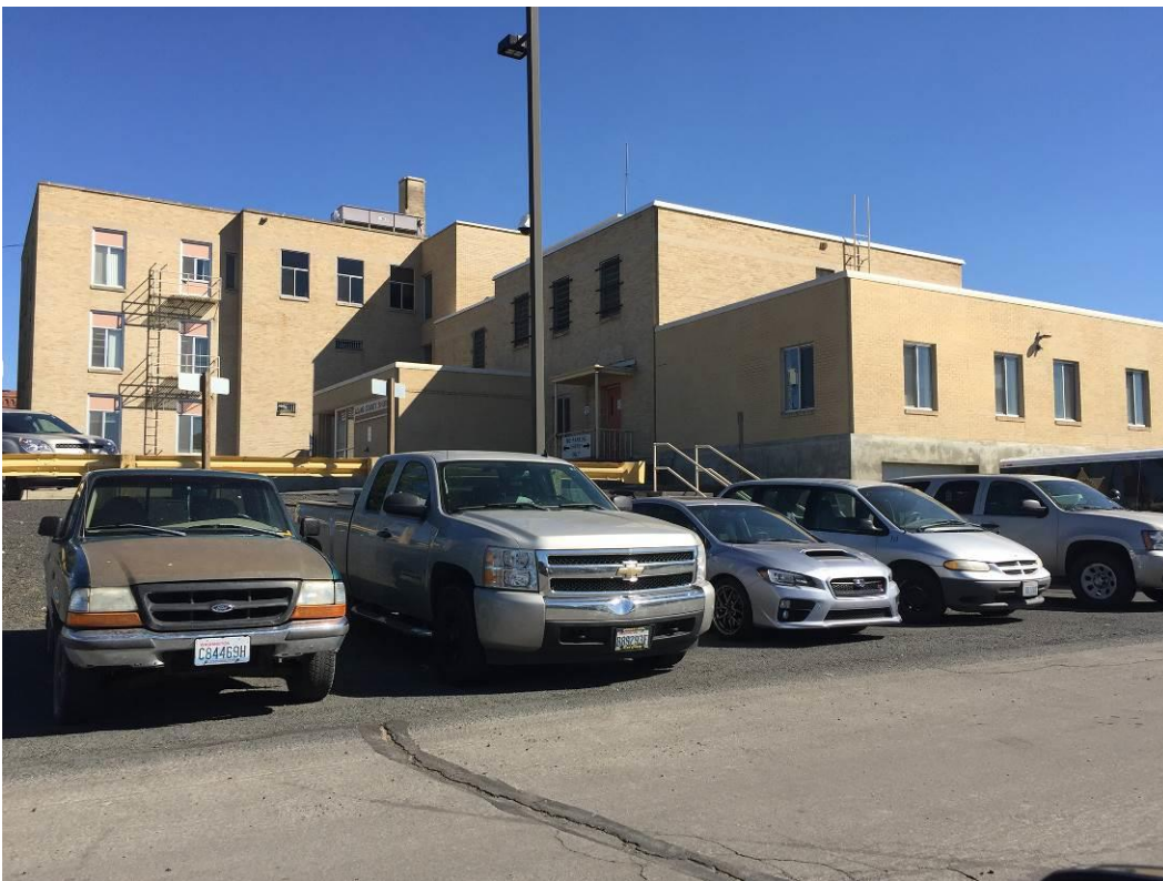
7 of 16 – West façade of building showing rear jail wing.
