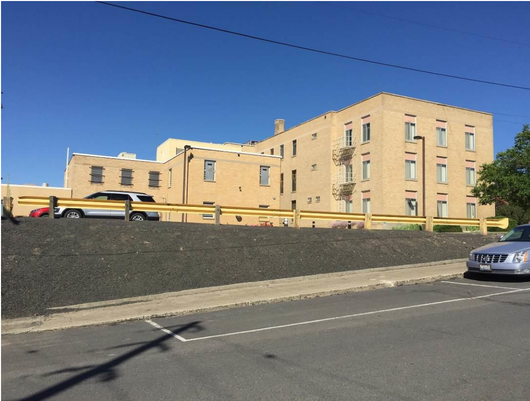
8 of 16 – South façade of building showing rear jail wing.
