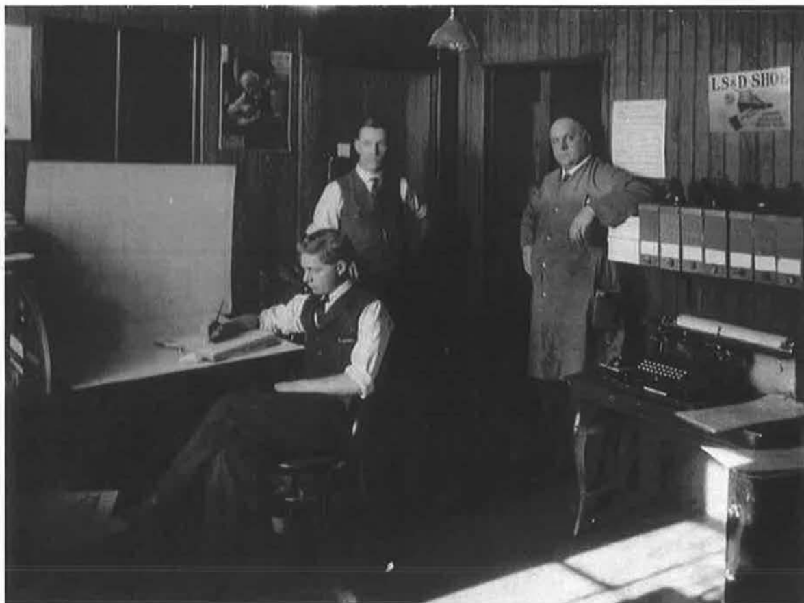
The managers of Leonard, Shaw & Dean pose momentarily for the photographer in the Peirce Street plant offices. The office appears small and is clearly meant to fulfill its basic function. Notice the Leonard, Shaw & Dean advertisement on the wall featuring canvas-top leather shoes beneath which are a number of samples of the high quality men's shoes for which the firm was noted.
