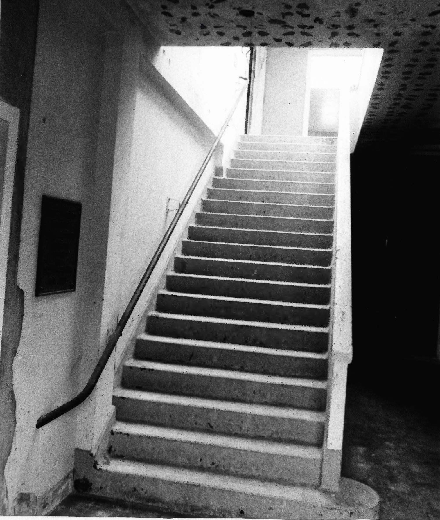
Stairs to second floor (natural light).
