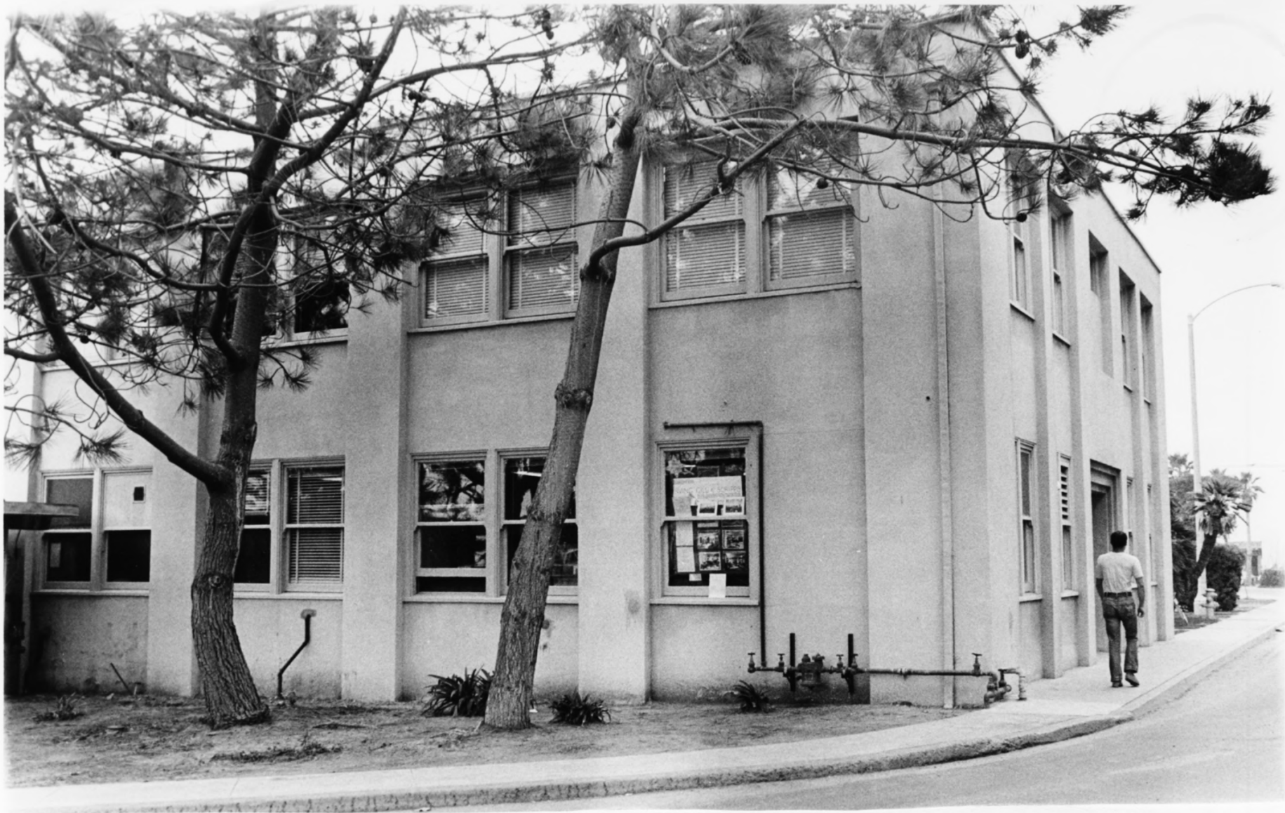
Old Scripps, south (left) and east (right) facades, 1977.
