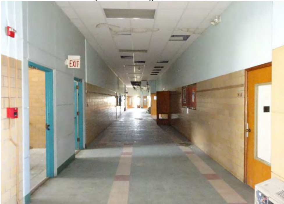
26 of 29 Third floor hallway. Camera facing west.
