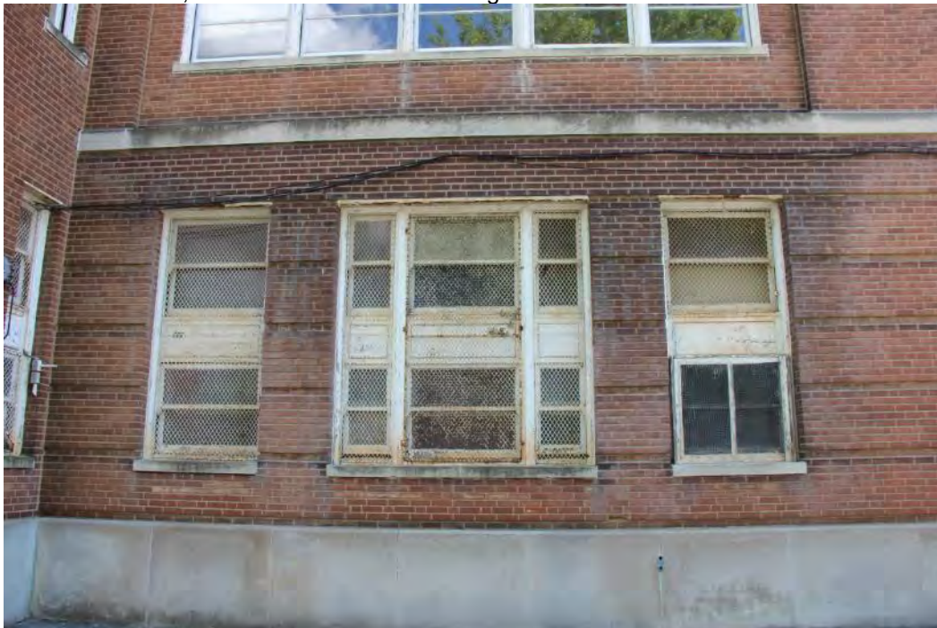
11 of 29. Detail, lower facade. Camera facing south.
