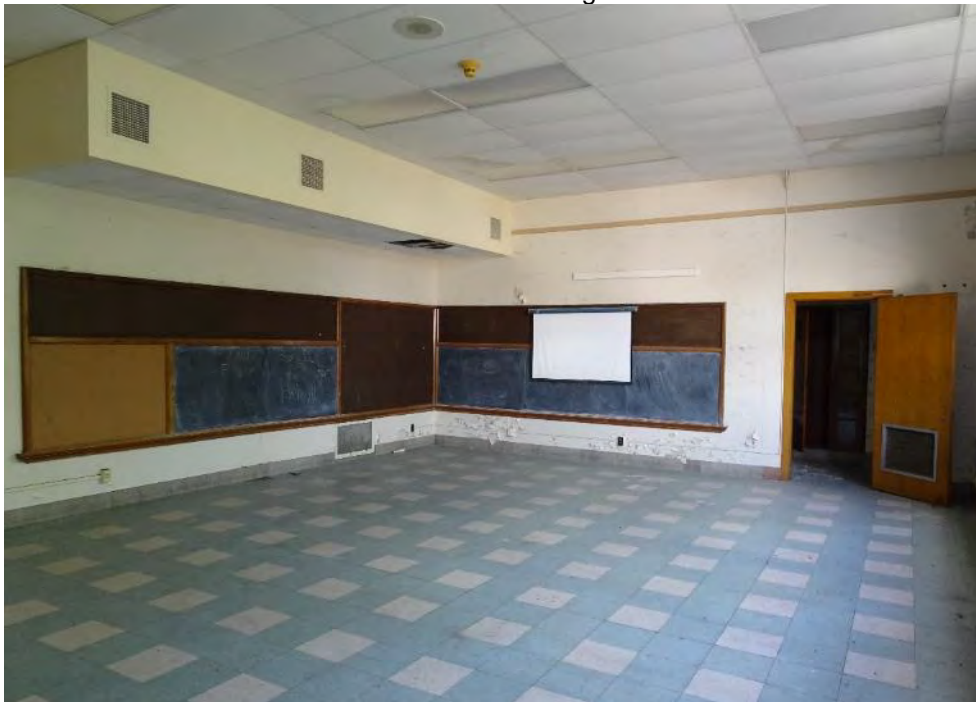
25 of 29 Second floor classroom. Camera facing southwest.
