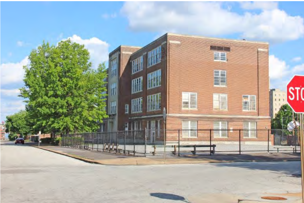
4 of 29. Northwest corner and west play yard. Camera facing southeast.
