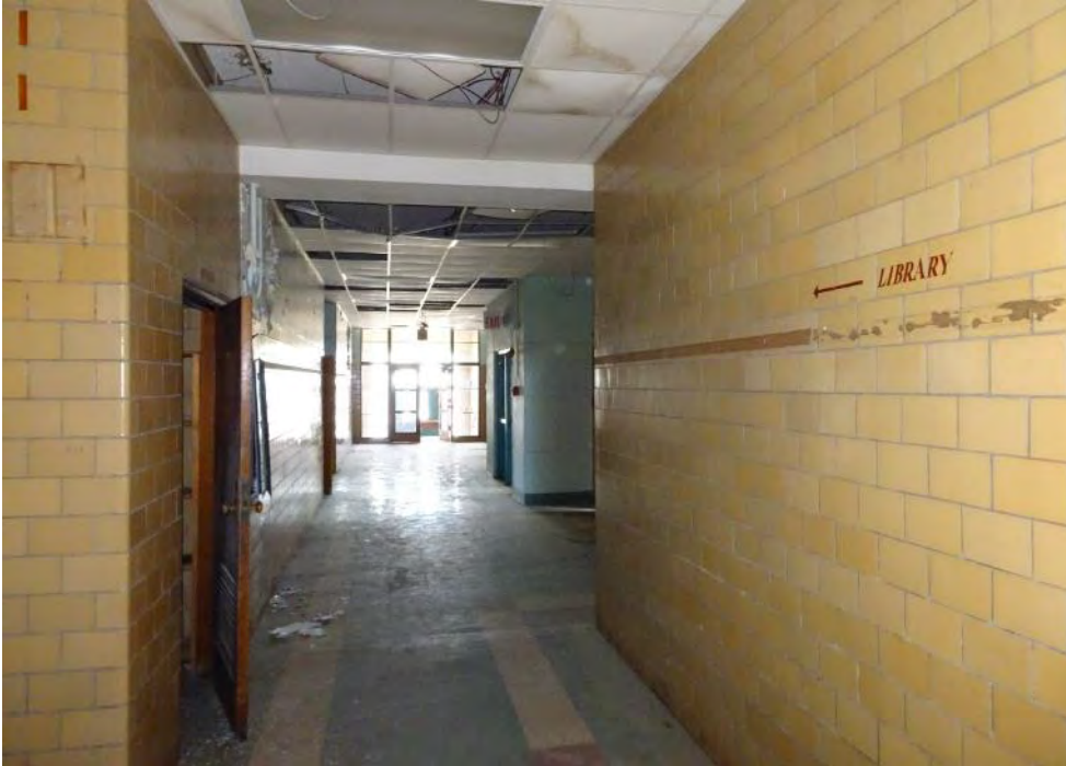
17 of 29 First floor hallway. Camera facing east.
