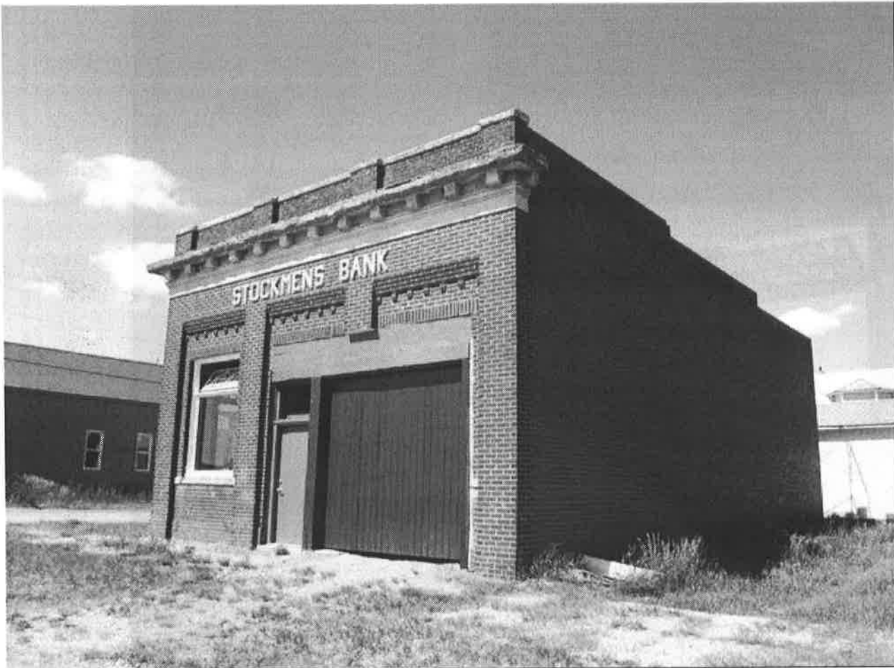
0004 Stockmen's Bank of Martinsdale, East Façade & North Elevation, Facing: SW
