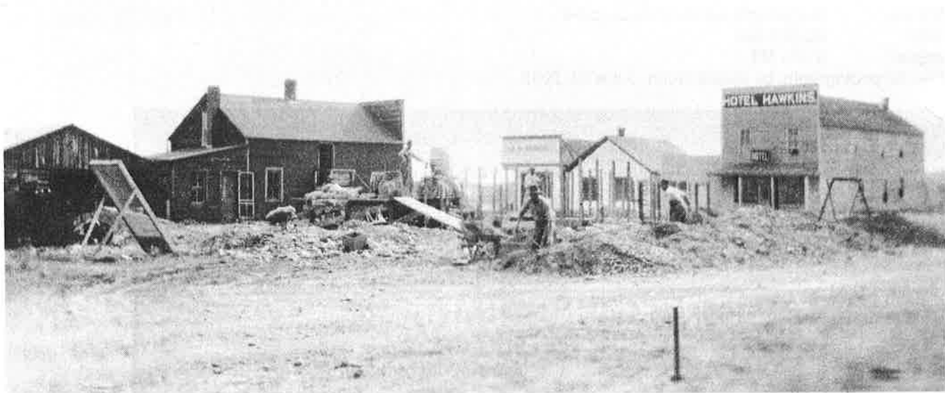
"Martinsdale, Montana, Excavating for New Bank, 1919. Photographer Unknown" PAC 2012-34.2, MHS Research Center.
