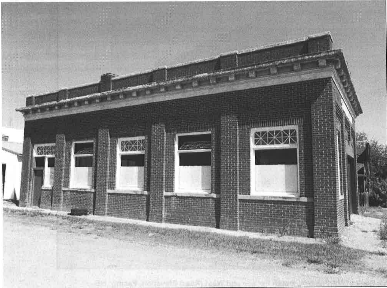
0002 Stockmen's Bank of Martinsdale, South (Grant Street) Façade, Facing: NW
