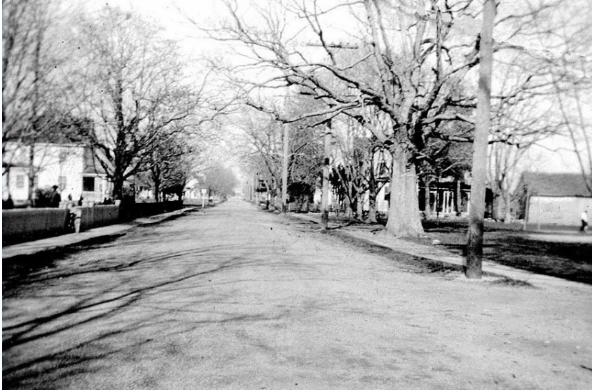
Figure 20: View east down Petersburg Road, ca. 1915. The house at the left is the Osman and Clara Geary House (extant) built in 1913 at 672 Petersburg Road.
