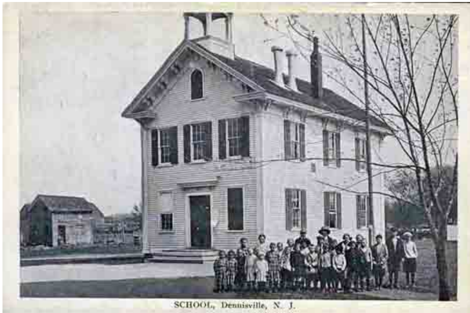
Figure 14: Dennisville Public School, ca. 1910. This is what the 1874 building looked like until the second story and attic burned in 1948. The school was then rebuilt to its present one-story height.
