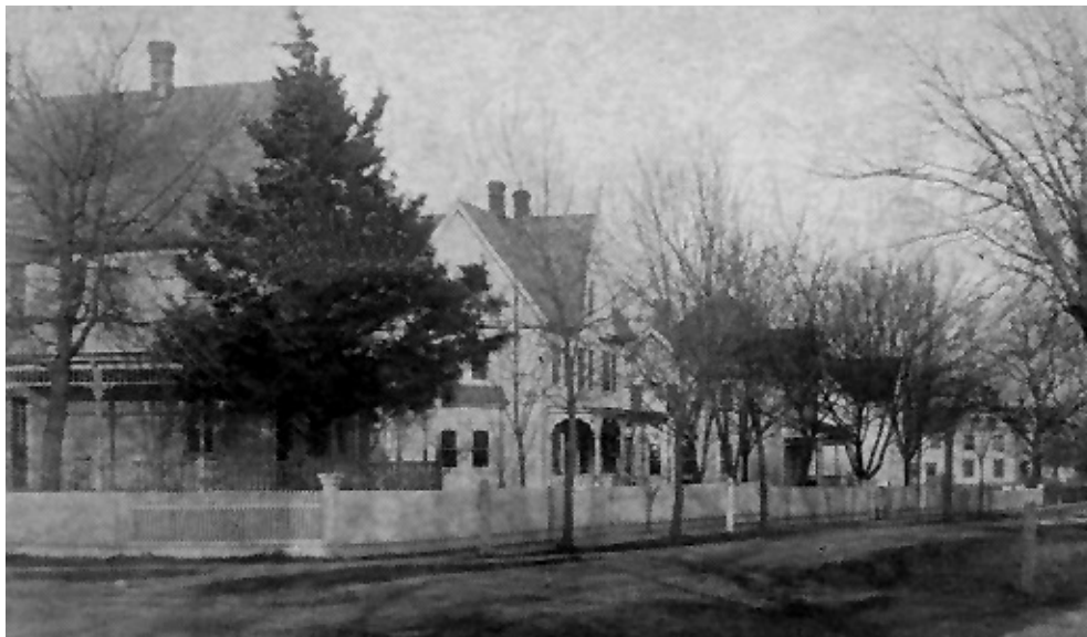
Figure 23: View northeast down Petersburg Road, from the Fidler Road intersection. Ca. 1920. Compare this with photo 11.
